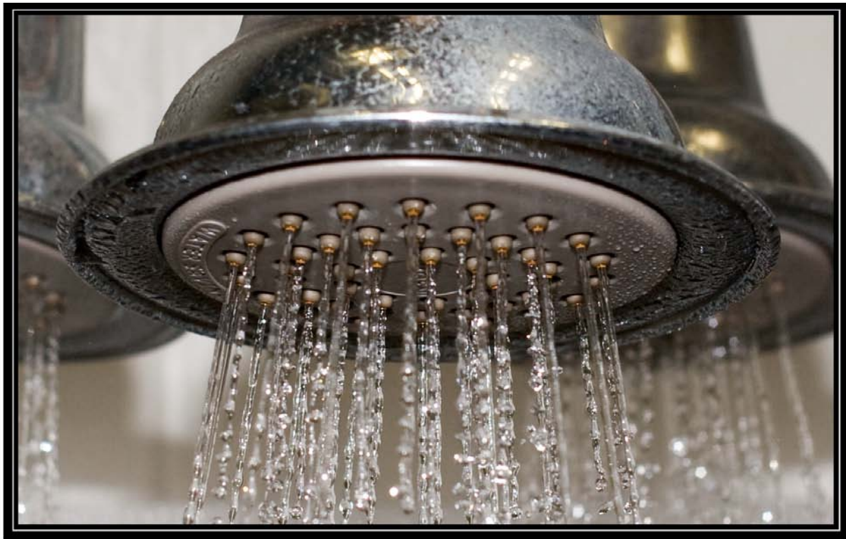
Figure 6-1D. Showerhead 1 on seventh day of testing with soft well water (<1 grain per gallon) showing spray pattern. Battelle testing for Water Quality Association. May 1, 2009
