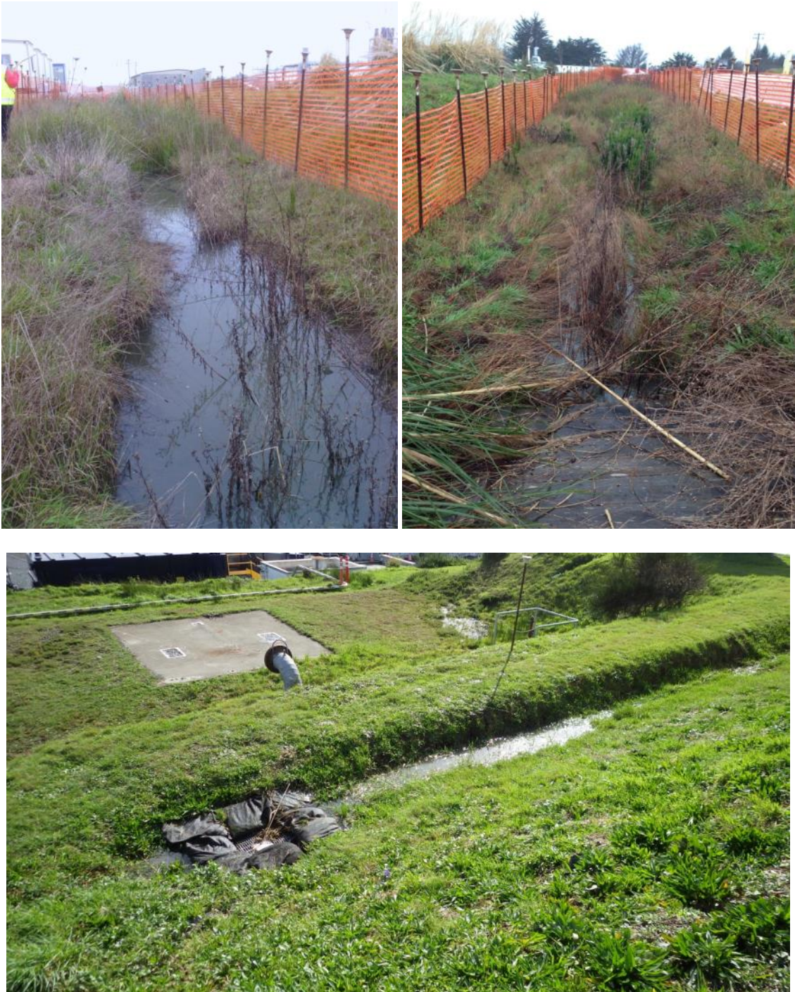
Figure D-3. Intermittently flowing drainage ditch (DD-1). Bottom image shows connectivity to adjacent drainage ditch and drainage inlet to stormwater system, see Figure 5.
