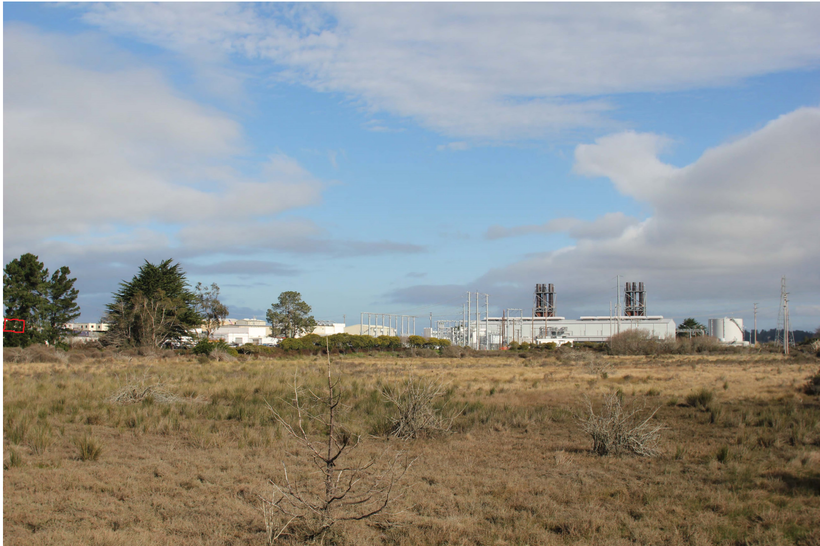
View from King Salmon Avenue with the location of the Waste Management Building outlined in red.
