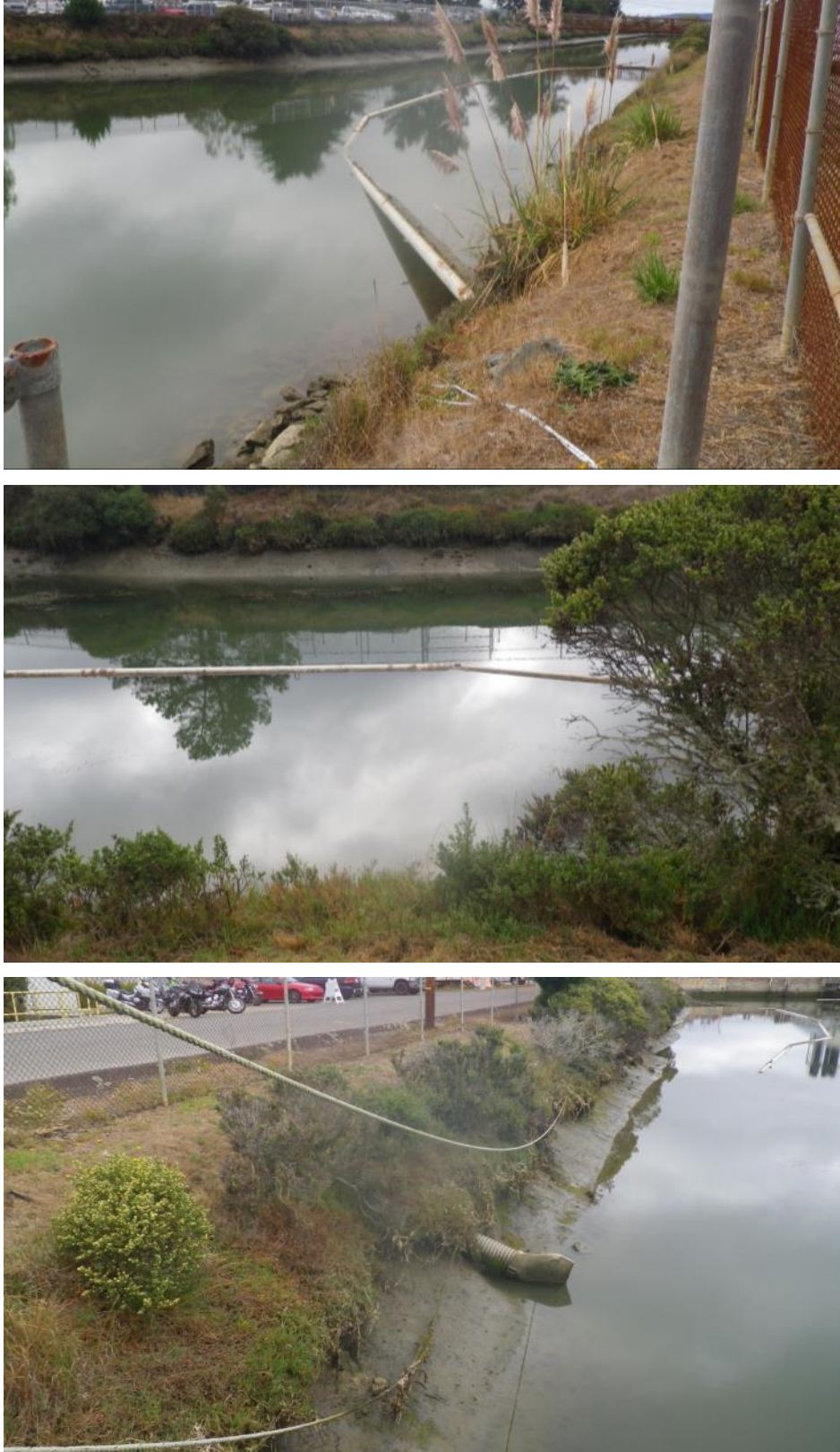
Figure D-2. Intake Canal (W-2).
