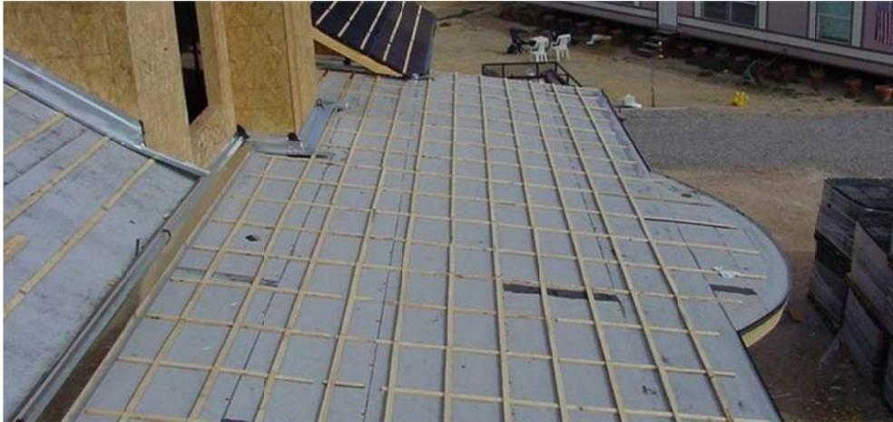
**Figure 9: Ventilation for Tile Roofing – Counter Batten (CBIA Forum)**
