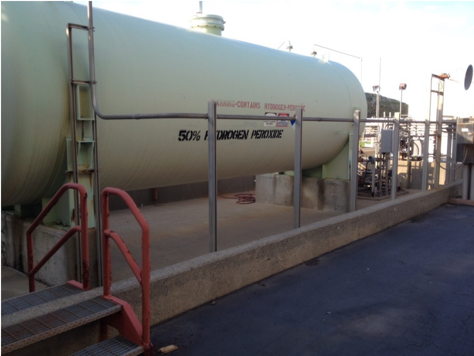
Attachment B Photos of Existing Hydrogen Peroxide Storage Tank and Containment Plant 2
