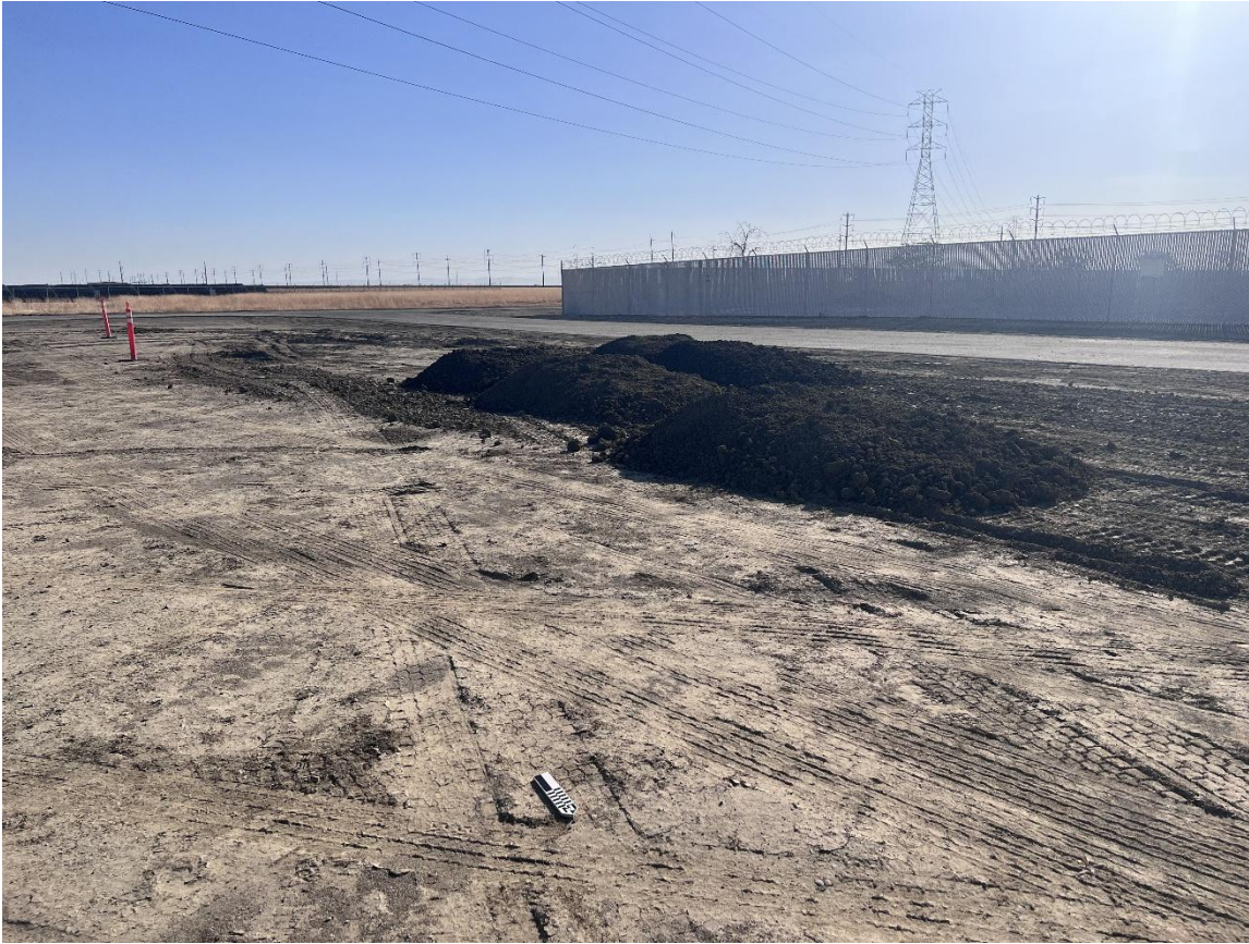
16:32 Facing south Spoils being spread south of auger location.
