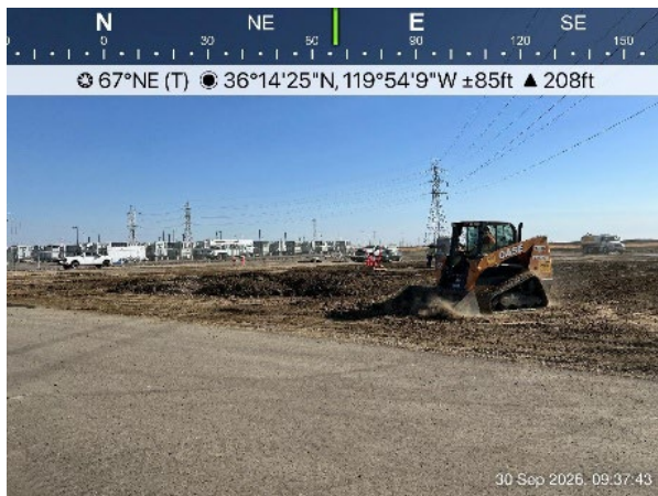
Crew began spreading the spoils in the parking area using a bulldozer and water truck.
