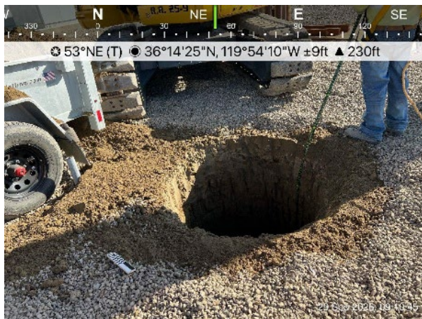
Completing the 2nd bore hole with a scale and north arrow.
