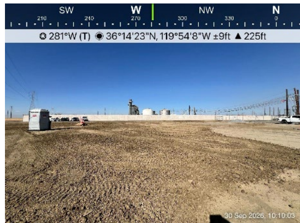
End of day. Spreading of the spoils is complete.
