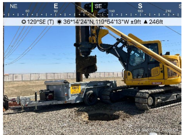
Drilling the 3rd bore hole using the auger. The previous two poles are to the top left of the photo, behind the fence and out of frame.
