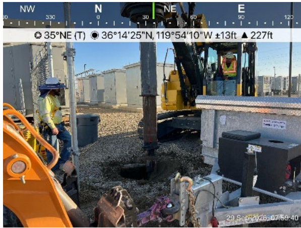
Crew digging the 5 ft hole. The auger is seen in this photo.
