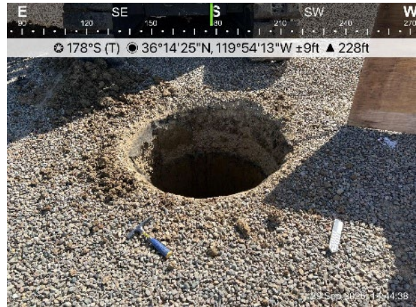
The completion of the 3rd bore hole. Rock hammer and north arrow for scale.
