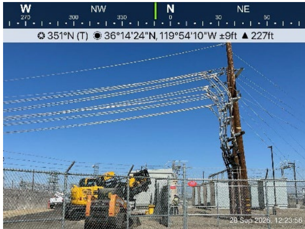
Overview of the project area. Pictured is the augur and power poles that need to be moved forward. The little dozer was used to carry off excavated material.
