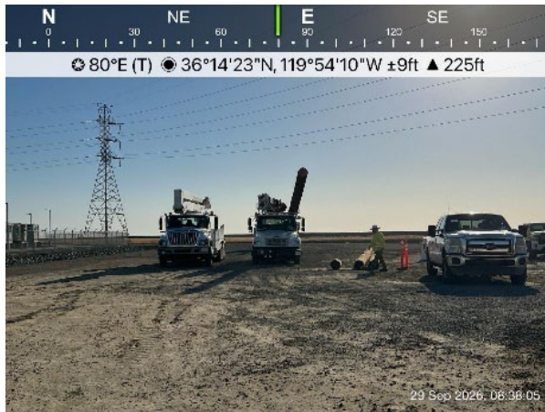
The crew prepared the poles to be inserted into the bore holes dug this morning and yesterday.
