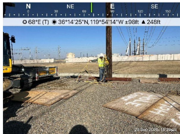
End of day. The final two bore holes are completed and covered with wood.
