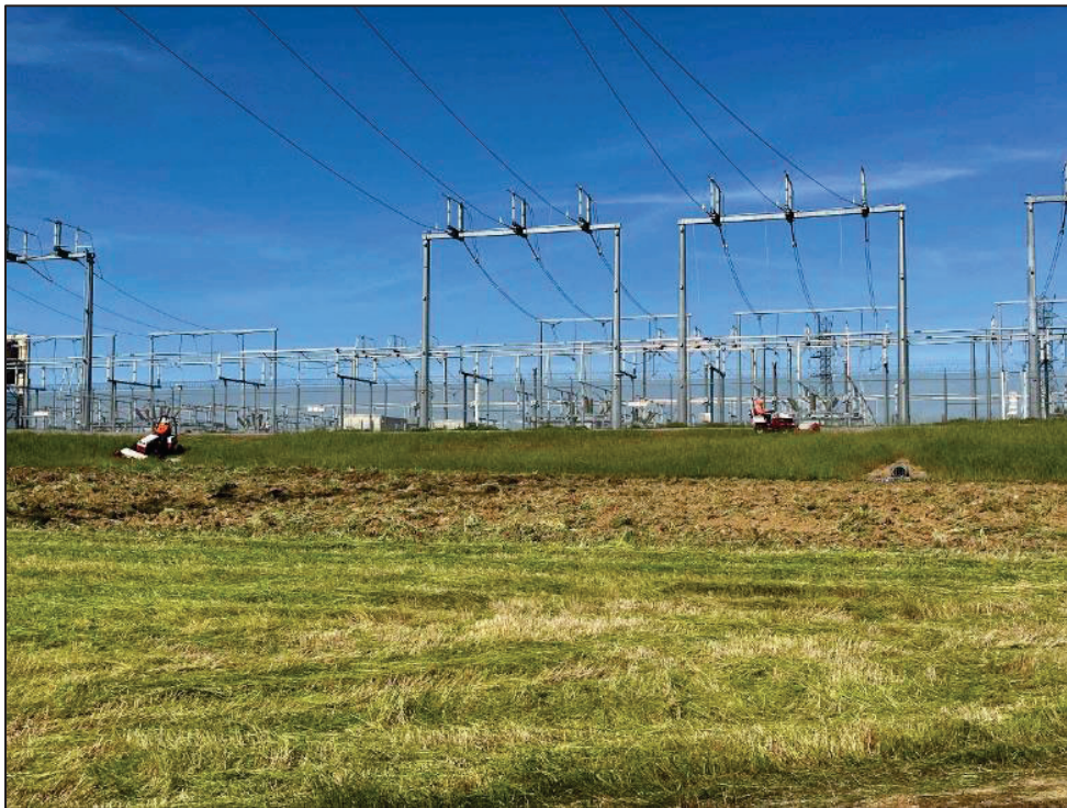
Photo 6: The Sierra Integrated Services vegetation management crew mowing the grass embankment east of the Delevan Substation on April 29, 2025.
