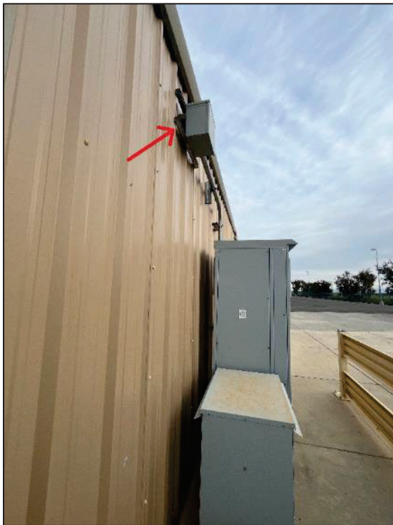
Photo 2: A house finch nest was found east of the warehouse behind a metal box on April 7, 2025. The Biological Monitor could not determine if the nest was being incubated or if it contained eggs.
