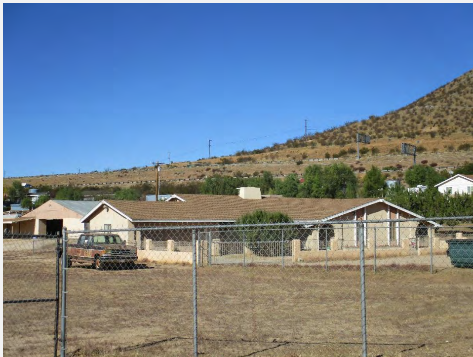
Photograph 2. East and south elevations, view looking northwest.
