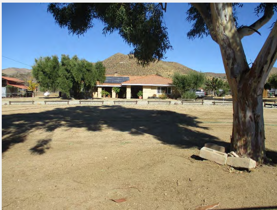
Photograph 2. Primary (south) elevation, view looking north.
