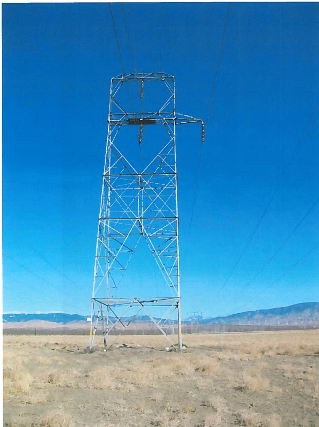
Tower Type #3: Transposition Vincent Tower (Mile 49-T1).
