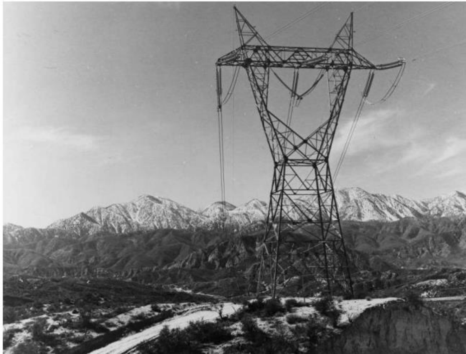
Exhibit 2. Typical SCE 500kV transmission tower, circa 1973
