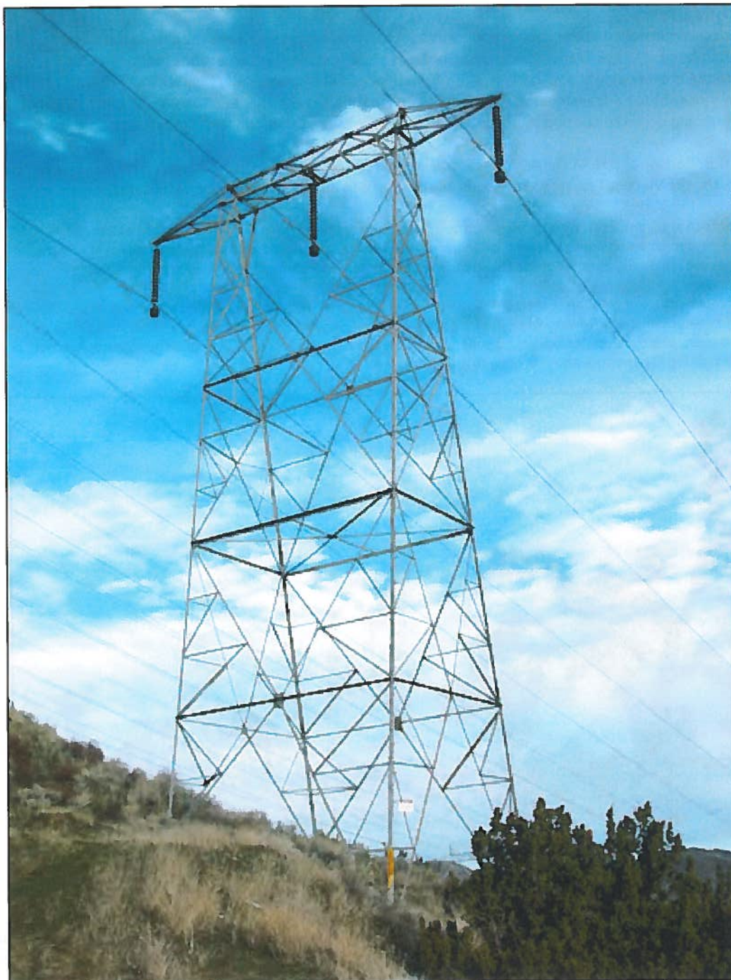
Tower Type #1: Suspension (Standard) Vincent Tower (M18-T1).
