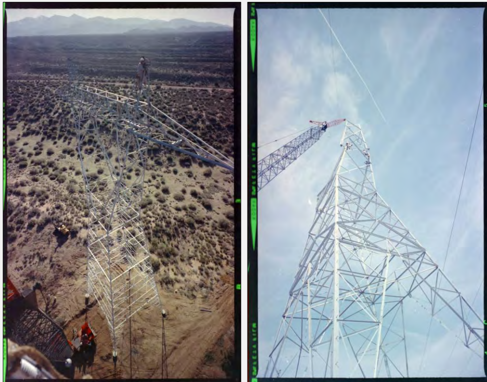
Exhibit 2. Lugo-Vincent 500kV towers under construction, 1968.
