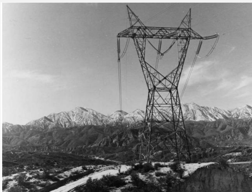
Exhibit 4. Typical SCE 500kV transmission tower, circa 1973.
