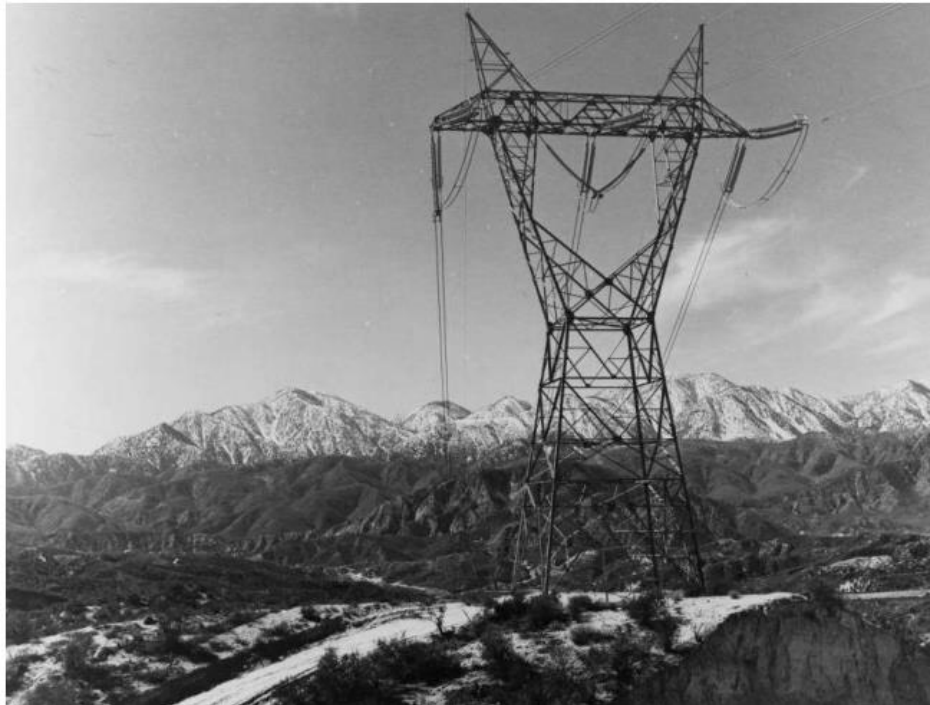
Exhibit 1. Typical SCE 500kV transmission tower, circa 1973
