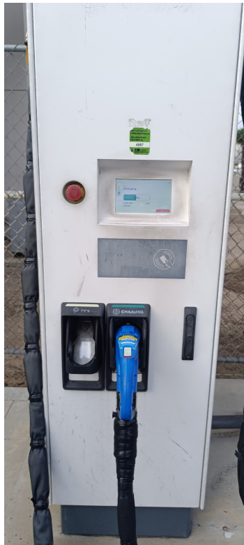
Exhibit K - Station 4987. Wider view; CCS position appears unavailable/empty while CHAdeMO hardware remains.
