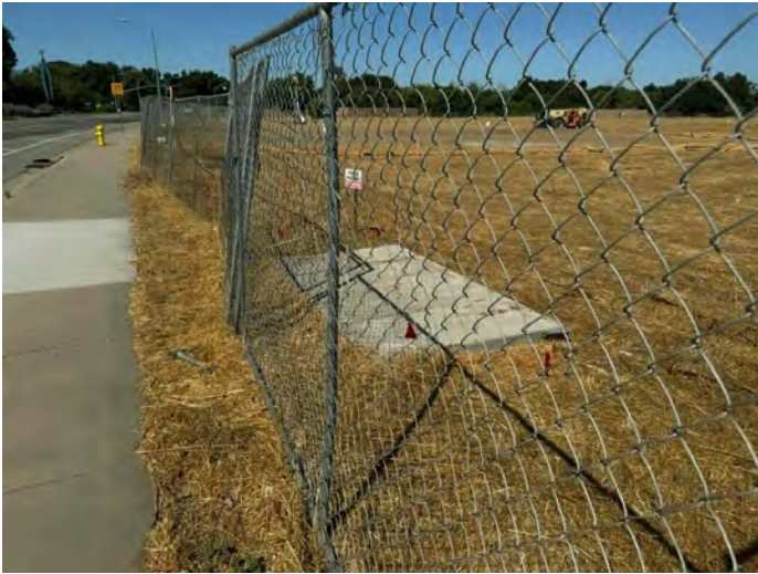
13. View of utility infrastructure at the subject property
