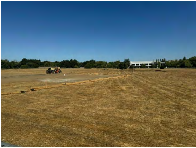
16. View of an area of grading and equipment at the subject property
