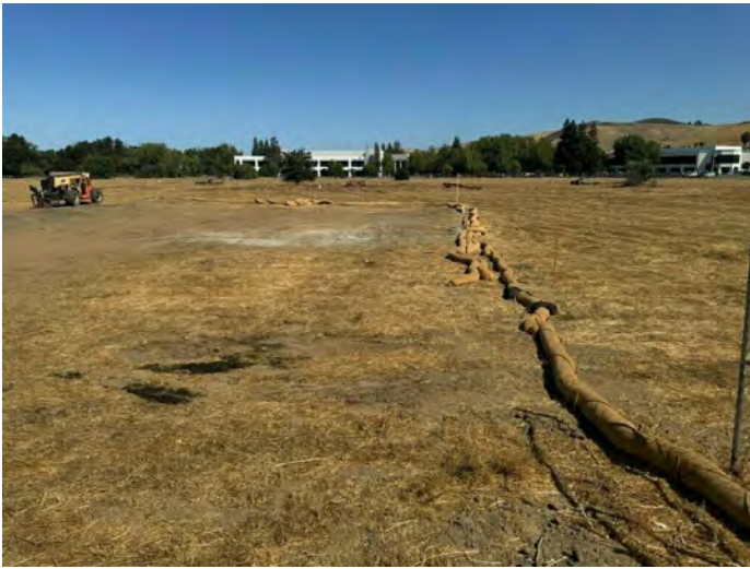
15. View of an area of grading and equipment at the subject property
