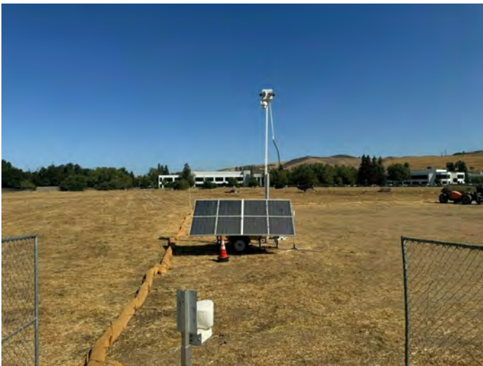
18. View of an area of grading and equipment at the subject property
