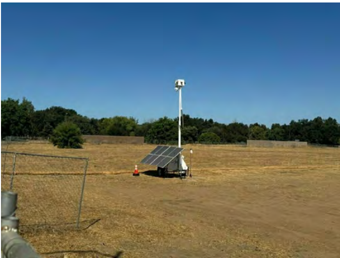
17. View of an area of grading and equipment at the subject property
