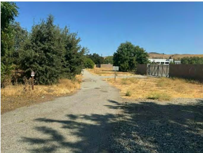
35. View of adjoining utility potable groundwater production well infrastructure to the west
