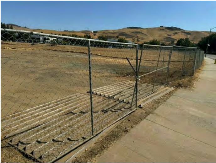
14. View of a gated entrance to the subject property
