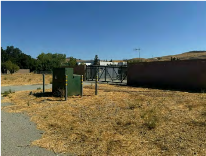
37. View of adjoining utility potable groundwater production well infrastructure to the west
