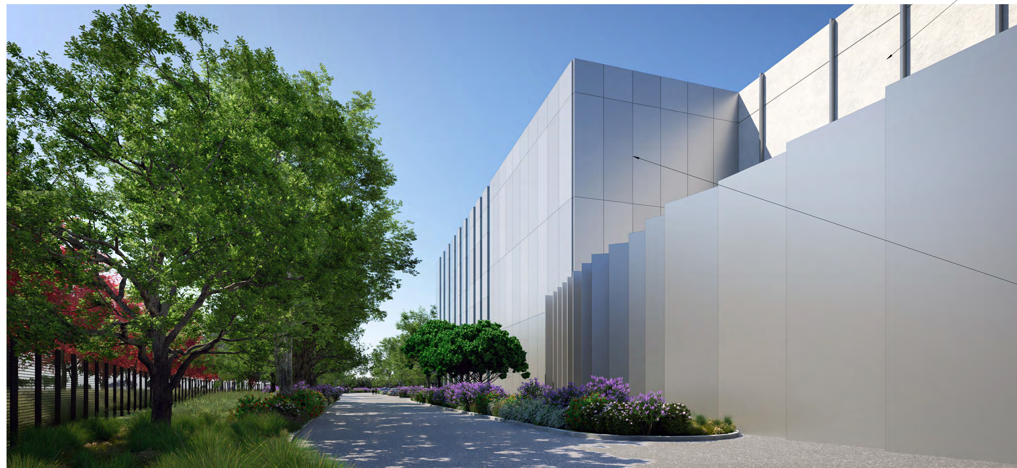
SOUTHEAST CORNER VIEW
