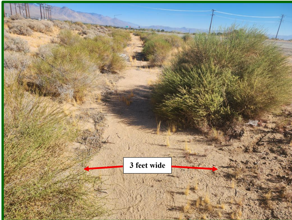
Exhibit 8b. Drainage 1 at right-of-way crossing, facing north.
