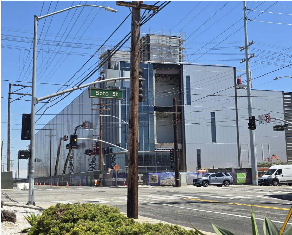
Figure 3. Image from August 2026, depicting the Goodman logo at the Goodman LAX01 Vernon Data Center site under construction. 21
