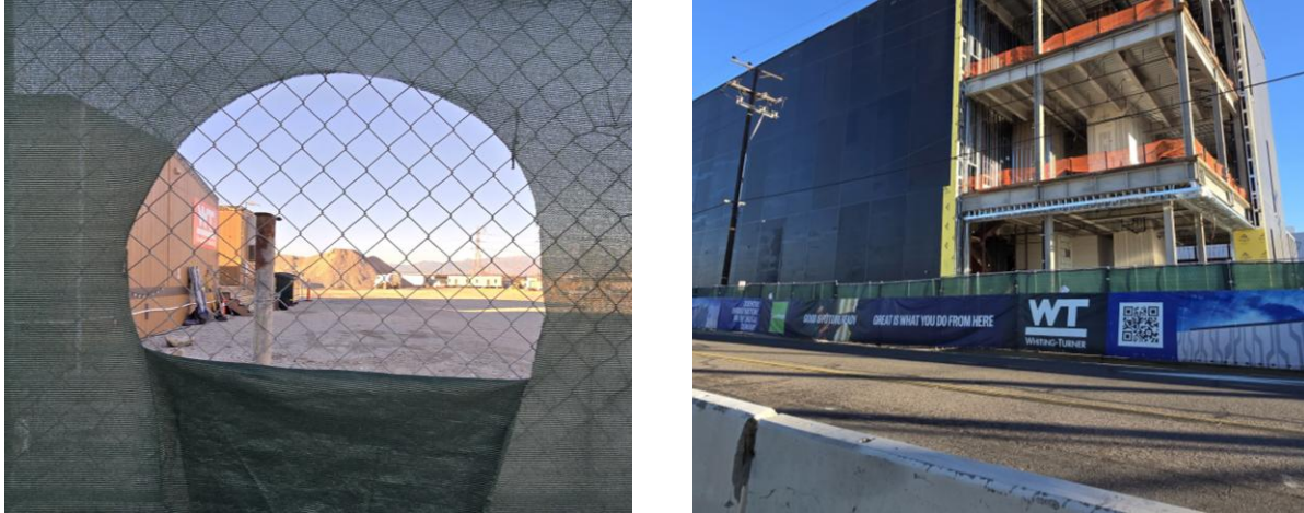
Figure 4. Images from February 2026, depicting Whiting Turner logos at (1) the fenced-in Goodman Energy Park Data Center site [left]; and (2) the Goodman LAX01 Vernon Data Center site [right] under construction. 26
