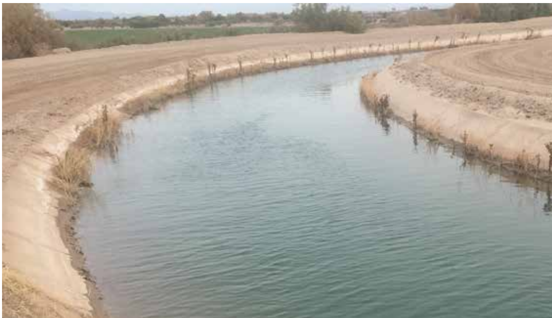
Figure 7. Example of Existing PVID Slip-lined Canal
