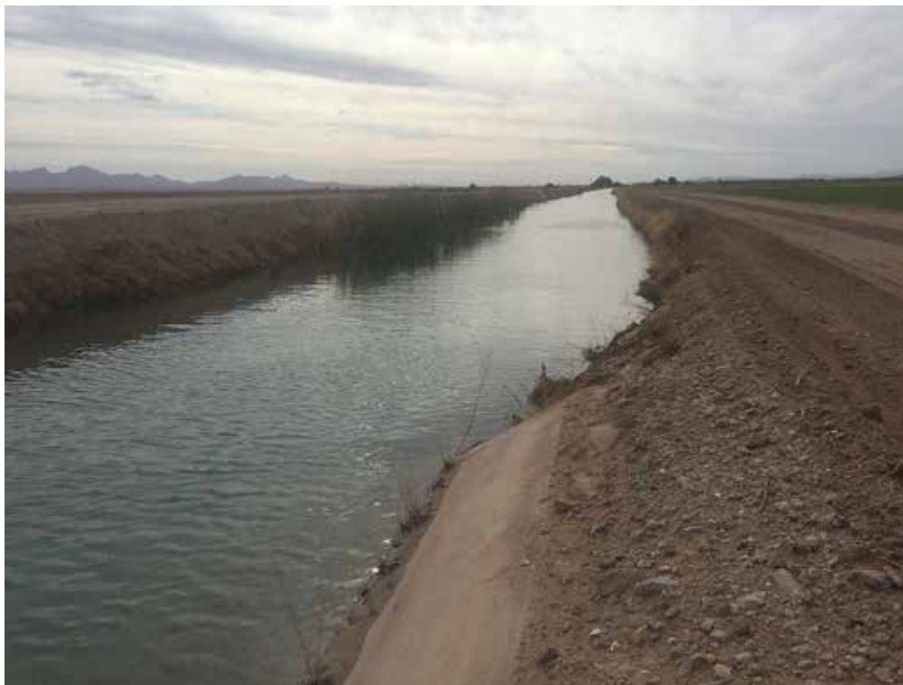
Figure 1. Termination of Current Lining on Canal D
