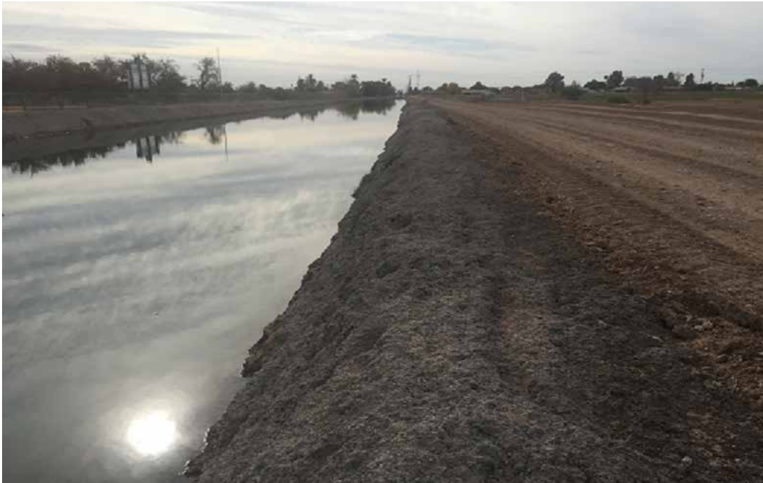
Figure 8. Example of Existing PVID Shotcrete-lined Canal
