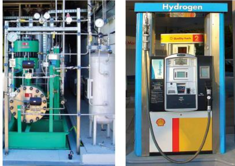
Figure 3.5 Typical Onsite Compression, Dispensing, and Storage Equipment for H 2
