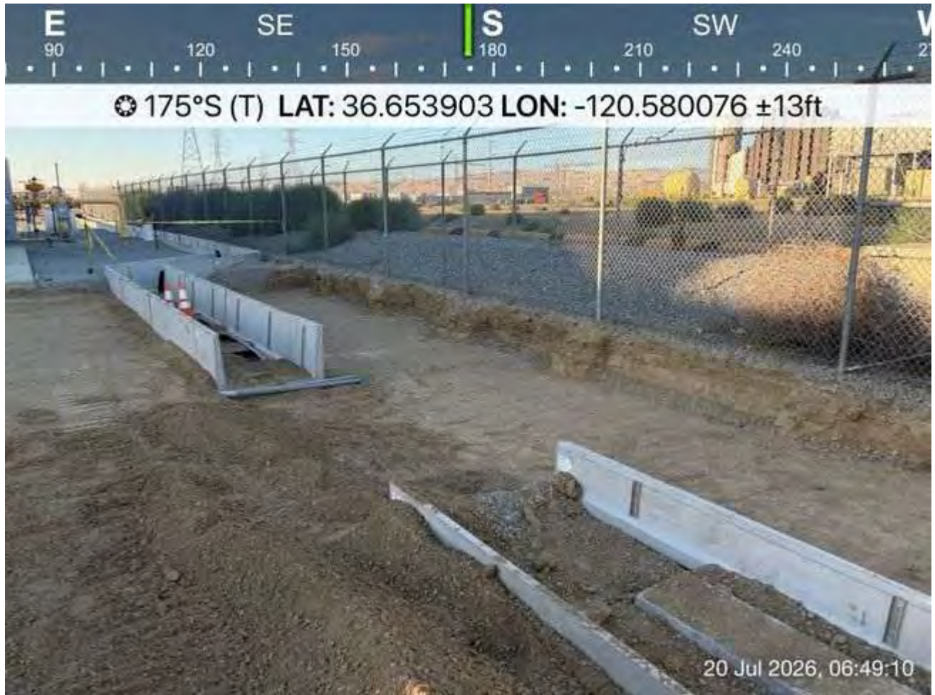
View of the work area during the pre-construction sweep.
