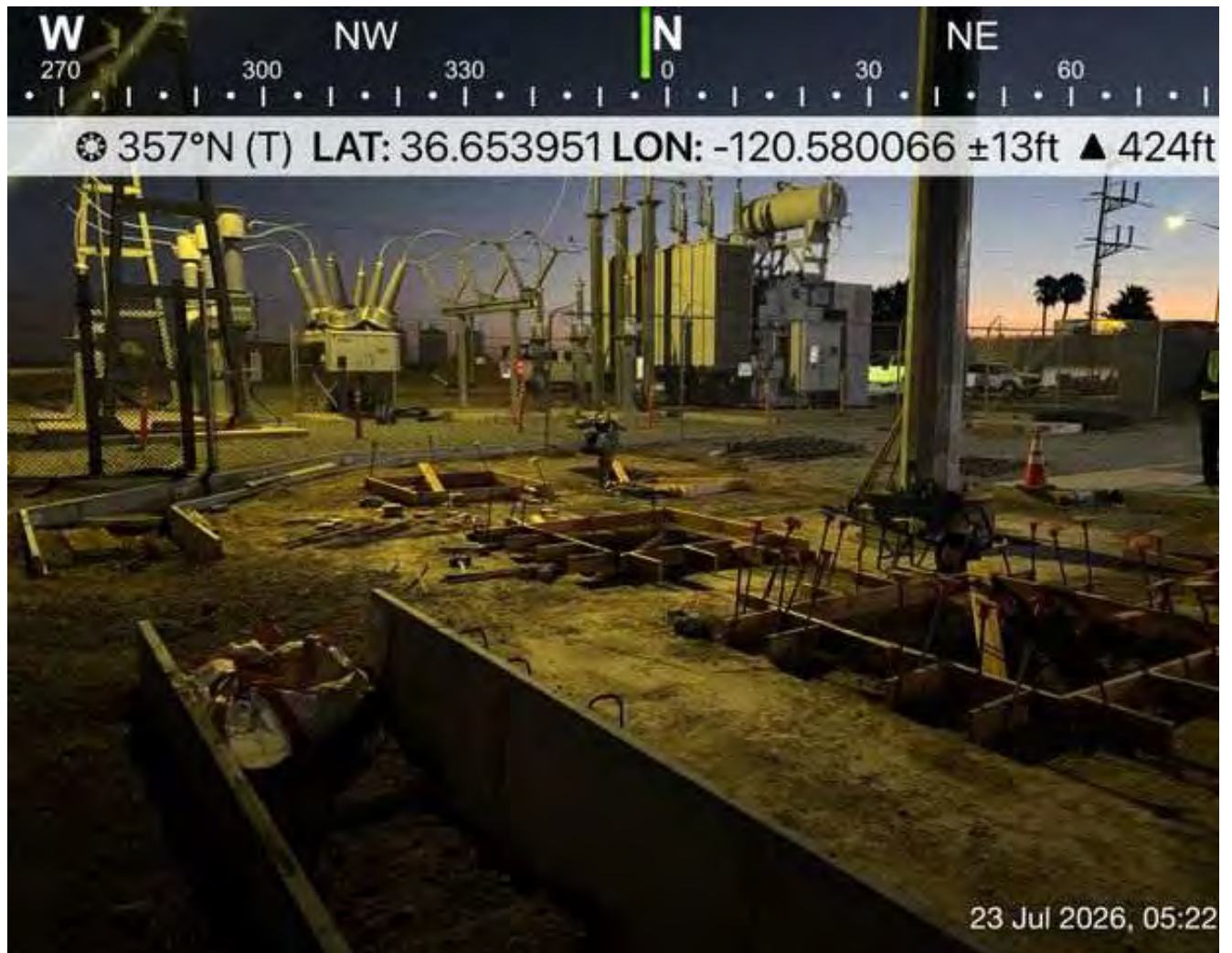
View of the work area.
