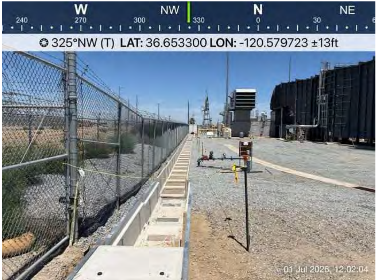
View of trench within Peaker Plant.
