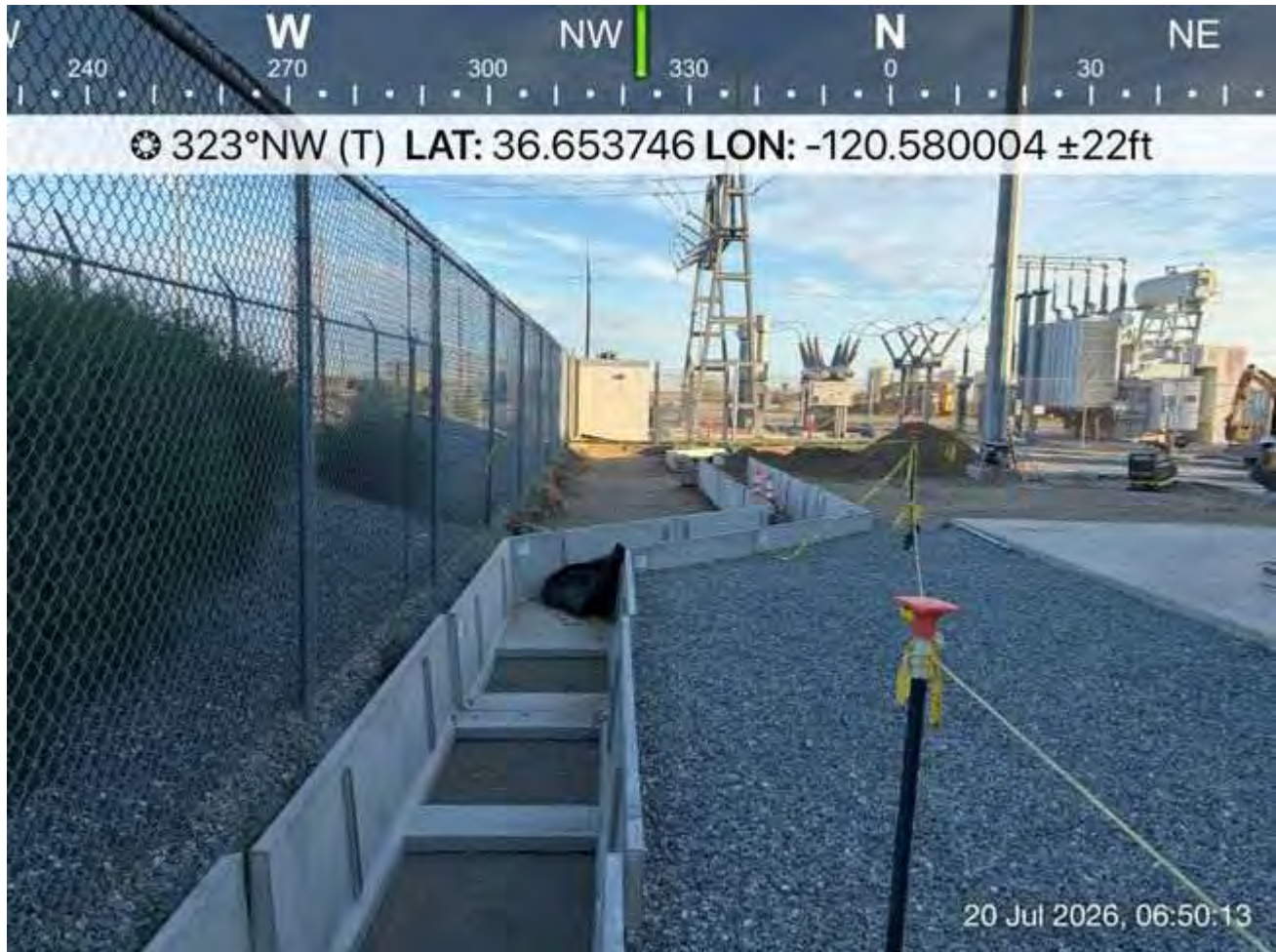
View of Gen-tie line during the pre-construction sweep.
