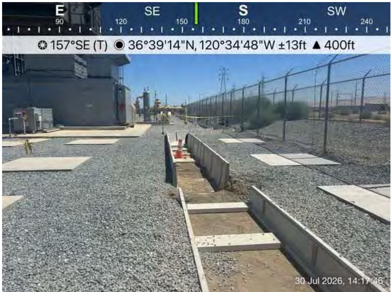
Conduit trench with ramp at end of day sweep.
