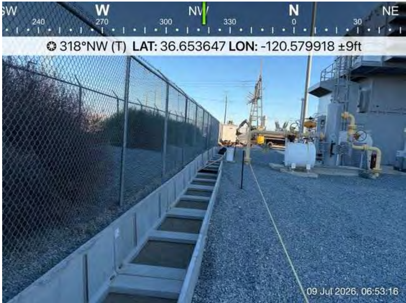
View of Gen-tie during pre-construction sweep.
