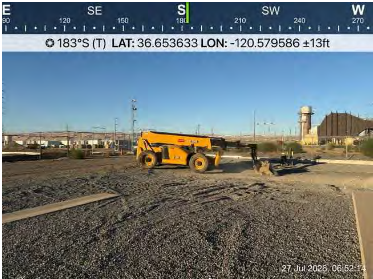
Crew moving gravel for trucks.
