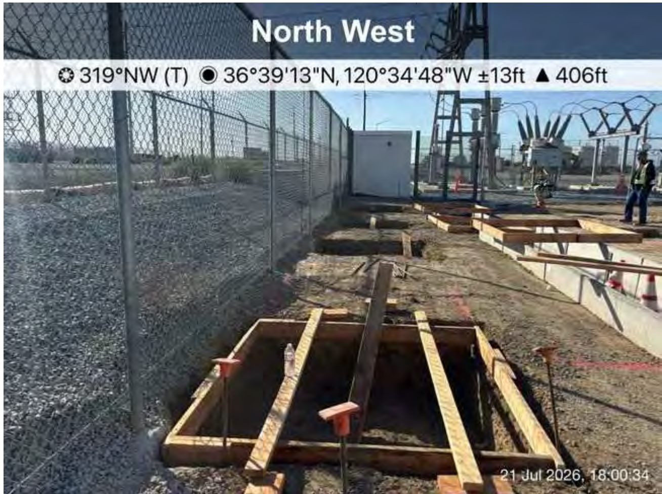
Footer holes with wooden ramps in place of each hole at end of day.
