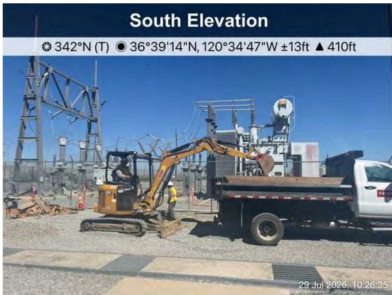
Mini excavator used to load dirt directly onto truck.
