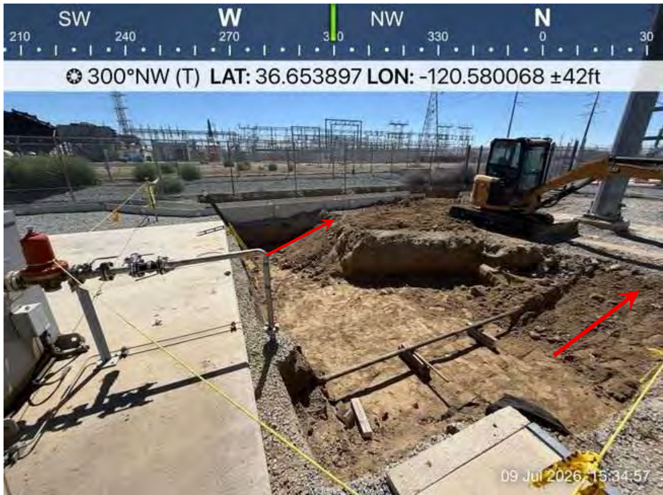
End of day progress on the trench including the wildlife ramps (arrows).
