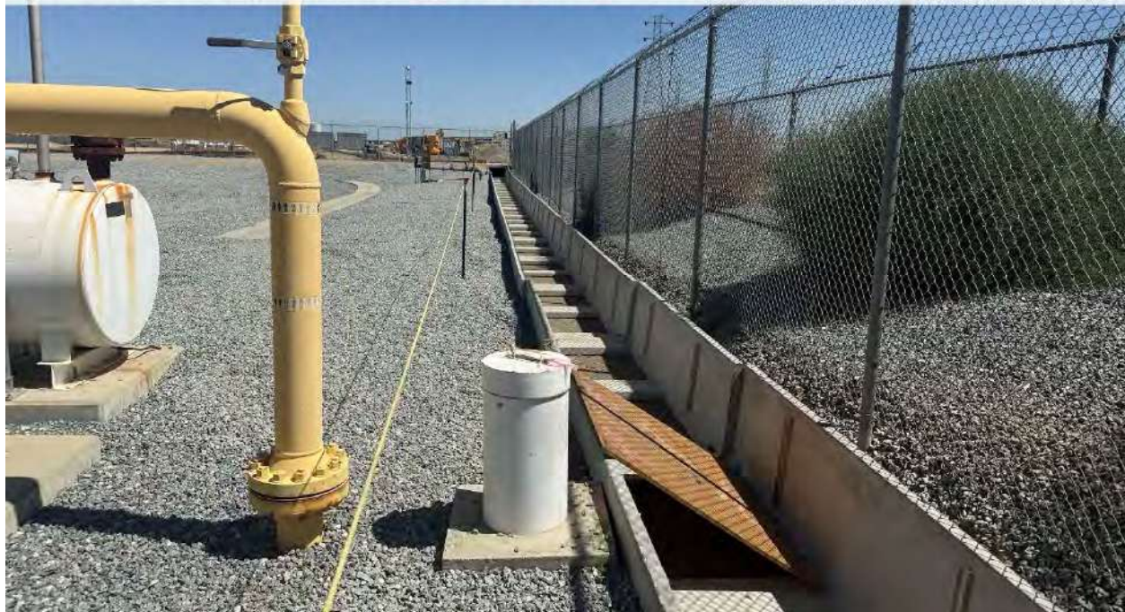
Pipes capped and escape ramps installed prior to construction crew demobilizing.
