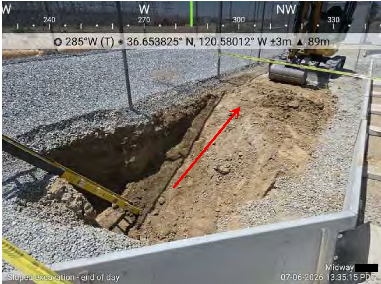
End-of-day overview of the excavation site showing the installed wildlife escape ramp (arrow) intended to prevent potential wildlife entrapment.
