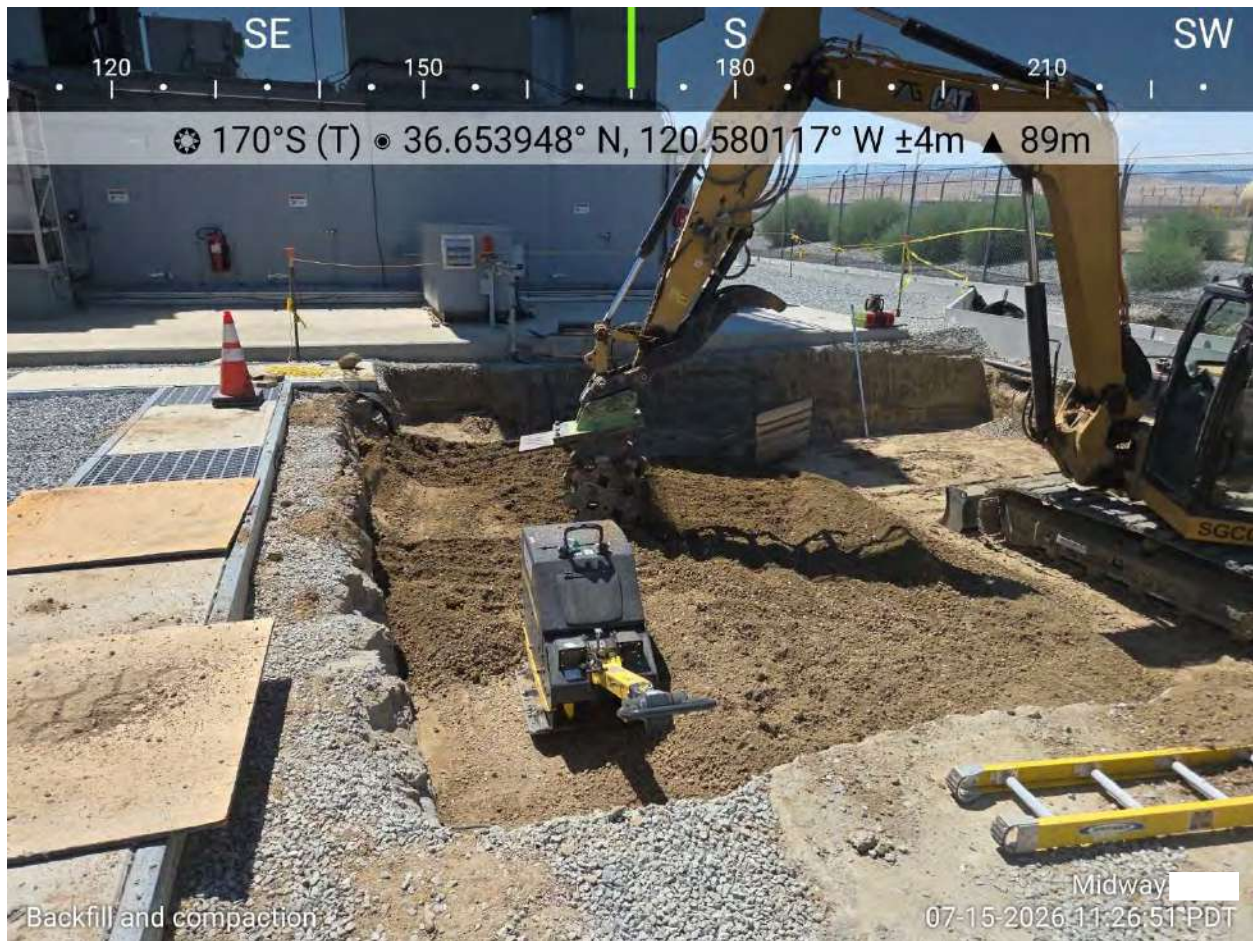
Backfilling and compaction activities.
