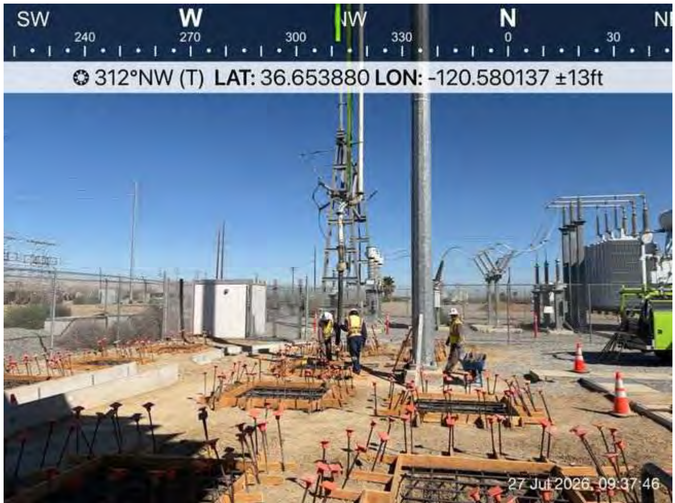
Crews pouring concrete at the pads.
