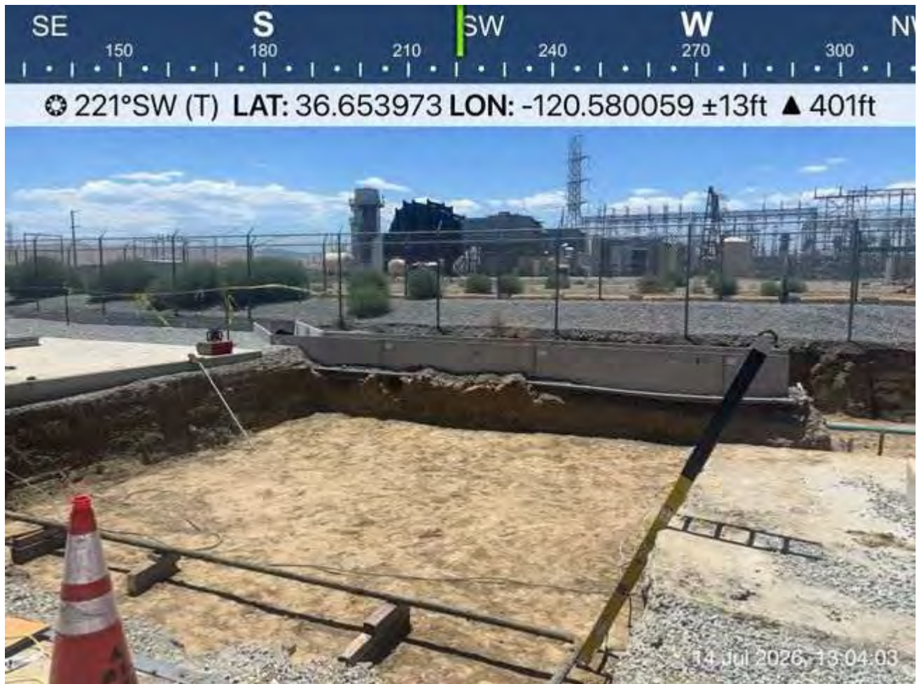
Fully excavated area.
