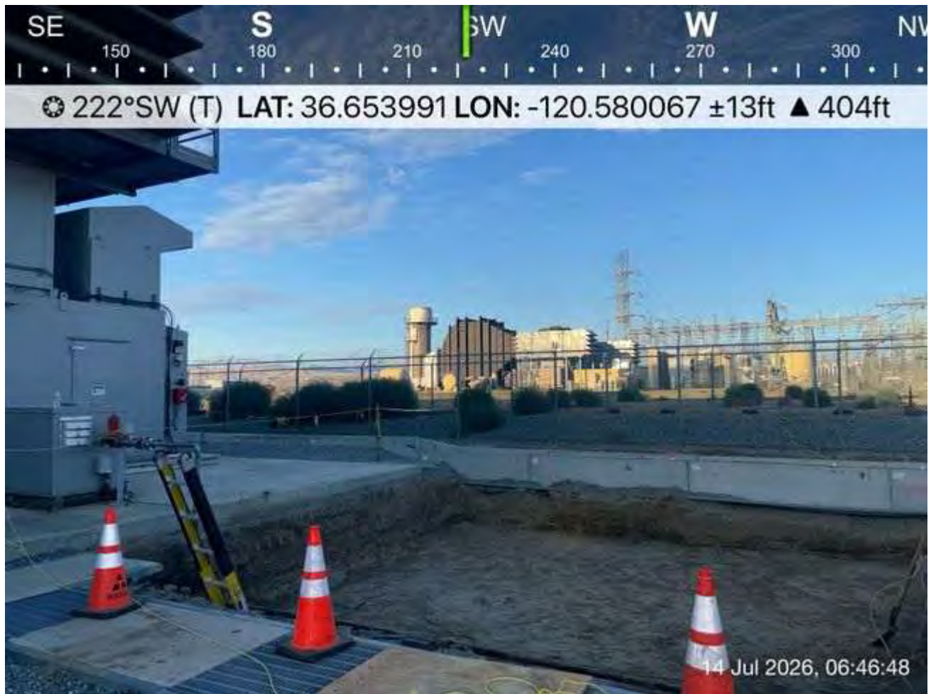
Excavated area in peaker plant.
