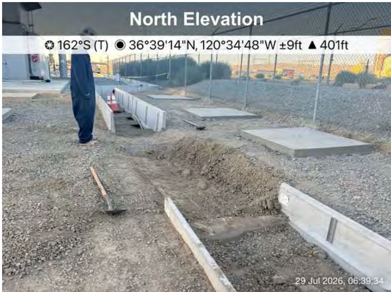
Trench with ramping at pre-activity sweep.
