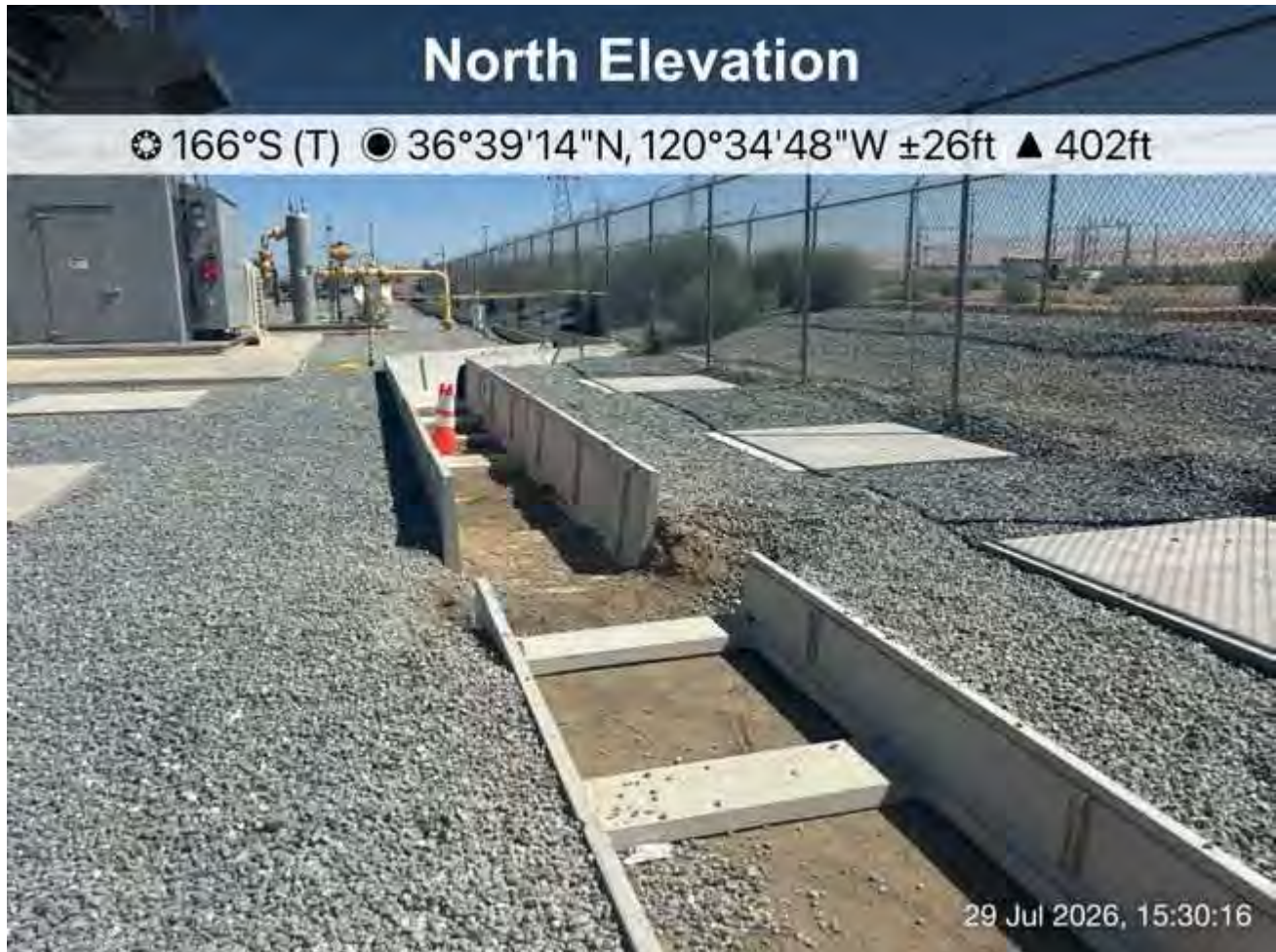
Trench with ramp out at end of day.
