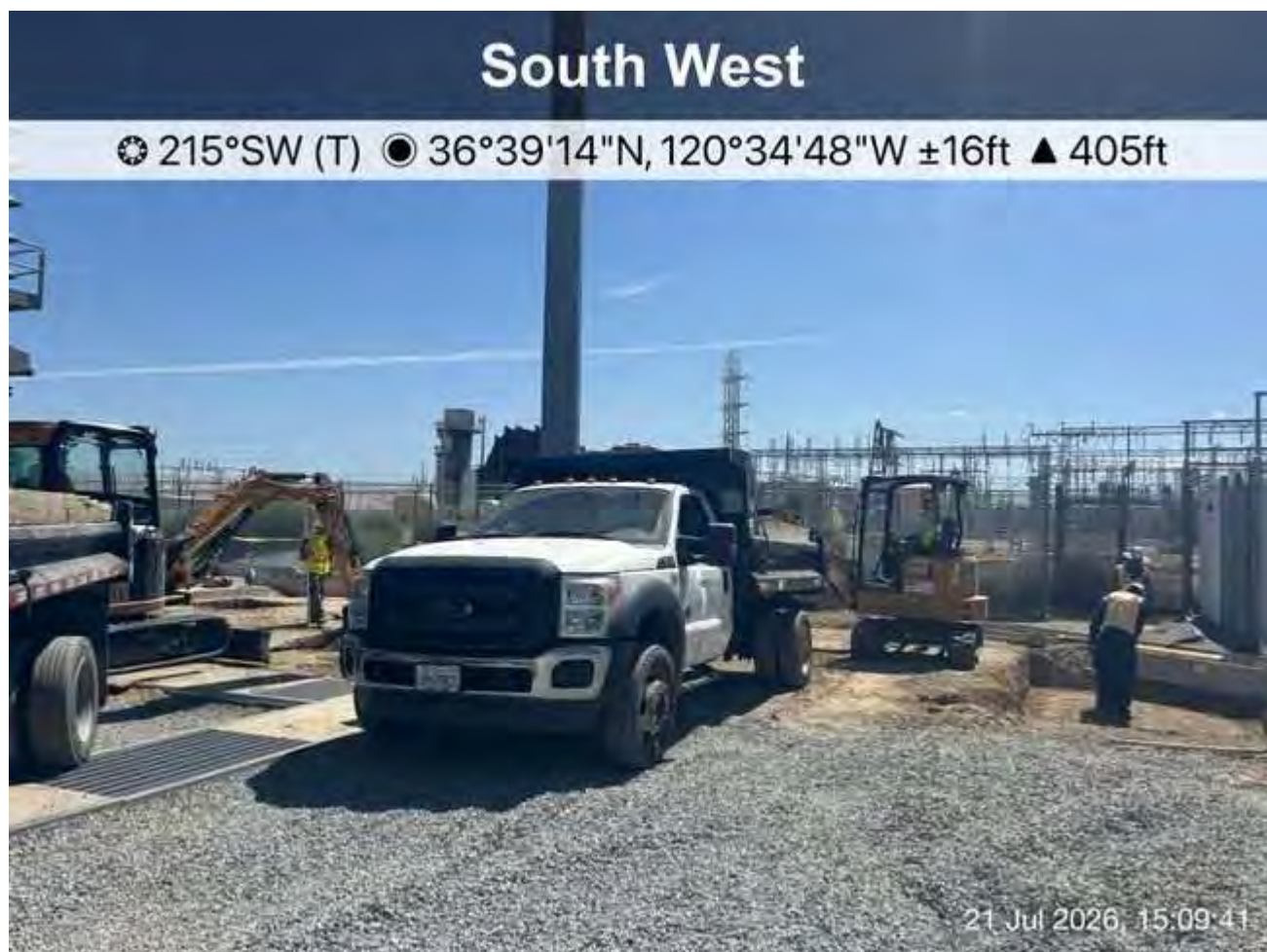
Backfill and compaction work activities.
