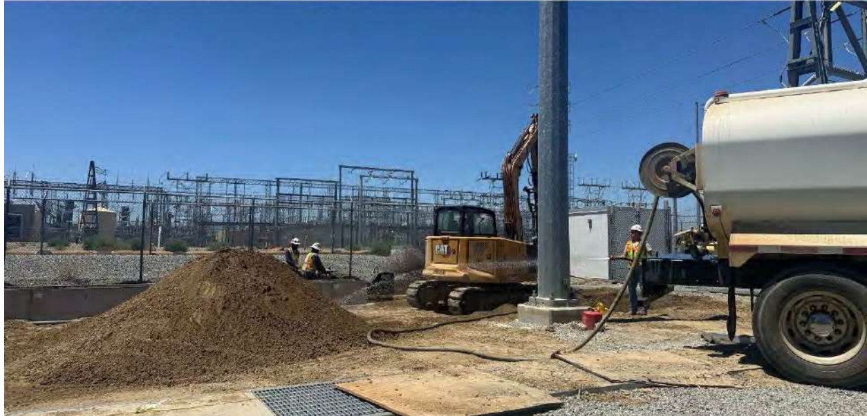
Backfill activities are ongoing with water truck present for dust suppression.
