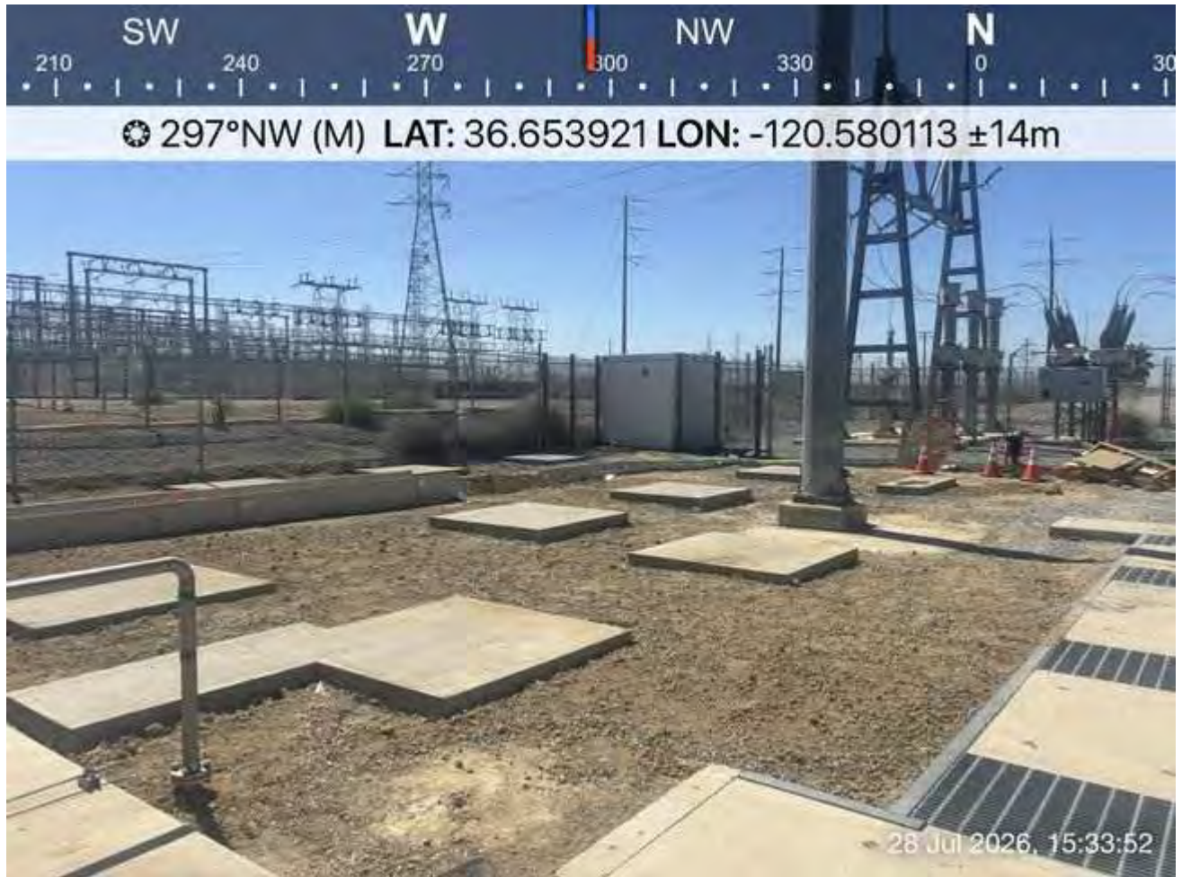
Work area within Peaker Plant at the end of day.
