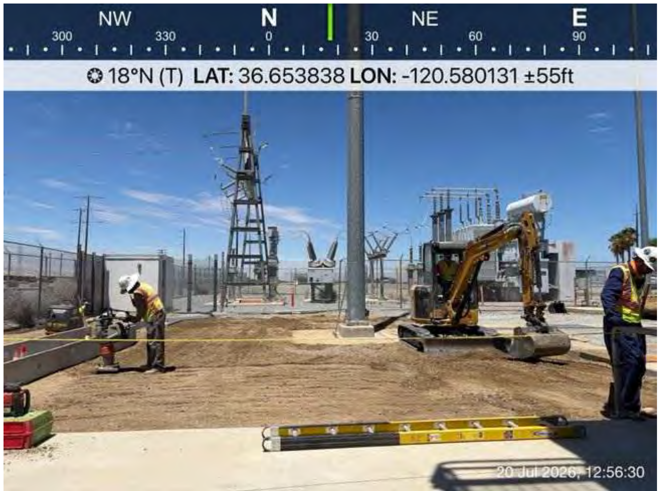
View of the crew compacting soil during backfill operations.
