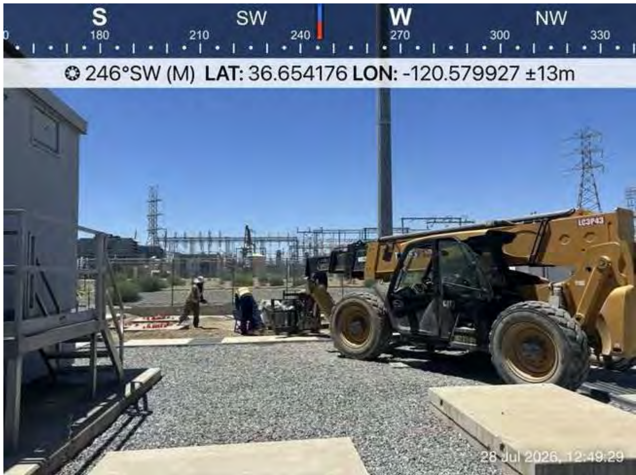
Crew removing materials from area.
