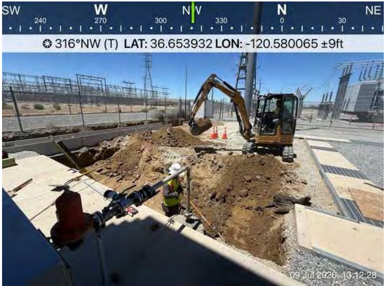
Crew excavating along the Gen-tie line.
