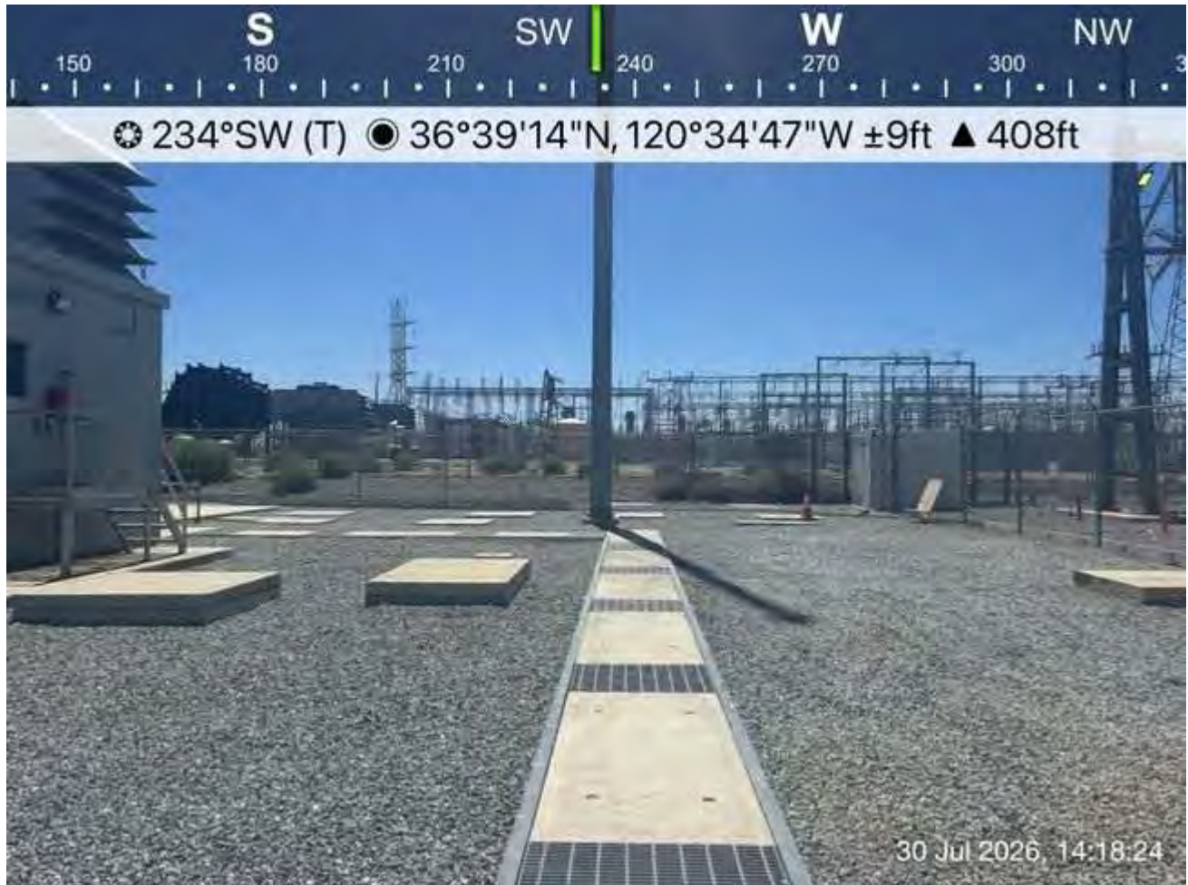
Site at end of day sweep.
