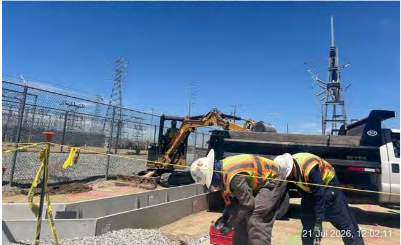
Excavation work activities for concrete footers.
