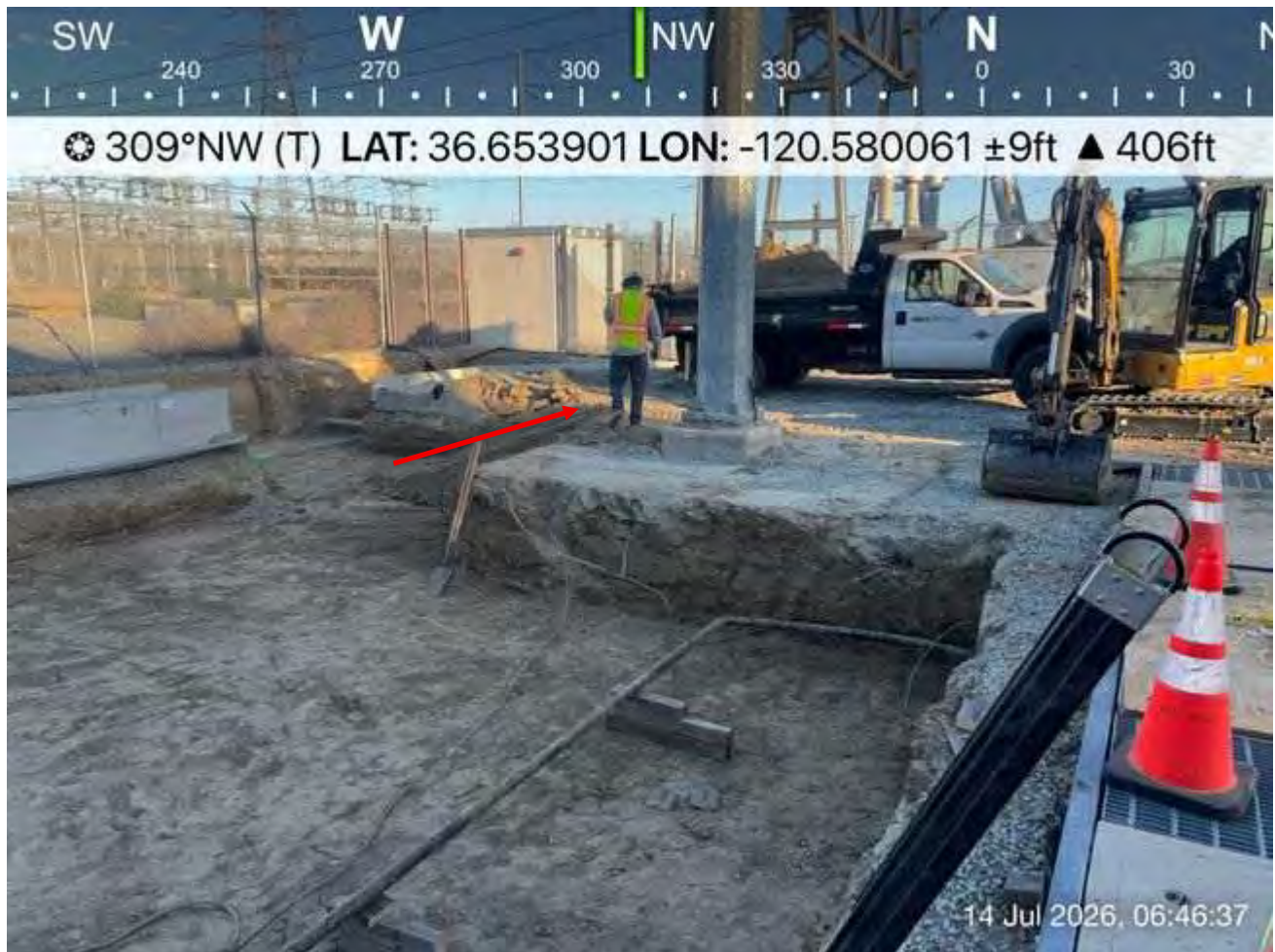
Excavated area in peaker plant. Adequate earthen ramp in place (red arrow).
