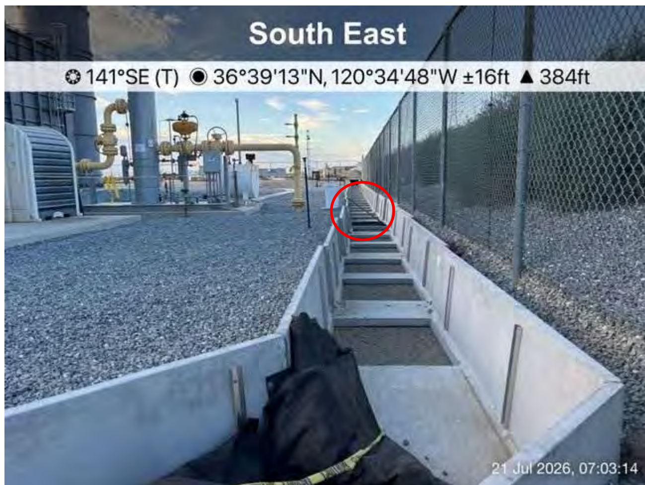
Trench with adequate ramping to prevent wildlife entrapment during pre-activity sweep.
