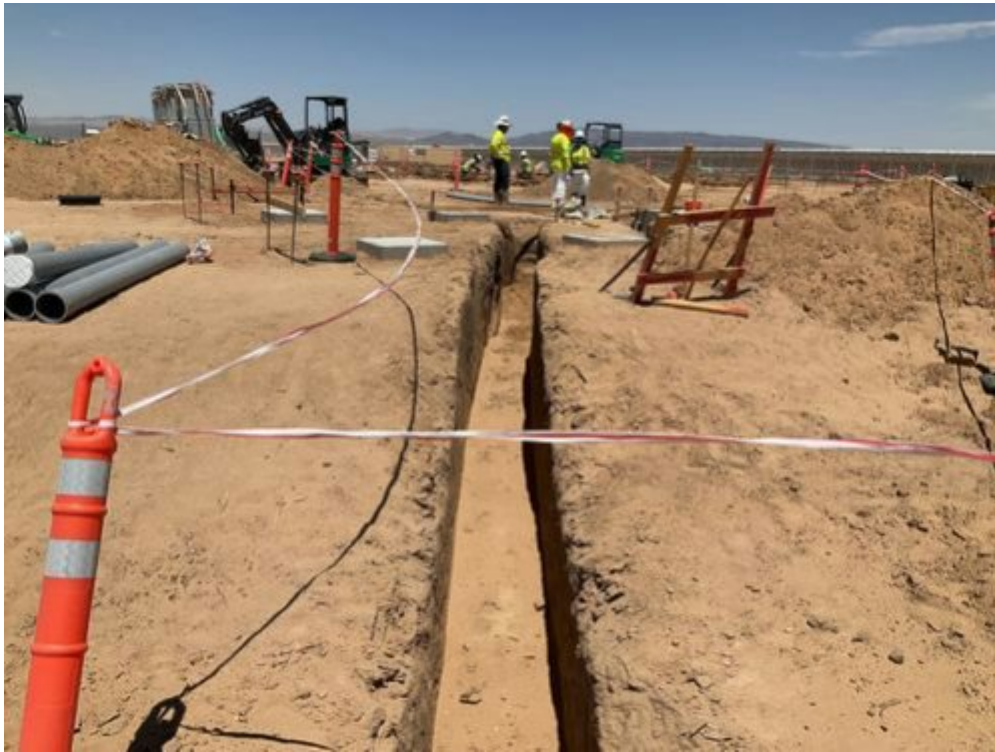
Photo Direction: West Location: 35.01129347222222,- 117.34954144444444 Date: 2026/05/13 Time: 13:11:17 Trench in substation for line installation, ~30 inches.
