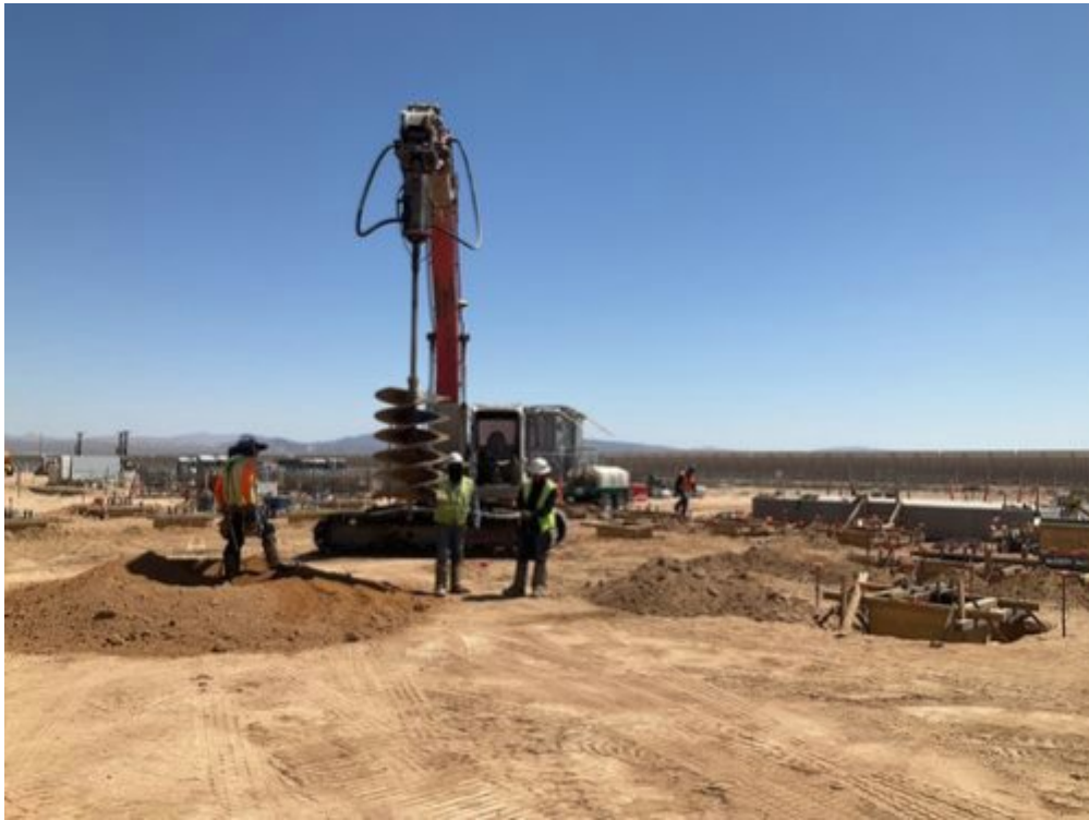
Photo Direction: Northeast Location: 35.01154533333333,- 117.34972624999999 Date: 2026/05/22 Time: 10:57:33 Boring for pier installation; loamy sand
