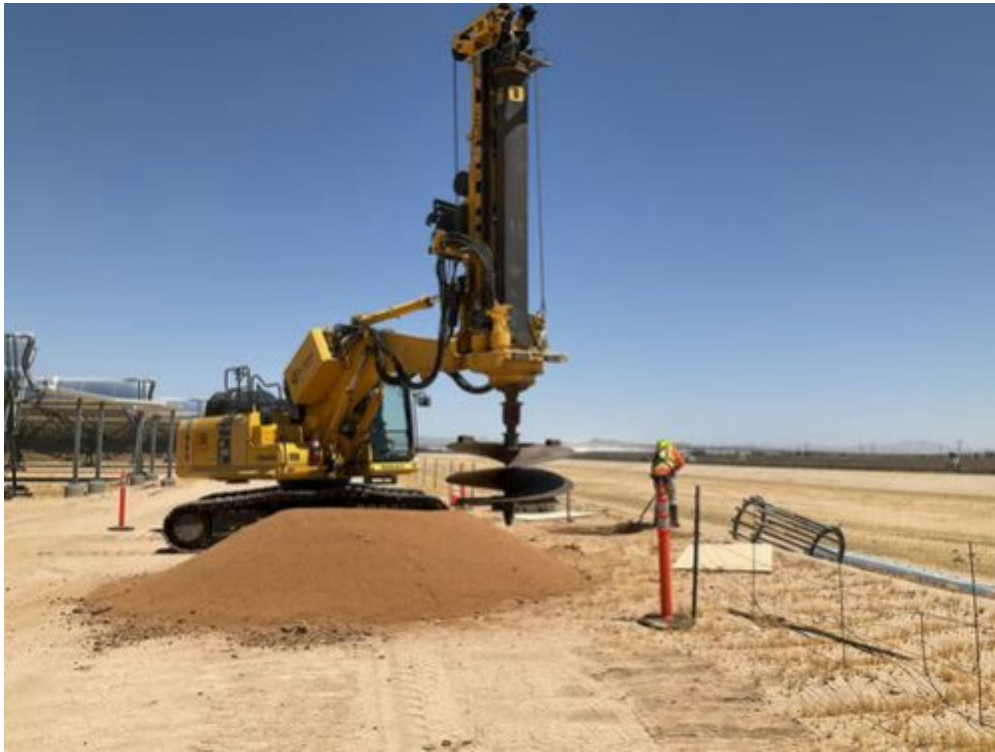
Photo Direction: South Location: 35.01183422222222,- 117.34520023333333 Date: 2026/05/14 Time: 13:46:13 Drill rig boring for pole installation; loamy sand
