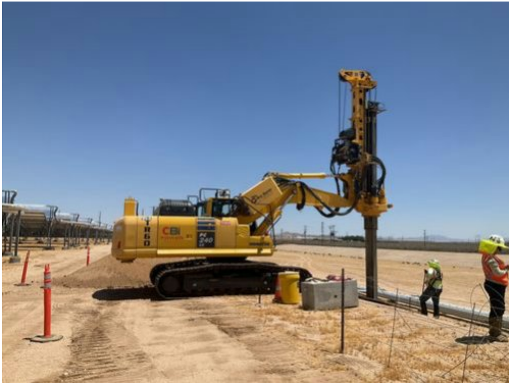
Photo Direction: East Location: 35.01171605555555,-117.33343680972222 Date: 2026/05/28 Time: 13:12:47 Drill rig boring for pole installation; loamy sand
