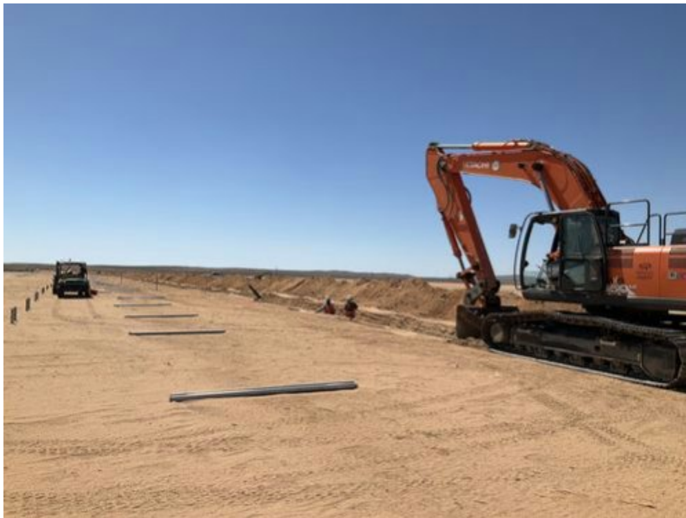
Photo Direction: South Location: 35.01104863888889,- 117.3533557611111 Date: 2026/05/11 Time: 15:06:11 Excavator trenching for MV line.
