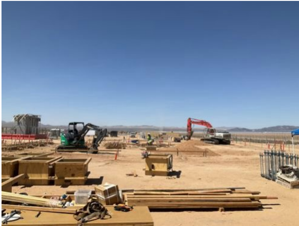
Photo Direction: Southwest Location: 35.01137141666667,- 117.34922177777777 Date: 2026/05/11 Time: 14:58:12 Drill rig parked after boring holes in the morning.
