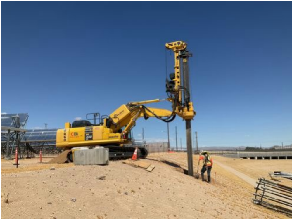
Photo Direction: Northeast Location: 35.011642333333334,- 117.33167013888888 Date: 2026/05/29 Time: 14:46:19 Drill rig boring for pole installation; loamy sand
