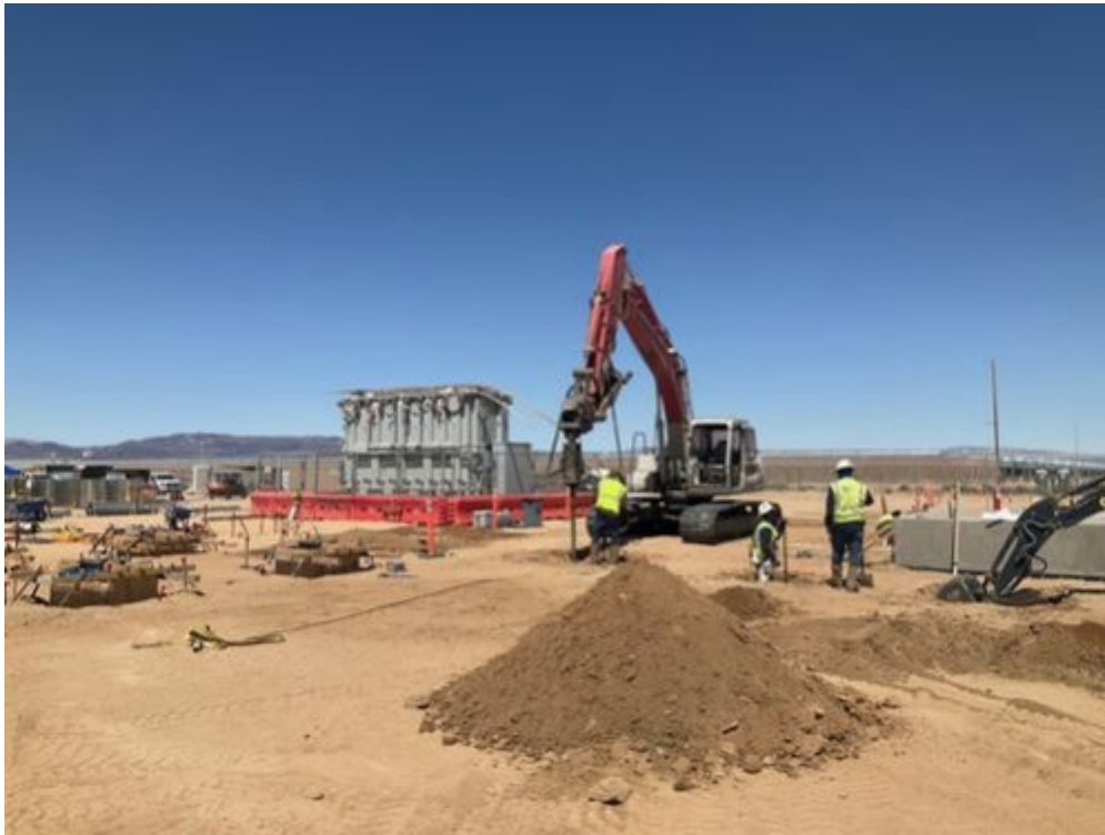
Photo Direction: West Location: 35.011478805555555,- 117.34956747222222 Date: 2026/05/19 Time: 14:38:15 Drill rig boring for pier installation; loamy sand
