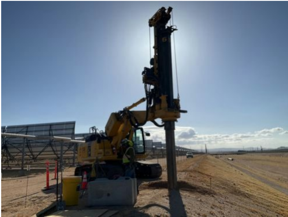
Photo Direction: Northwest Location: 35.01166747222222,- 117.33674375 Date: 2026/05/27 Time: 07:53:00 Drill rig boring for T-line; loamy sand
