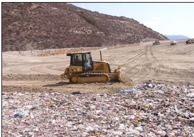
Figure 22 - Bulldozer placing cover soil on exposed waste.
