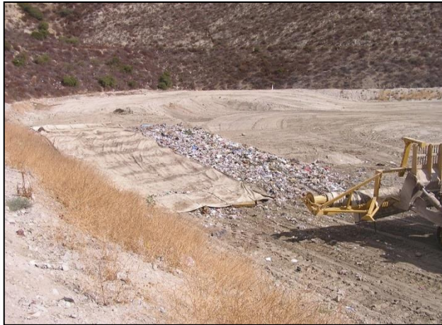
Figure 23 - Bulldozer placing ADC (tarp) on exposed waste.
