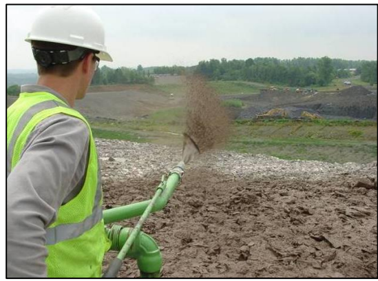
Figure 27 - Spray-on cement-based ADC.
