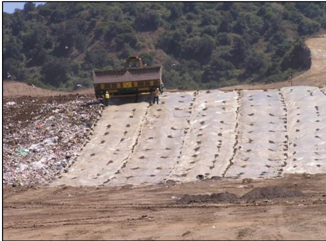
Figure 26 - Disposable film applied as ADC.
