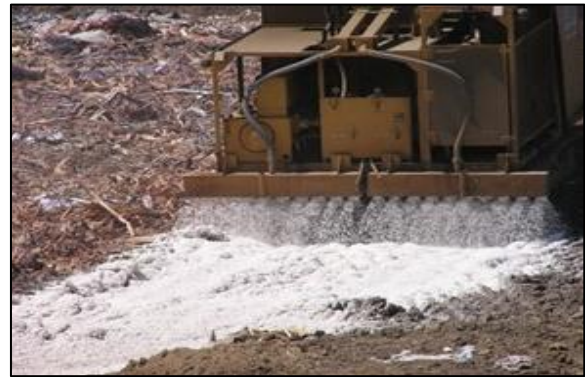
Figure 24 - Spray-on Foam ADC.
