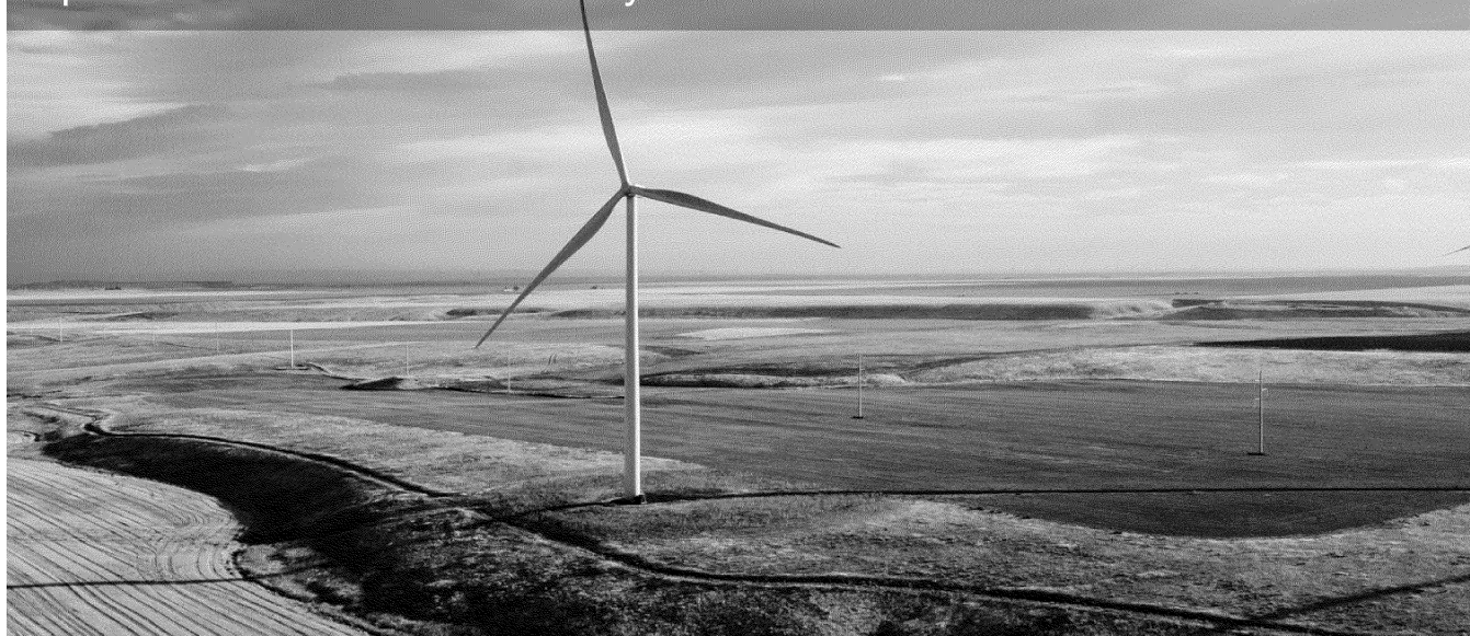
The Wheatridge Renewable Energy Center in Morrow County, Oregon is the first large-scale energy facility in North America to combine wind, solar and battery energy storage at a single location.
