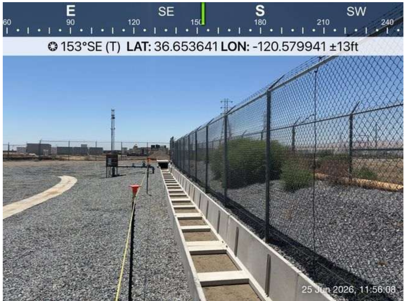
End of Gen-tie trench facing south towards the BESS.
