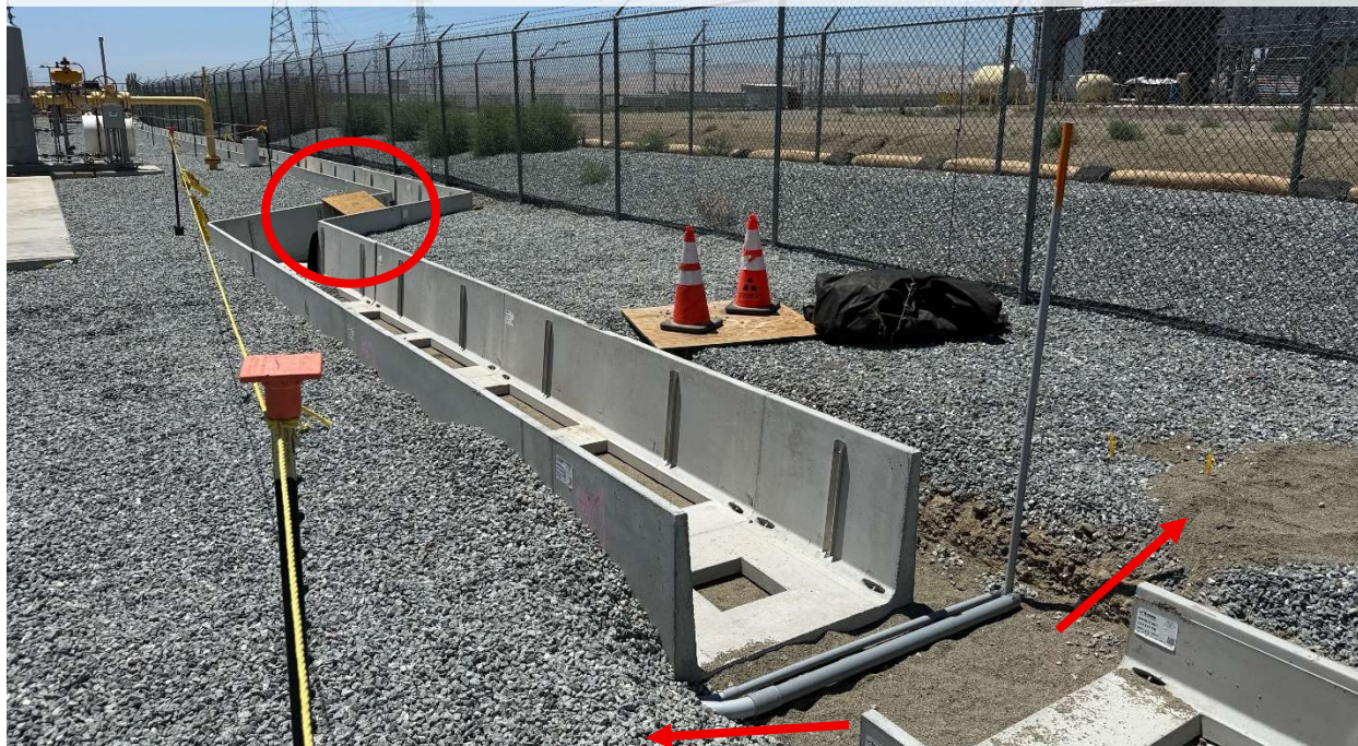
Trench in MPP area; earthen escape ramps and boards present throughout and at midpoint (shown).
