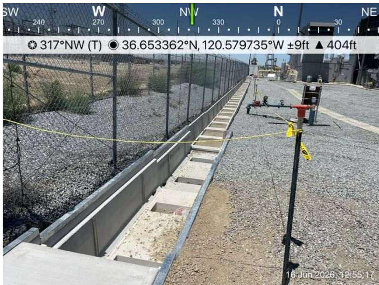
Work area along Midway Peaker Plant fenceline
