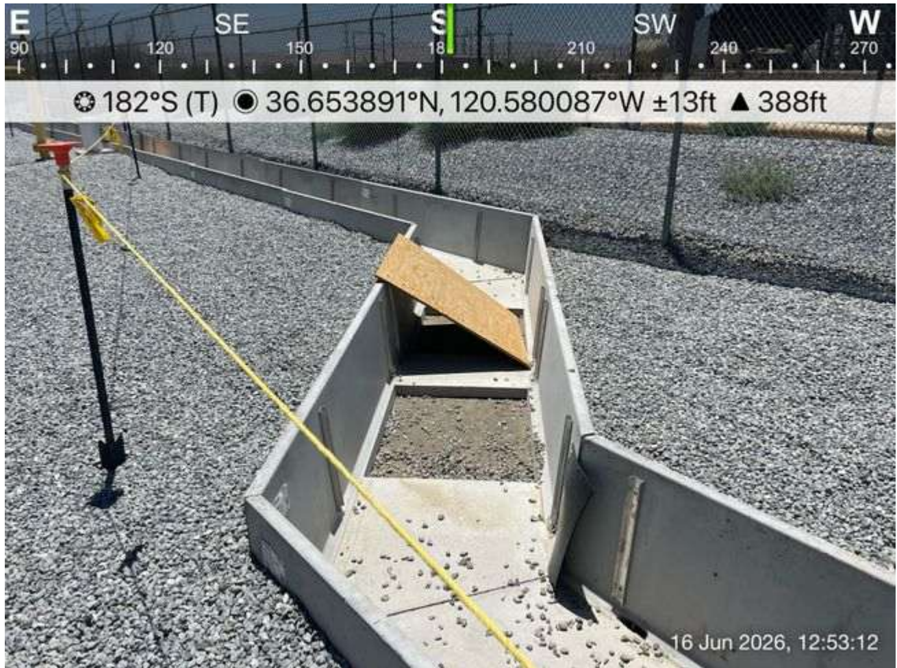
Wildlife escape ramp within trench
