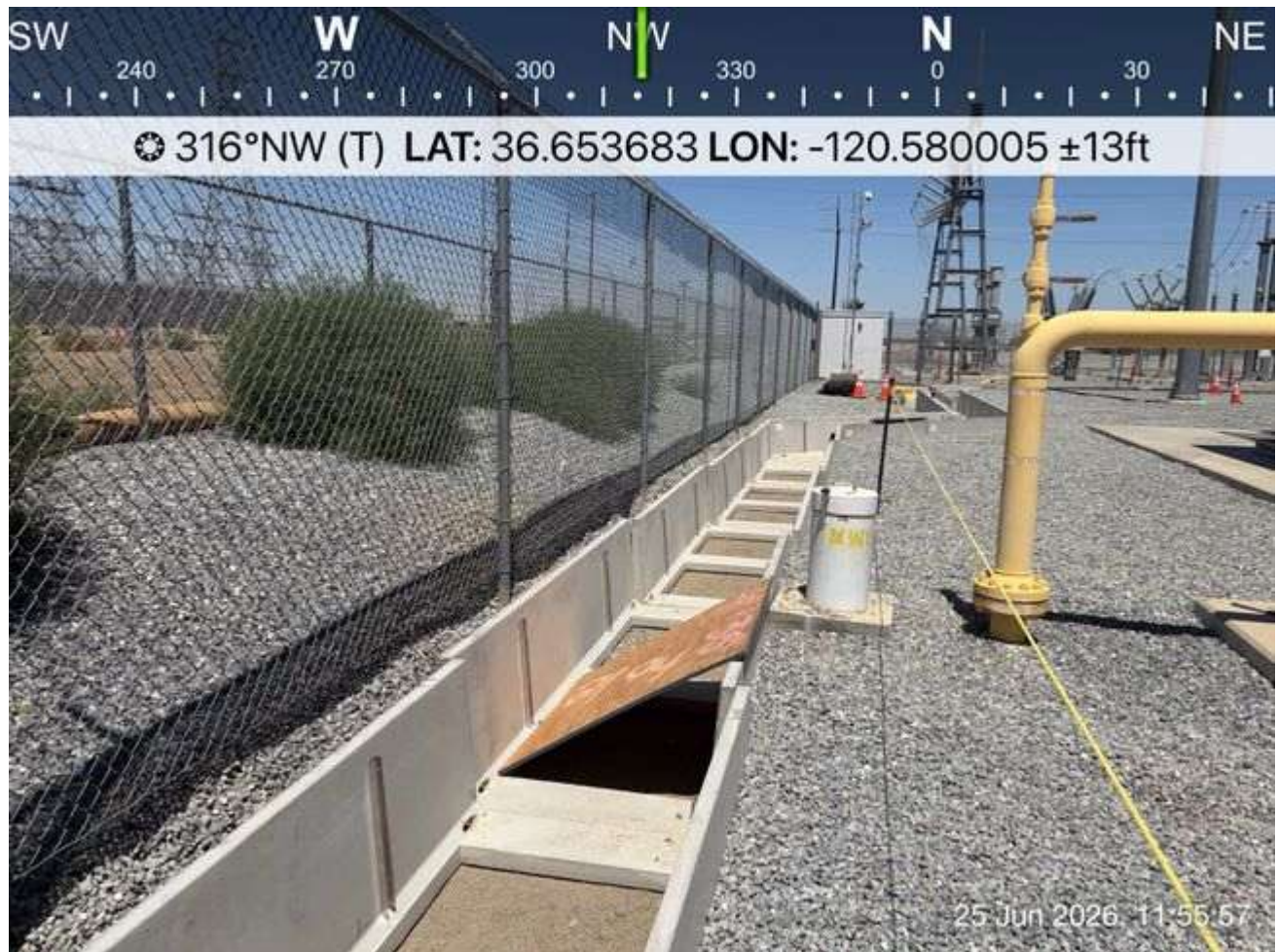
Gen-tie trench with boards.
