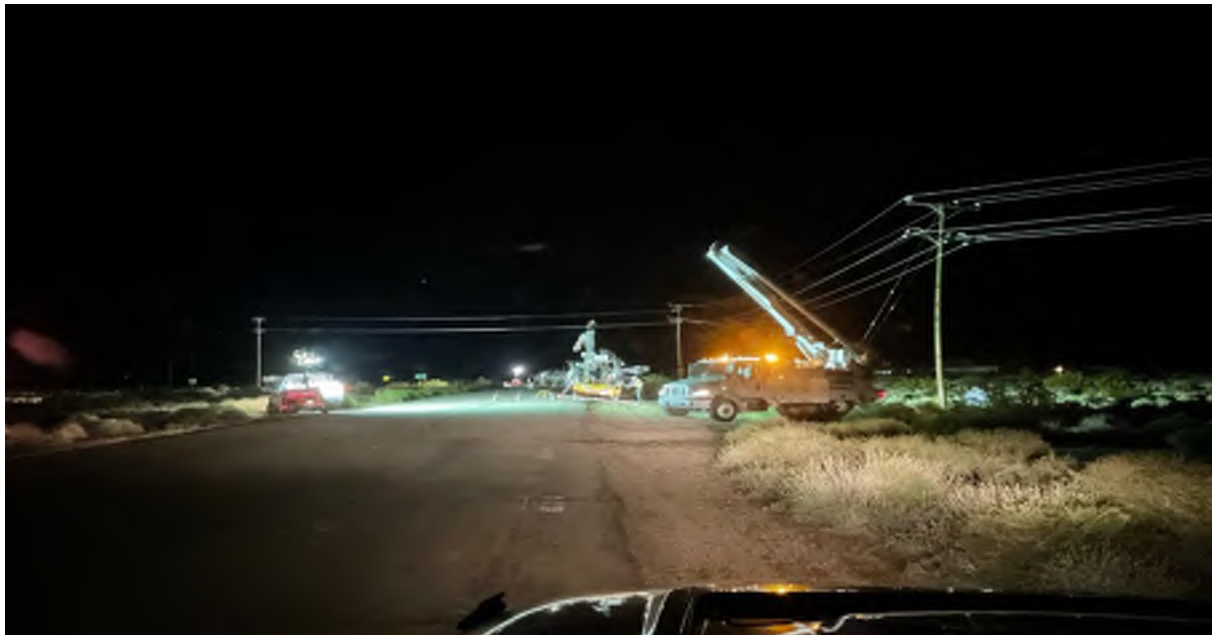
Photo 2. Line removal at poles 115E, 116E, and 117E, facing north. Taken by Curtis Uptain on April 14, 2024.
