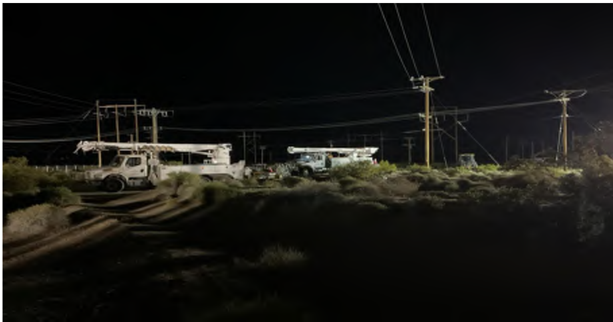
Photo 2. Work area N of substation, facing north. Photograph taken by Curtis Uptain on May 1, 2024.
