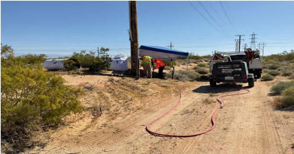
Photo 3. Crew hand-digging hole for replacement of pole 2025110E, facing east. Taken by Curtis Uptain on April 12, 2024.
