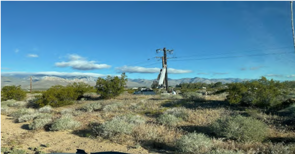
Photo 4. Pole replacement at 110E, facing north. Taken by Curtis Uptain on April 14, 2024.
