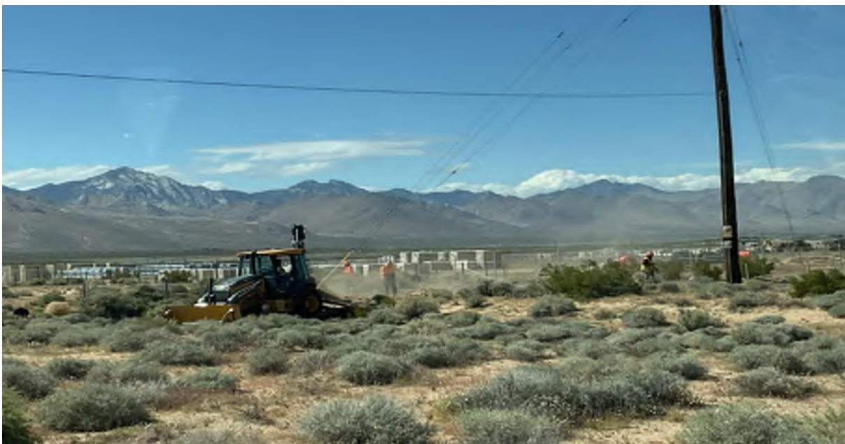
Photo 4. Excavating for anchor installation at pole 2025118E, facing northwest. Taken by Curtis Uptain on April 12, 2024.
