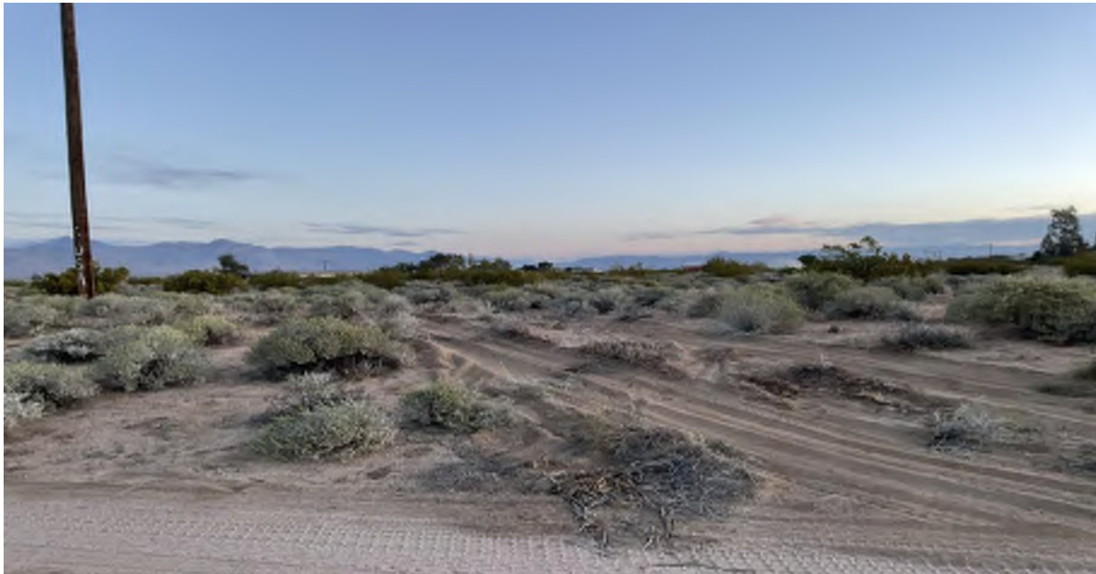
Photo 3. Access road into pole 2025114e before access track was repaired. GPS coordinates 35.654282°N, -117.802255°W, facing northwest. Taken by Danielle Temple on April 24, 2024.
