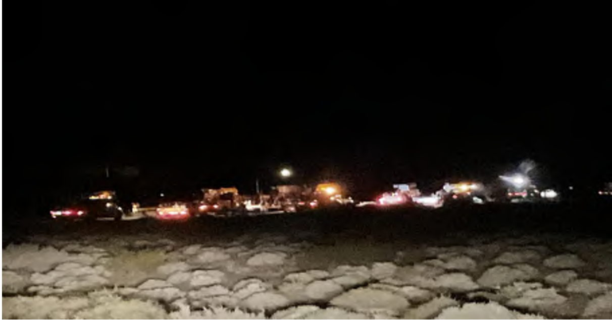
Photo 1. Work crew staged along Clodt road preparing to start work, north. Taken by Curtis Uptain on April 14, 2024.
