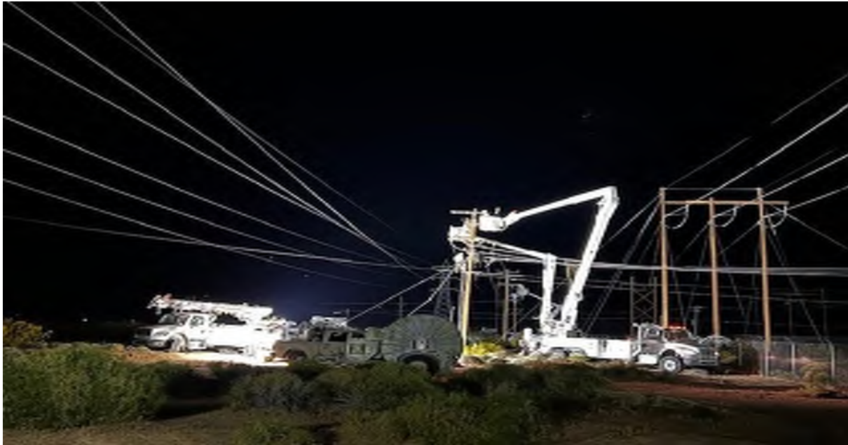
Photo 1. Replacing cross arms on pole 4028512E, facing north. GPS Coordinates: 35.65296, -117.79603. Taken by Brittany Gummo, 05/02/2024.
