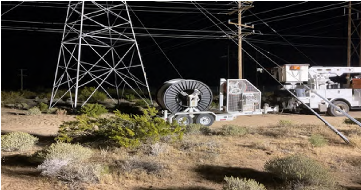
Photo 2. Laying cable from pole 306 to the west. Taken by Curtis Uptain on April 24, 2024.
