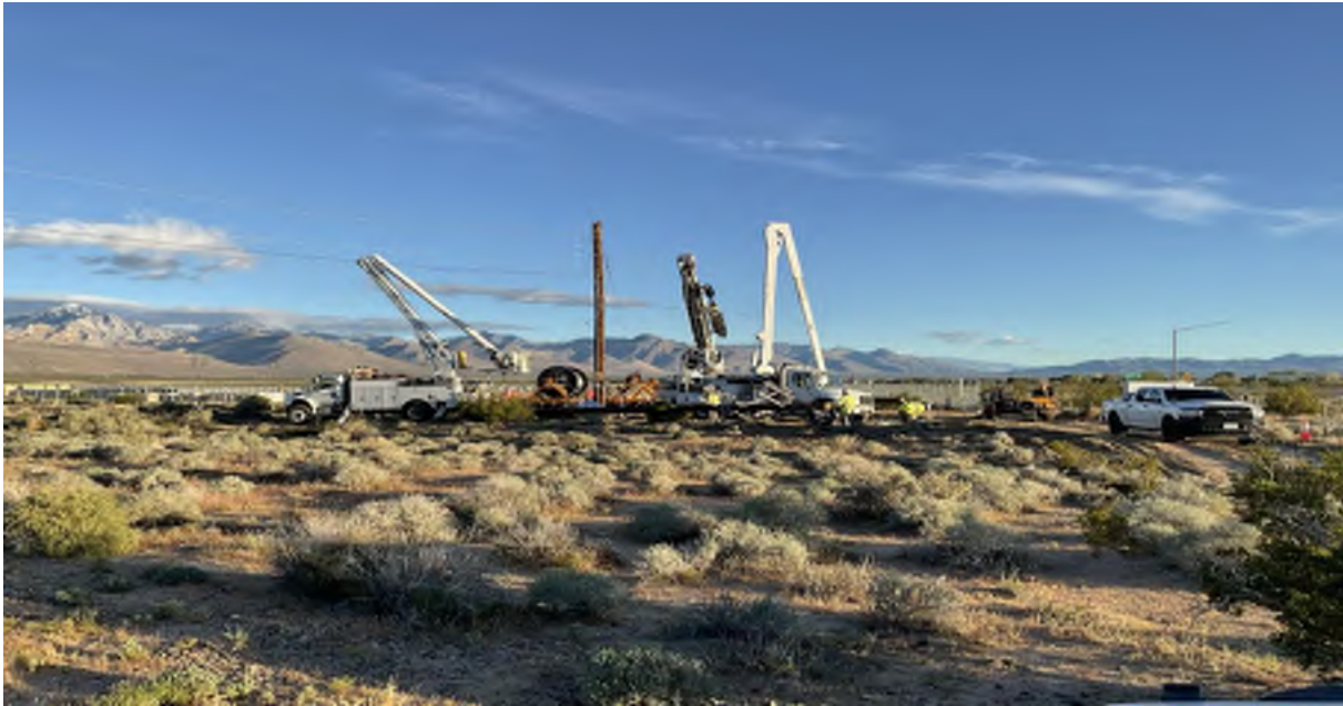
Photo 3. Pole replacement at 118E, facing north. Taken by Curtis Uptain on April 14, 2024.
