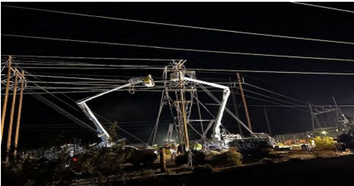
Photo 2. Pulling and Stringing power cable, facing northeast. GPS Coordinates: 35.65334, -117.79651 Photograph taken by Brittany Gummo on May 2, 2024.
