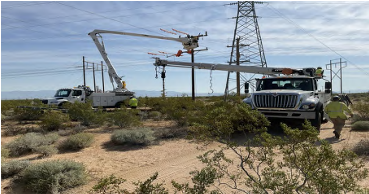
Photo 1. Pole replacement at 2025148E, facing northwest. Taken by Curtis Uptain on April 22, 2024.
