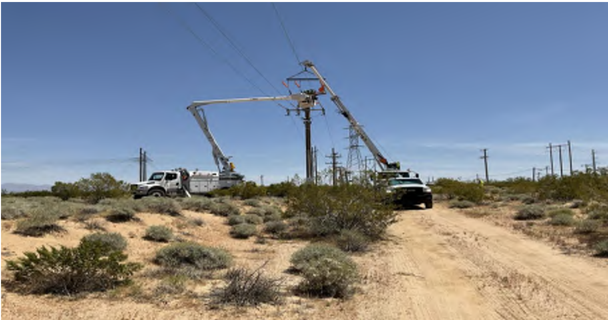
Photo 2. Arm replacement at pole 109E, facing east. Taken by Curtis Uptain on April 22, 2024.
