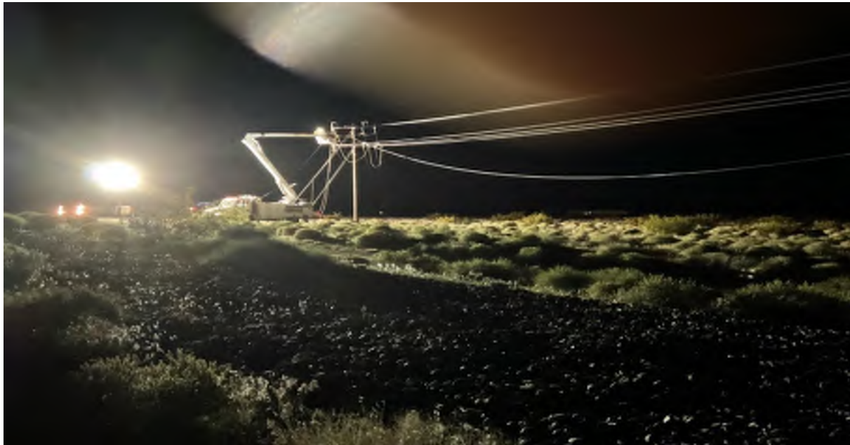
Photo 2. Stringing line from start point at pole 2025115E. GPS coordinates 35.654107°N, -117.801974°W, facing northeast. Taken by Danielle Temple on April 24, 2024.
