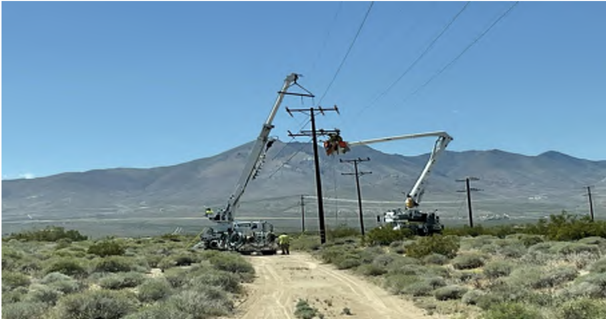
Photo 3. Arm replacement at 113E, facing west. Taken by Curtis Uptain on April 22, 2024.
