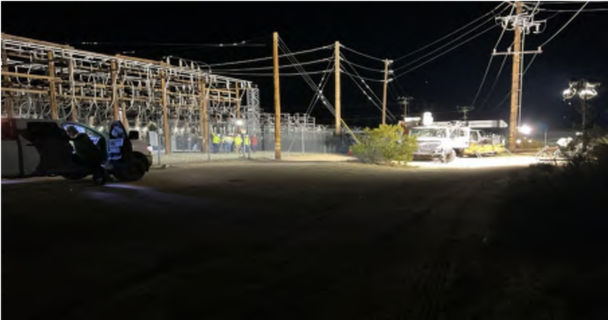
Photo 1. Work area east of substation, facing northwest. Photograph taken by Curtis Uptain on May 1, 2024.
