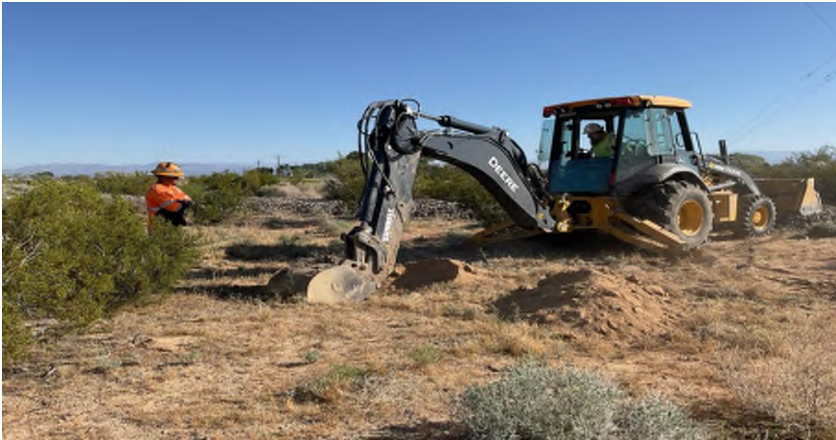
Photo 1. Crew digging an 8ft hole at 2025117E for a new anchor point. Taken by Karissa Denney on April 23, 2024.
