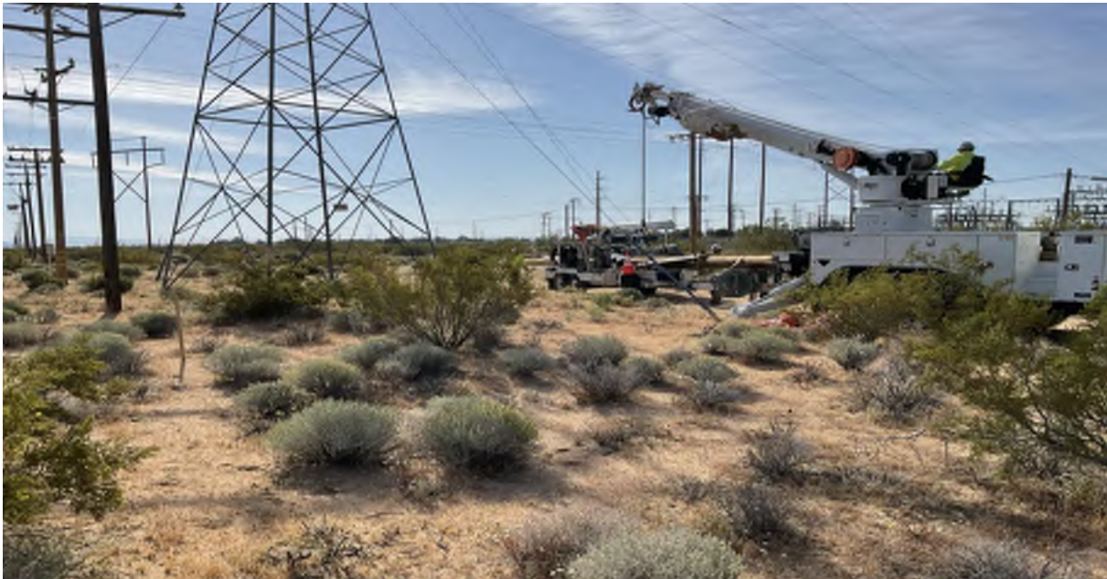
Photo 4. Arm replacement at pole 836E, facing northeast. Taken by Curtis Uptain on April 22, 2024.
