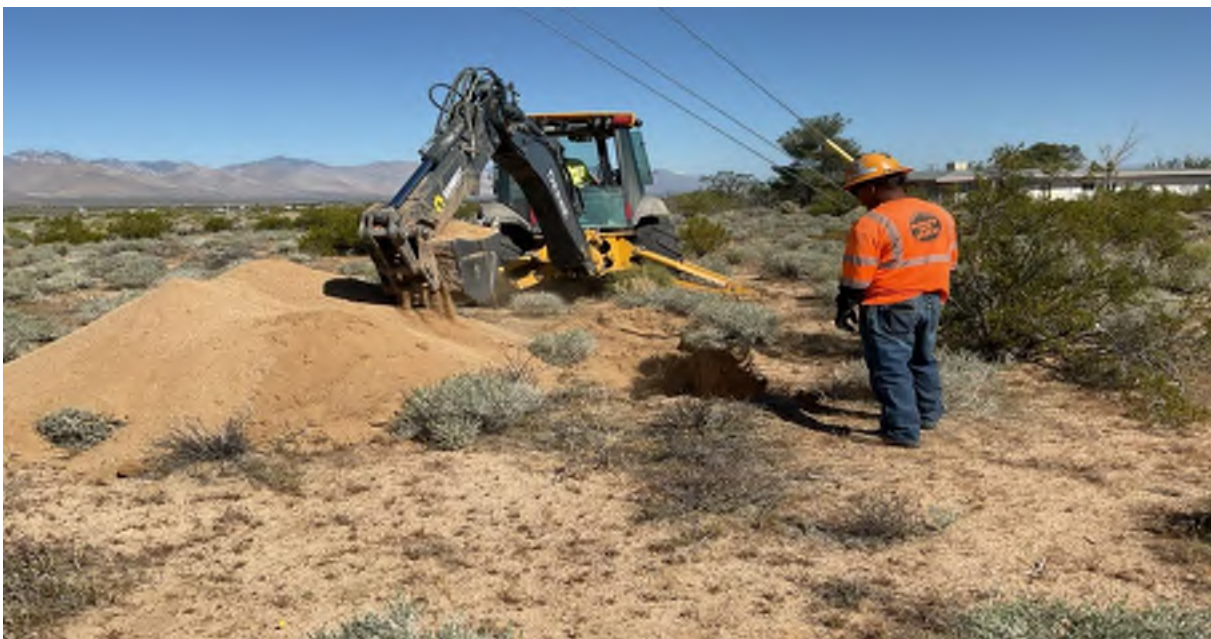
Photo 2. Crew digging pit at pole 2025116E for anchor, north. Taken by Curtis Uptain on 04/13/2024.
