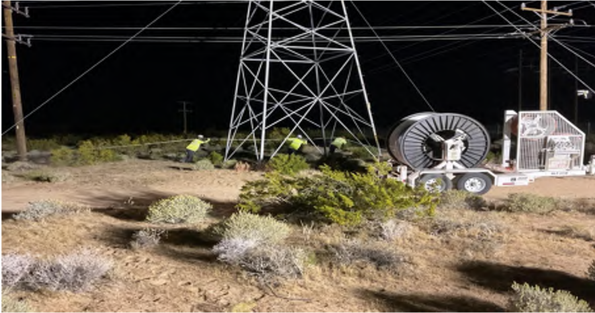
Photo 1. Laying cable from pole 306 to the west, facing north. Taken by Curtis Uptain on April 24, 2024.
