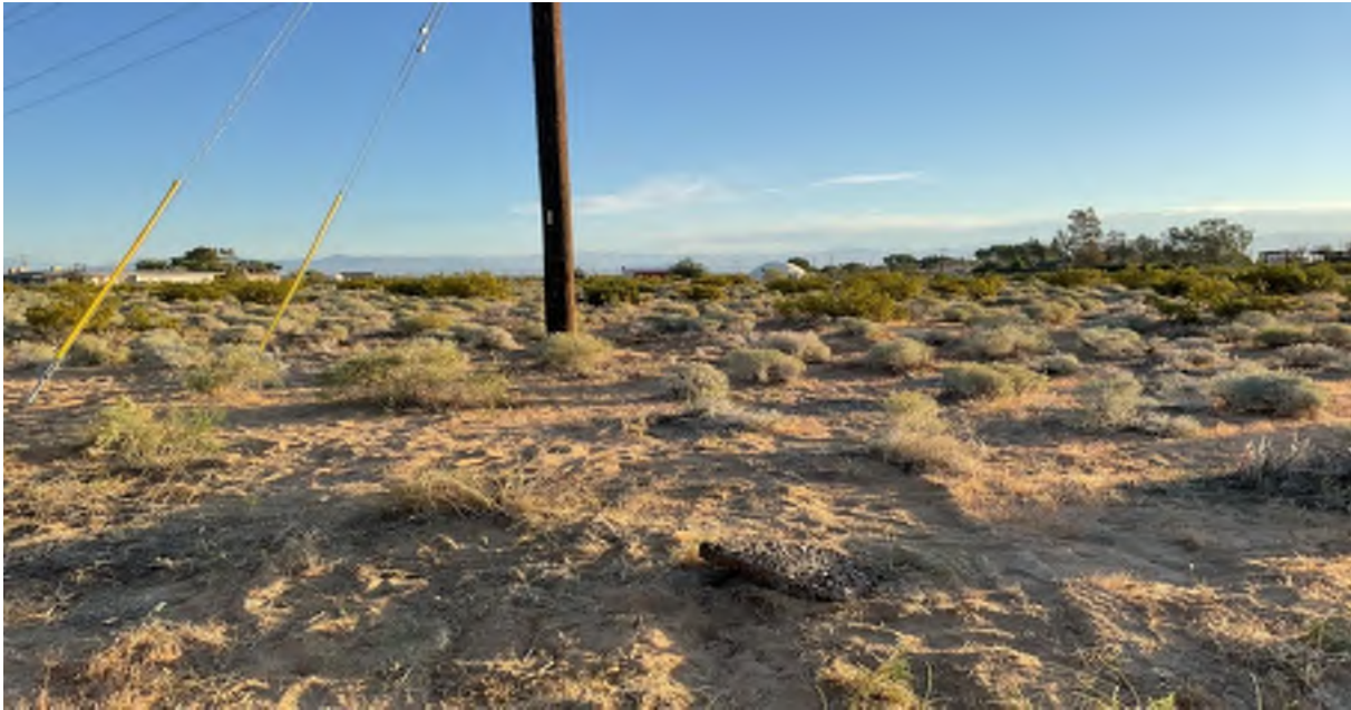
Photo 5. Access road into pole 2025115E after access track was repaired. GPS coordinates 35.654282°N, -117.802255°W, facing northwest. Taken by Danielle Temple on April 24, 2024.
