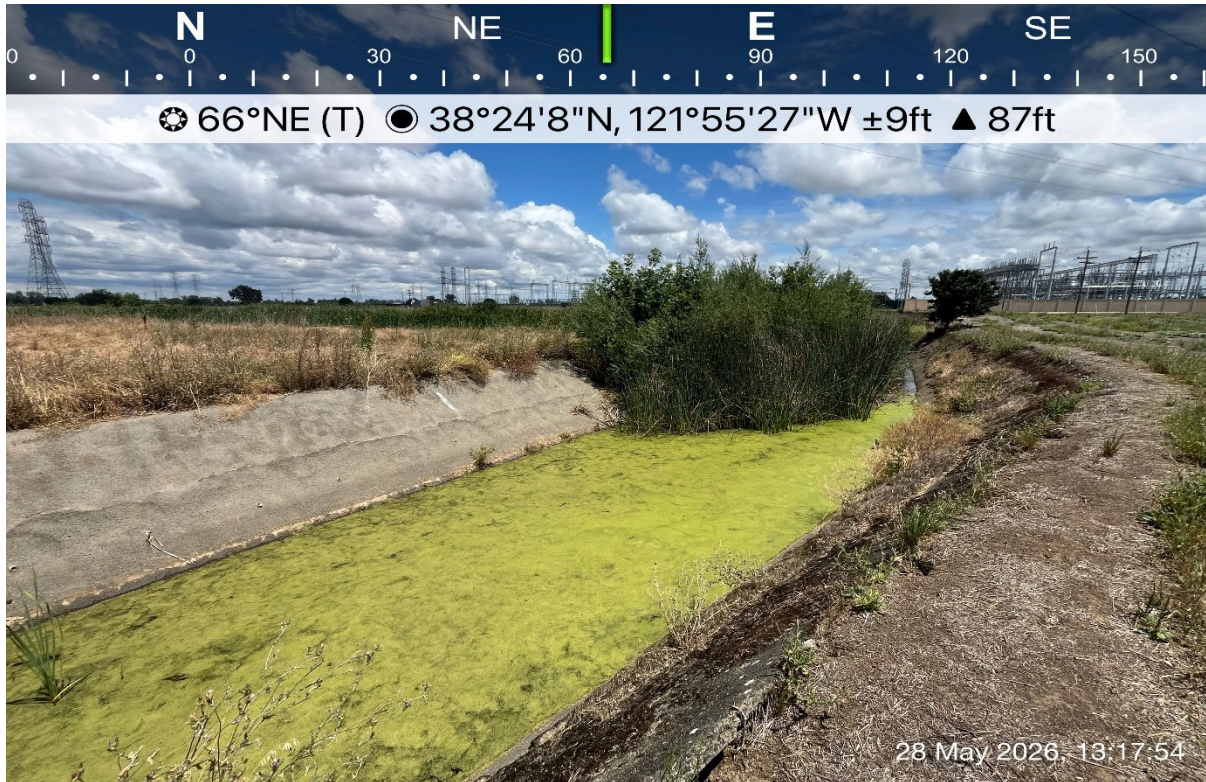
Photograph 7. Concrete channel along southern boundary of subject pond. May 28, 2026.
