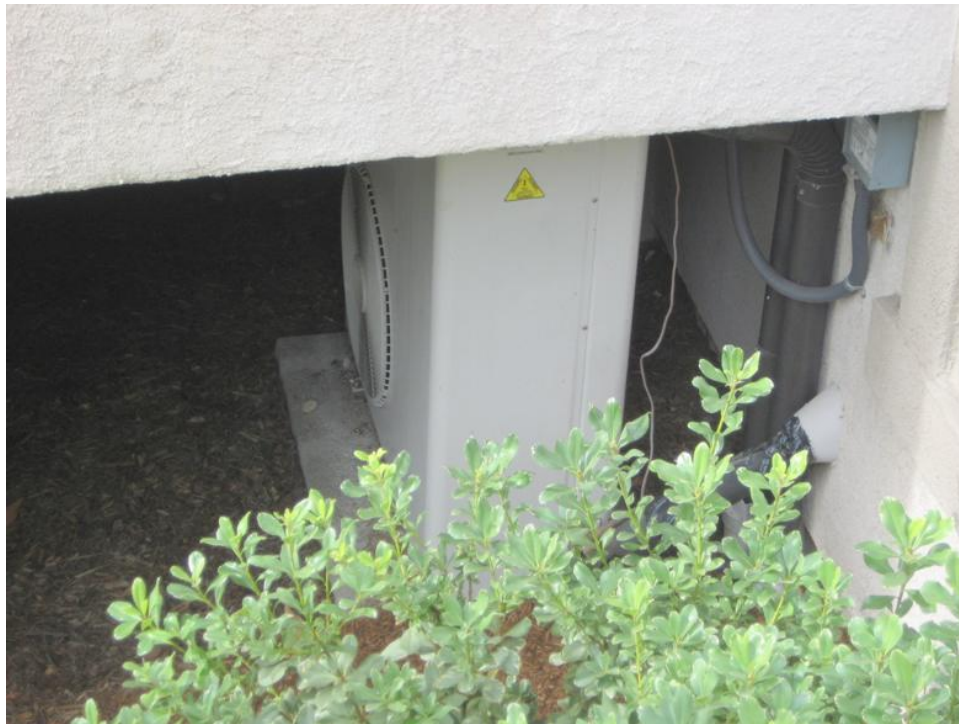
Figure 17: Unit 72—Condenser Recirculation
