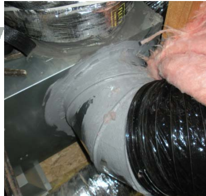
Figure 33: System 10—New Filter Grille Near Existing Grille and New 14 in. dia. Flex Duct Into Furnace Cabinet
