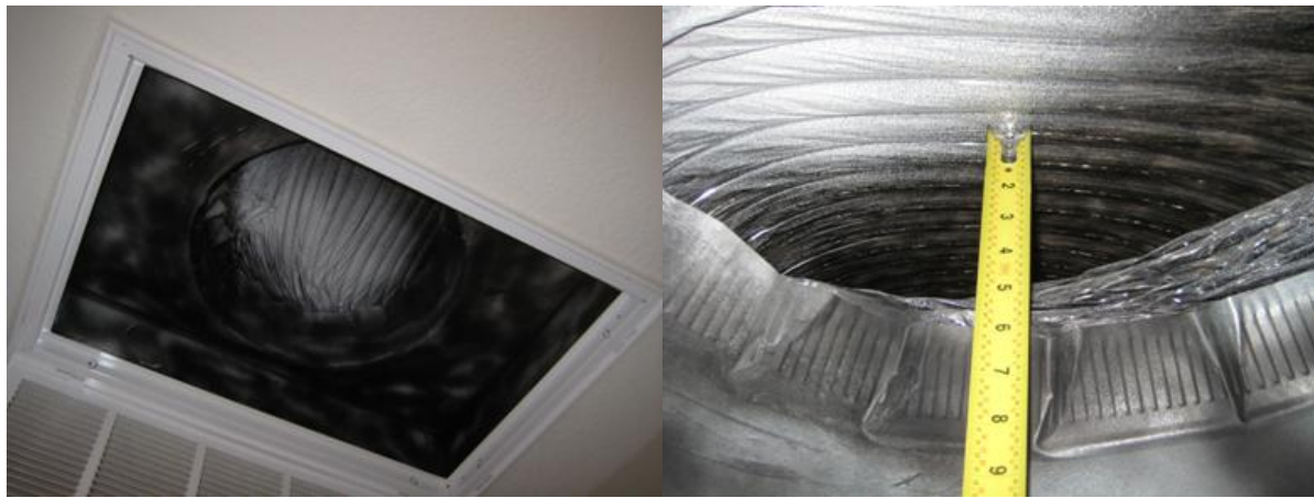
Figure 34: System 17—Existing Return With 5 in. Opening
