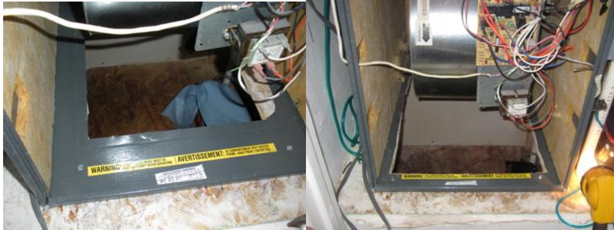
Figure 47: System 74—Furnace Return Opening Before and After Enlargement
