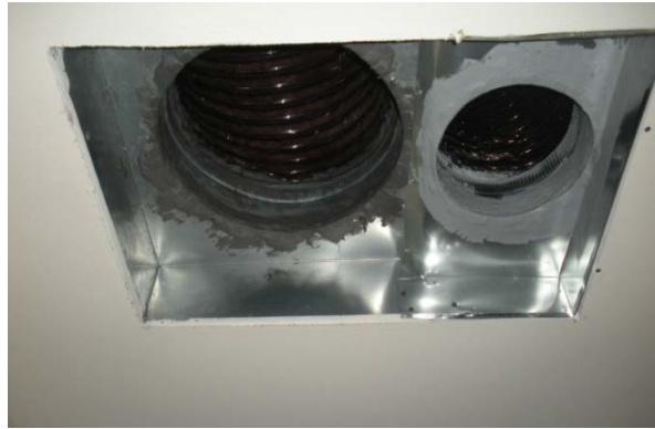
Figure 29: System 4—Original and Revised Return Can With Added 10 in. Return Duct
