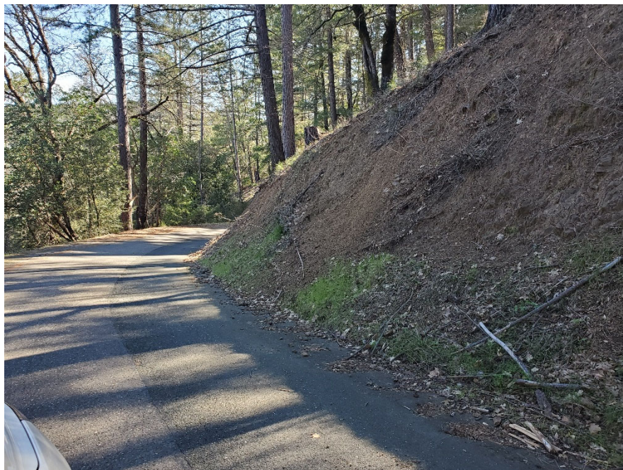
Photo 2 Upper re-seeded section of High Valley Road:
