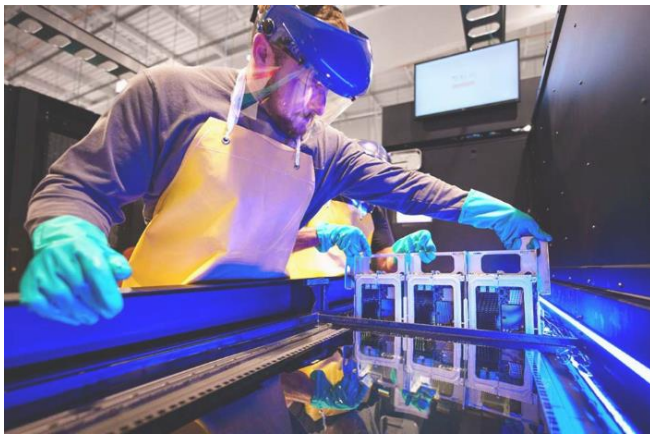
Figure 2: Immersion Cooling at Sandia National Laboratories
