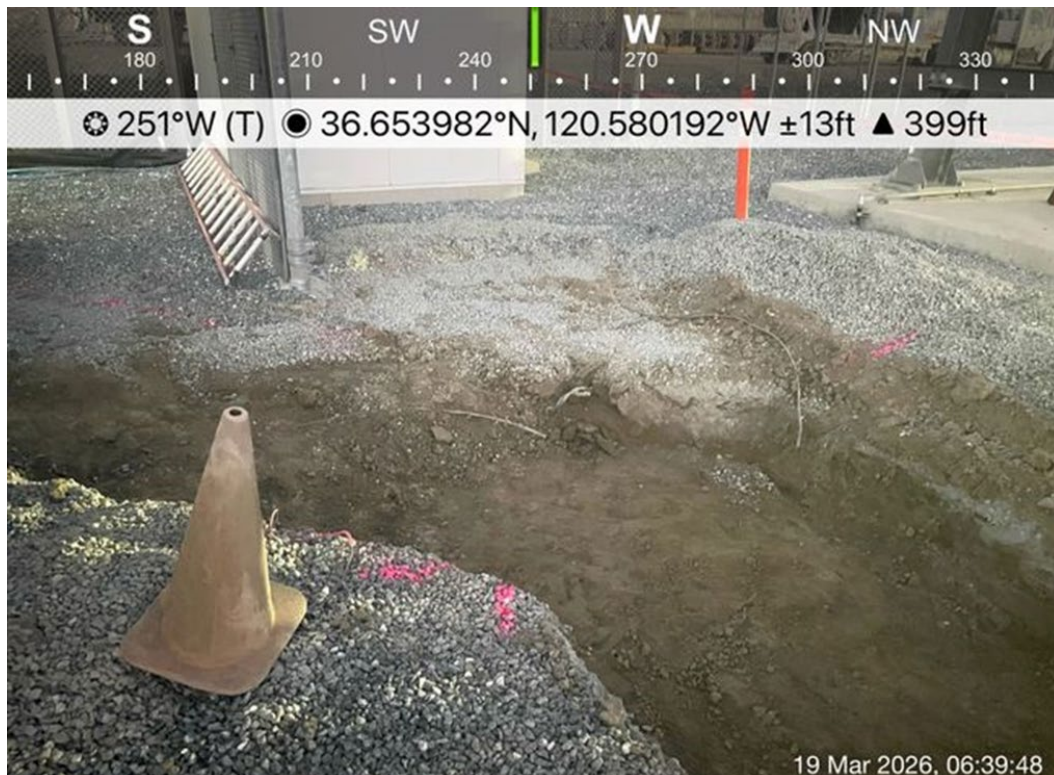
Photograph 3. Overview of Gravel and Previously Disturbed Fill
