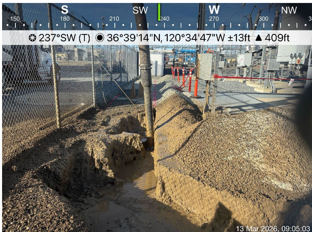
Photograph 4. Disturbed sediment being hydrovaced out of trench within MPP.
