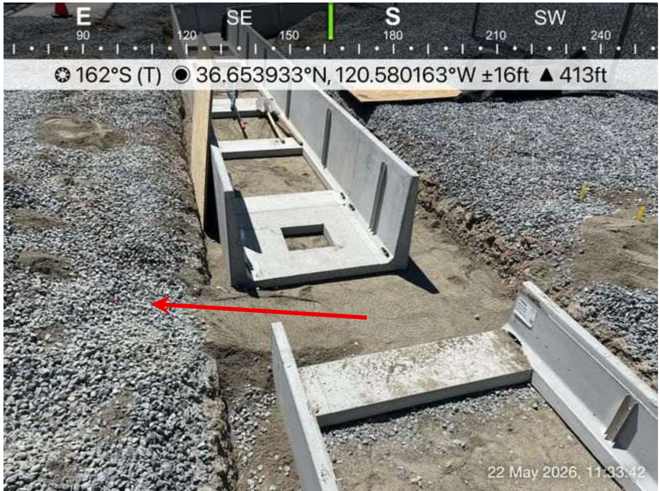
Earthen wildlife escape ramp
