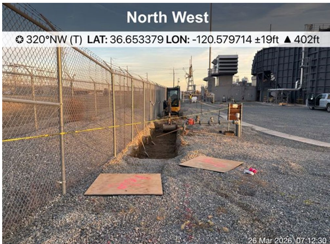
Photograph 4. Overview of Trenching Within Existing MPP Facility
