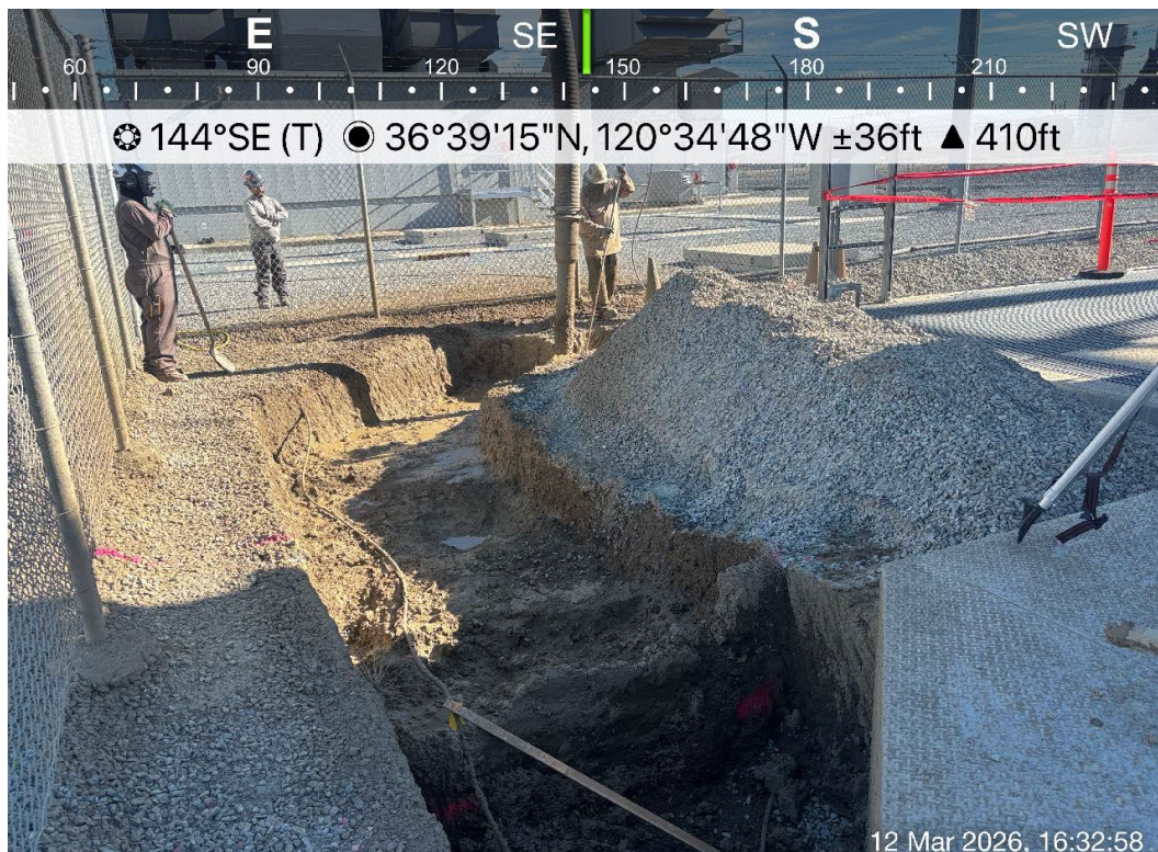
Photograph 2. Excavation within disturbed sediments (gravel and fill dirt) within MPP.
