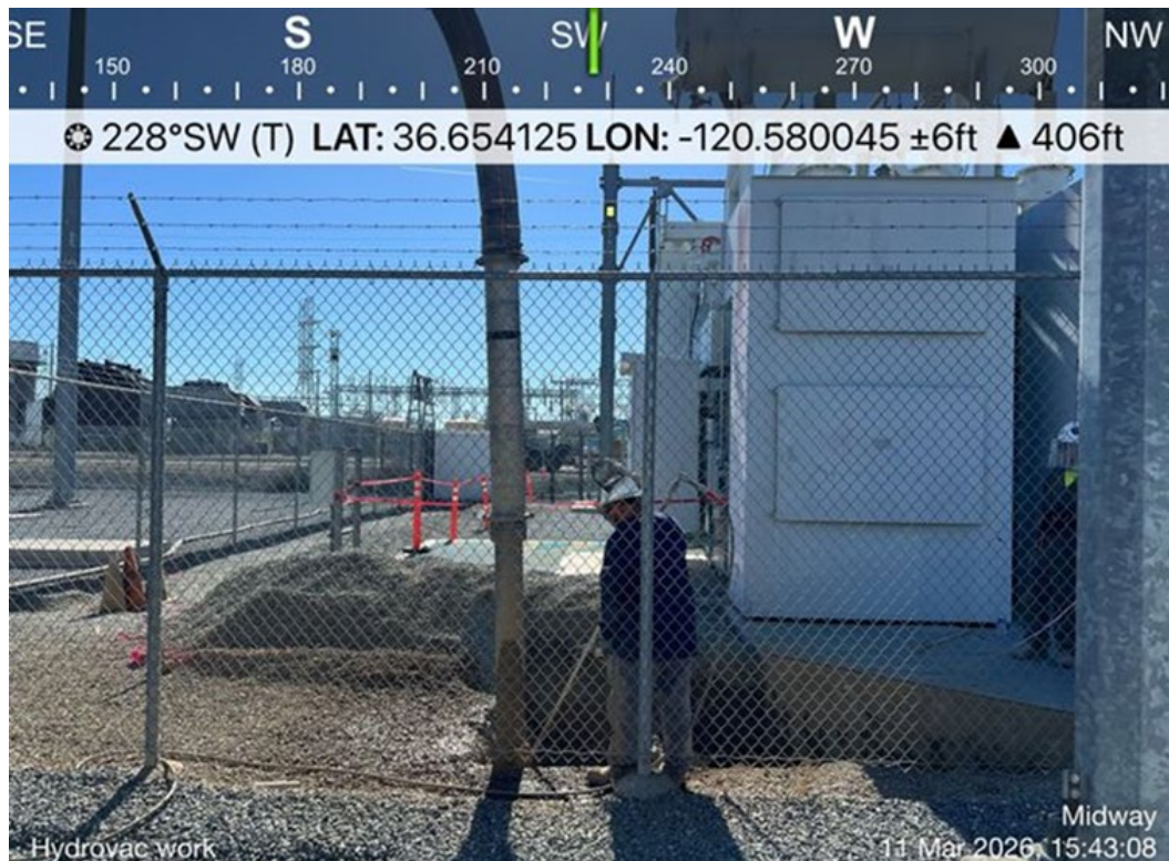
Photograph 1. Excavation in Disturbed Fill Below Existing MPP Facility
