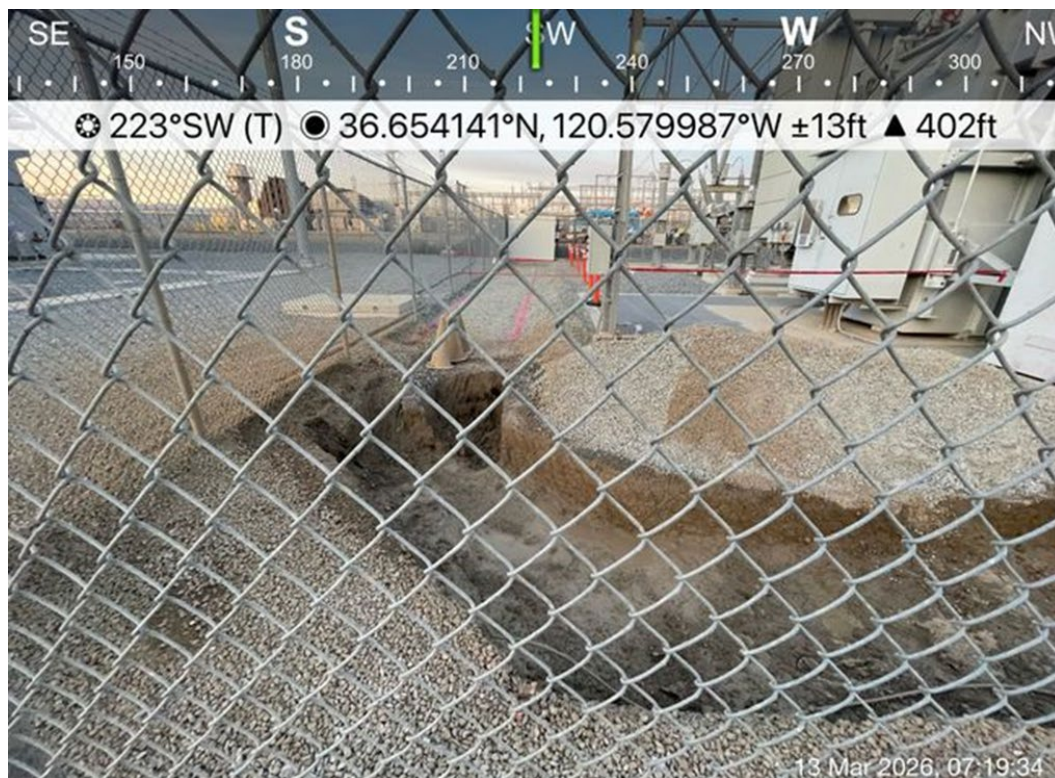
Photograph 2. Overview: Excavation in Previously Disturbed Fill within Existing MPP Facility
