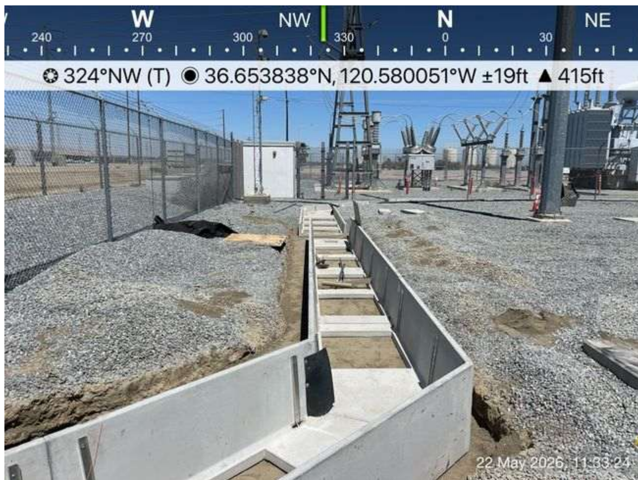
End of day concrete run progress
