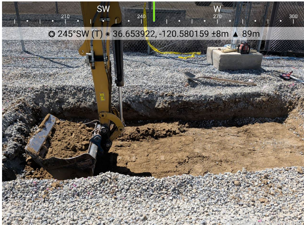
Photograph 1. Excavation within disturbed sediments (gravel and fill dirt) within MPP.
