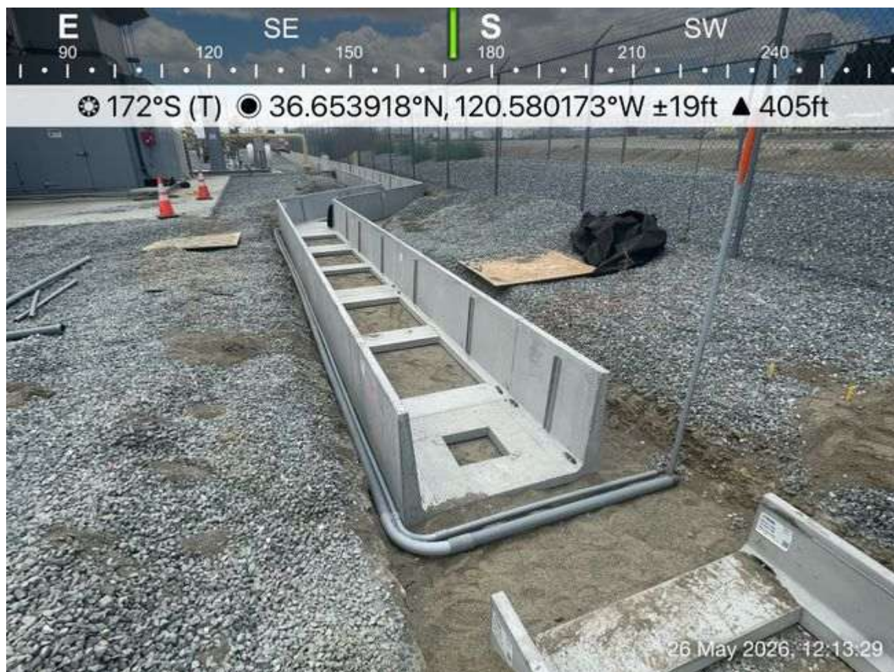
Conduit installed along concrete runs.
