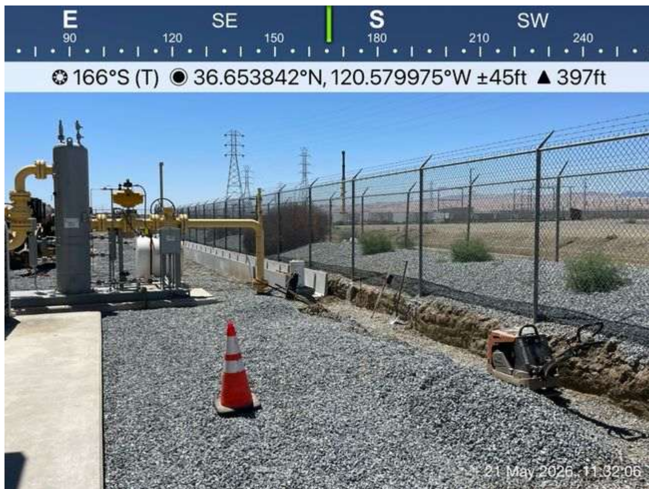
Compaction of ground within the trench
