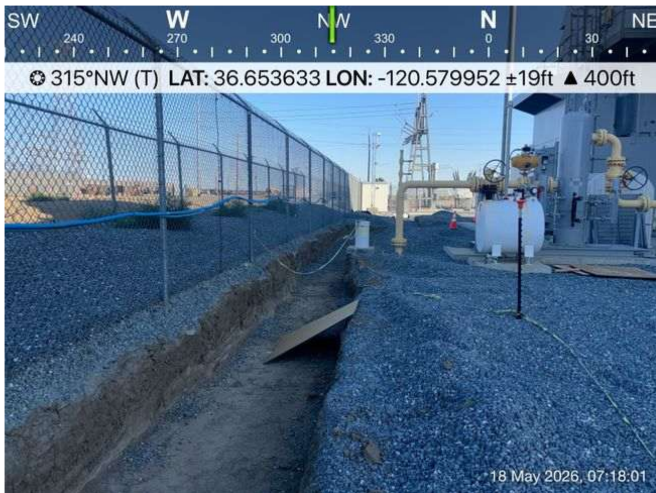
View of trench with wildlife escape ramp.
