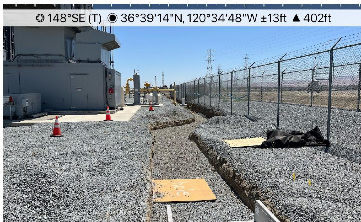
Overview of gen-tie work area.
