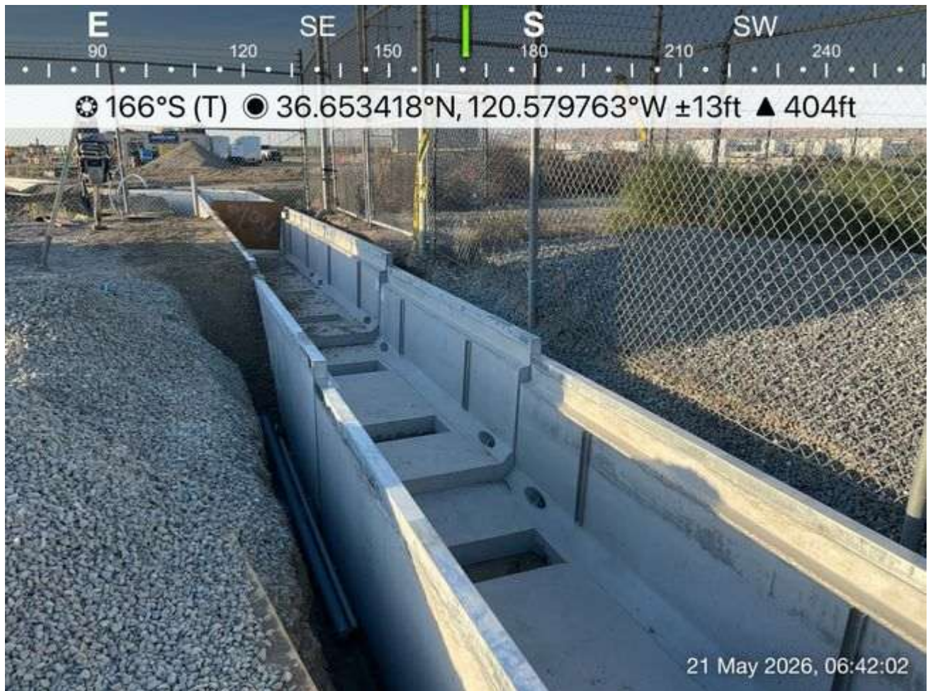
Morning trench check
