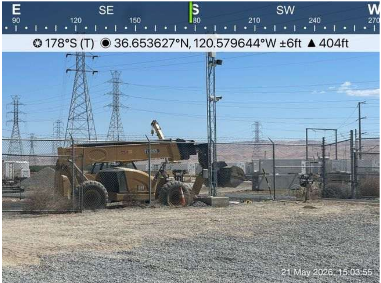
Back filling along edges of the concrete runs begins
