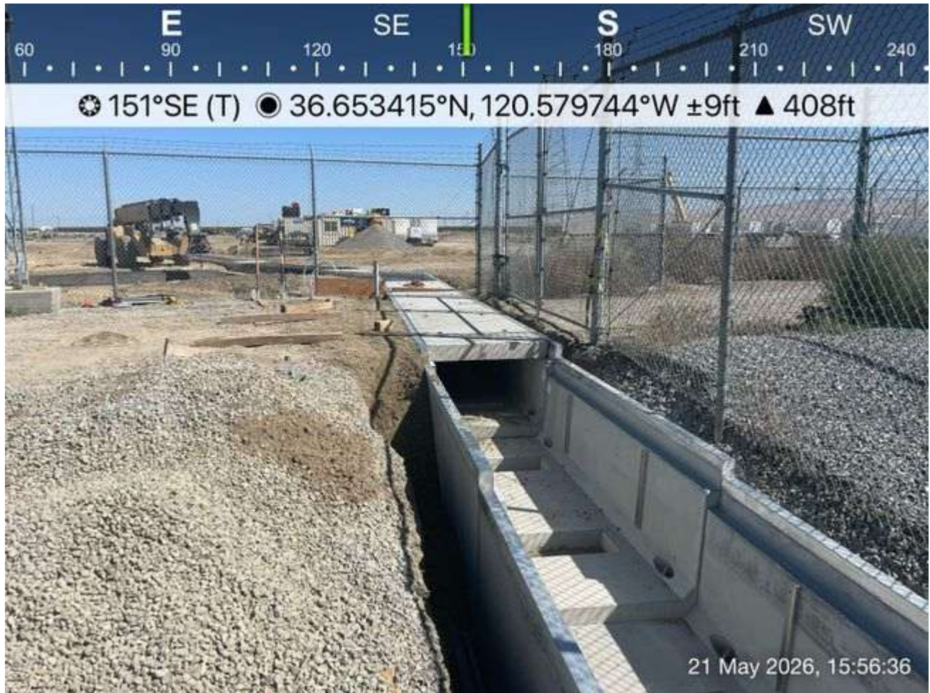
Covers placed on the concrete run
