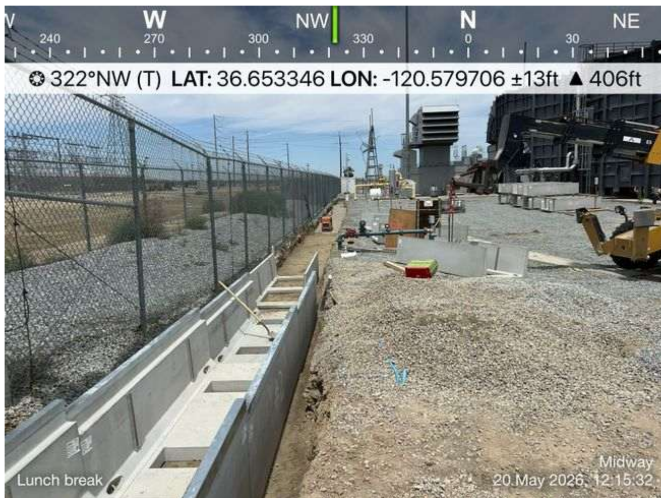
Crew on lunch break. Progress photo.
