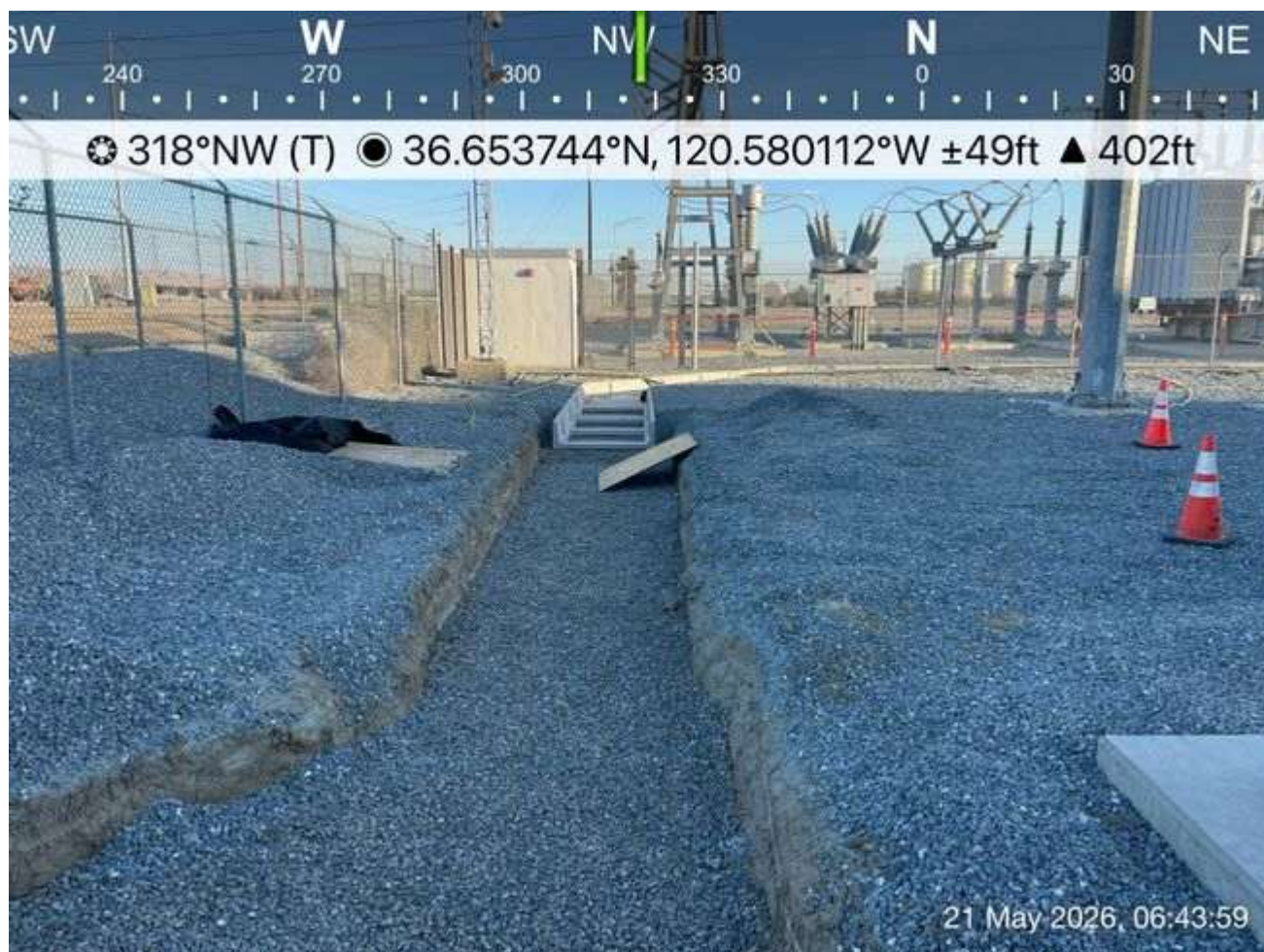
Wildlife escape ramp placed in trench
