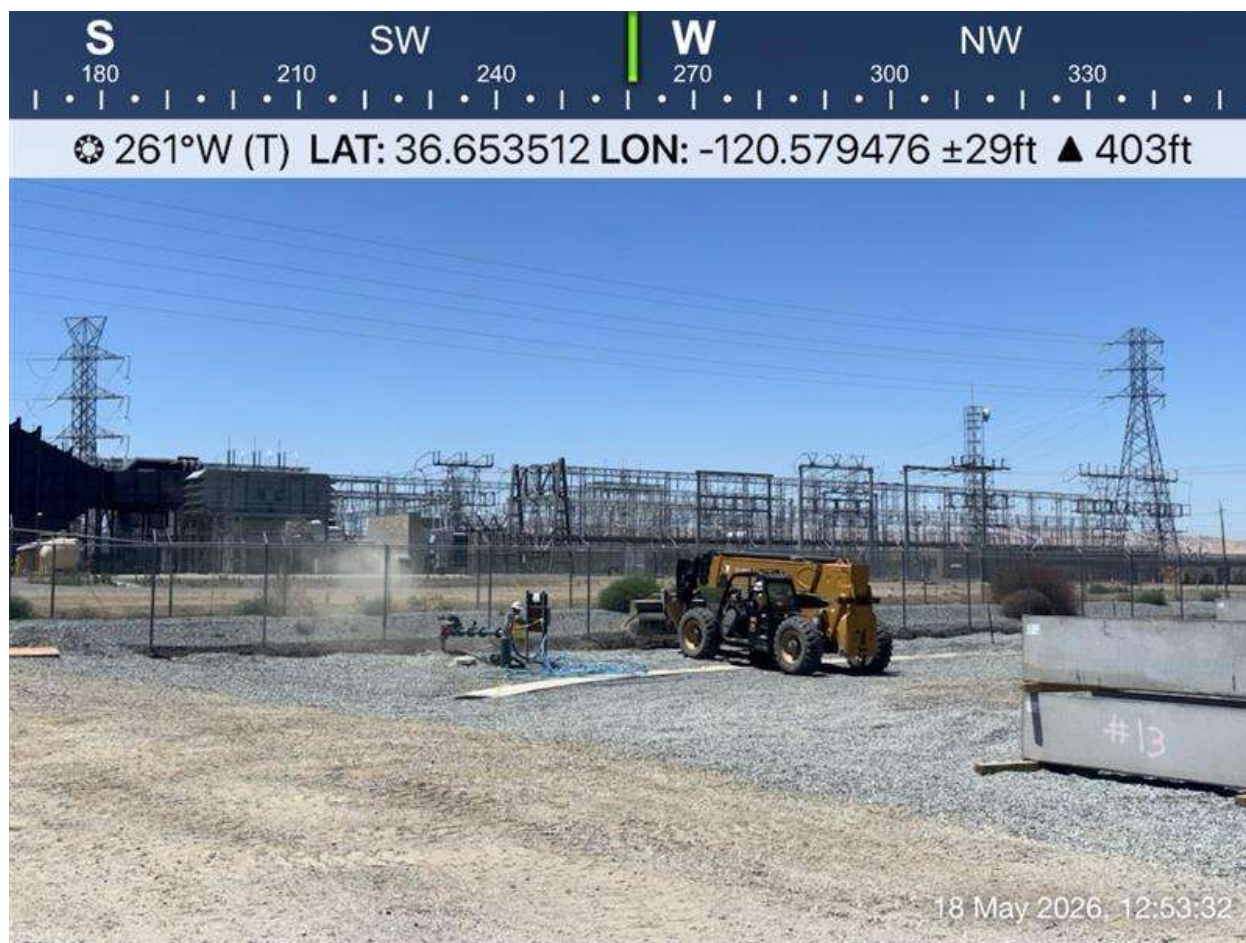
View of the crew adding gravel to the trench.
