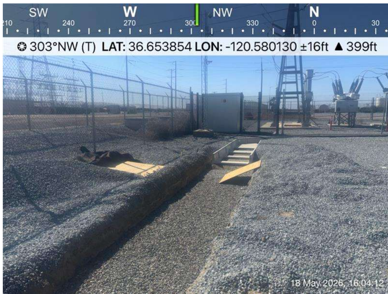
View of the ramps added to the trench at the end of the day.
