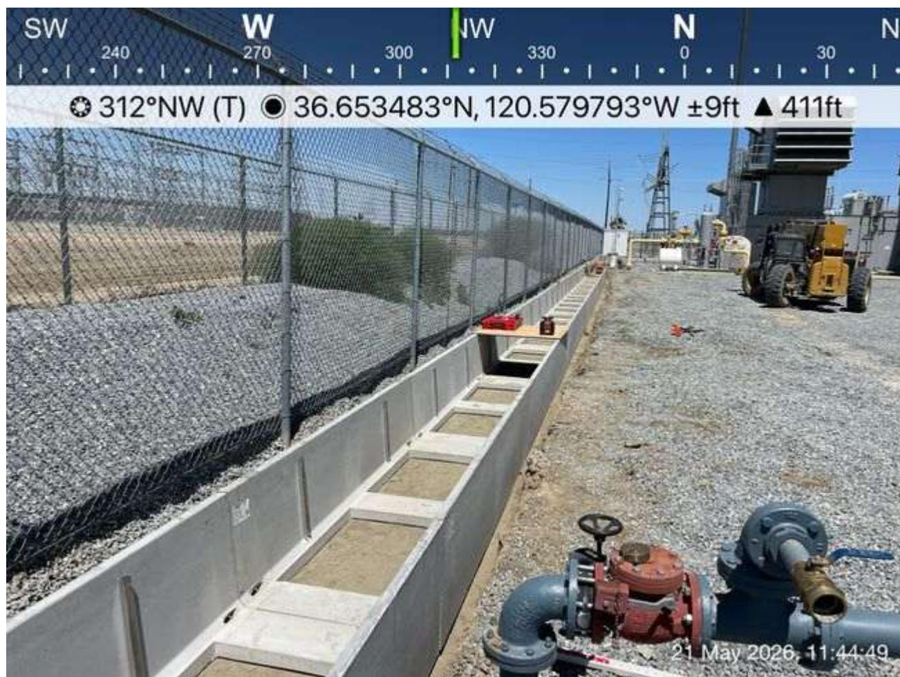
Midday progress of trench lining
