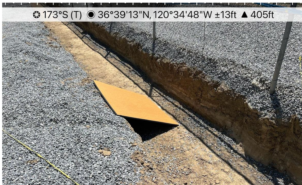
Escape ramp installed within trench.
