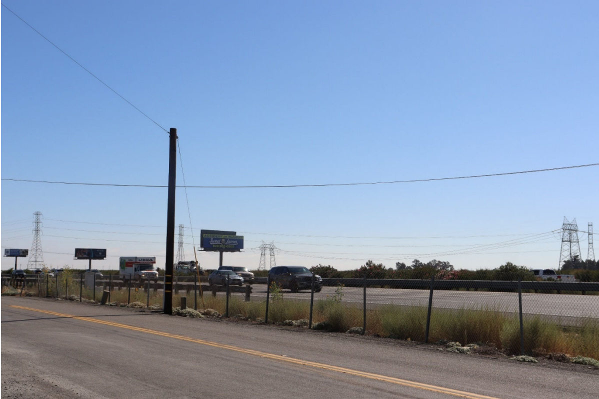
View 3: Existing view looking southeast along Quinn Road with I-80 in the foreground. The BESS Project Area is located on the far (south) side of I-80, and is obscured by vegetation. This image shows the existing transmission infrastructure surrounding and crossing over I-80 and proximate local roadways.
