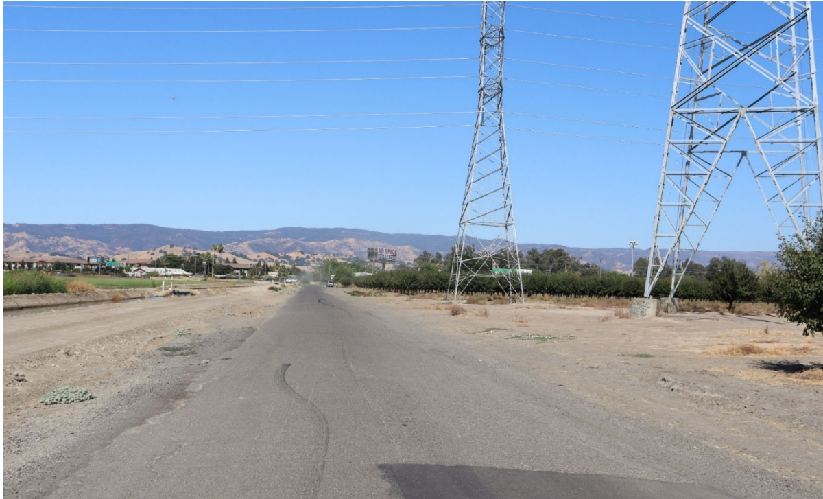
View 1: Existing view looking west along Kilkenny Road. The Project Site and existing transmission infrastructure are visible on the right-hand side of the foreground with distant views of the Vaca Mountains in the background.
