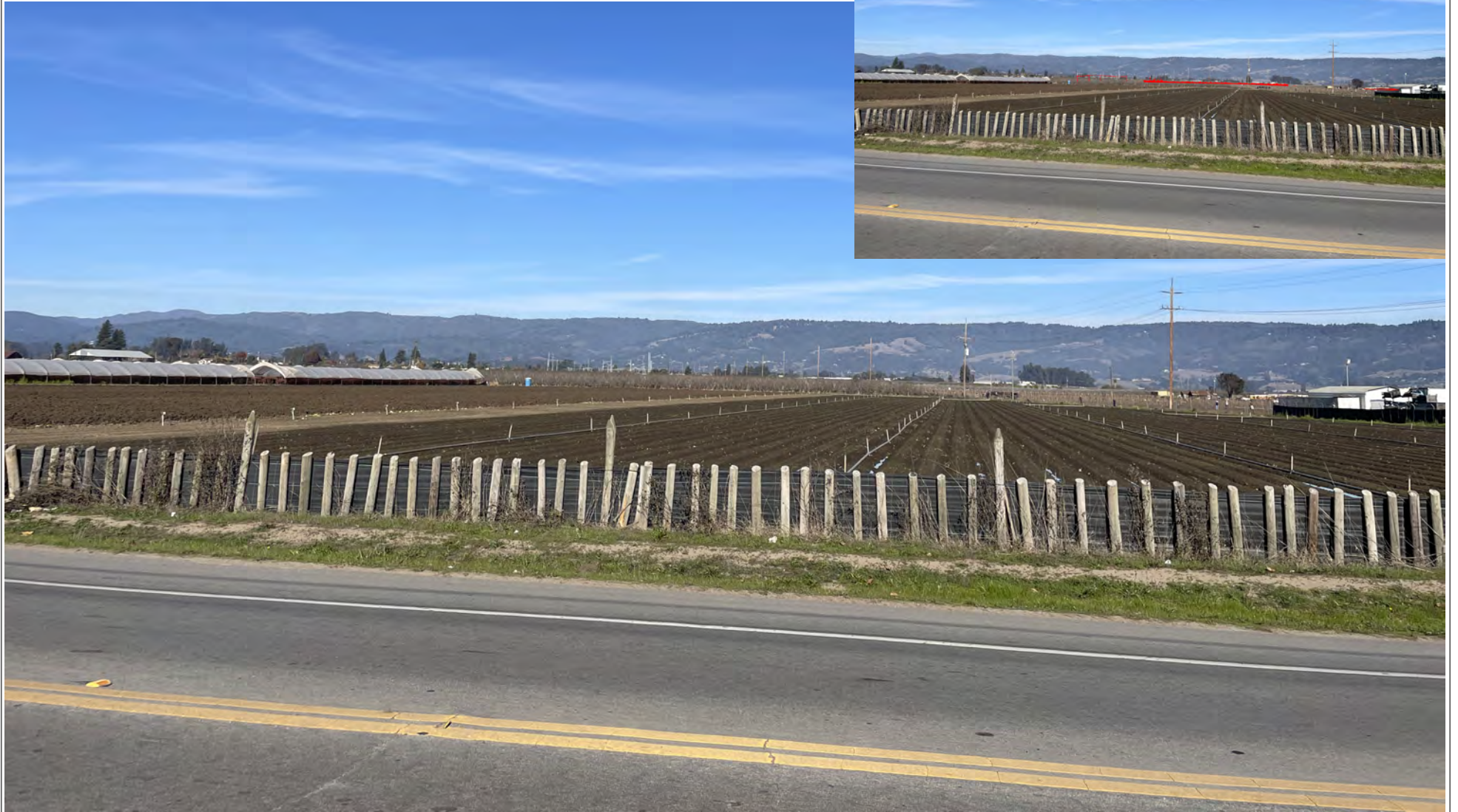
Visual Simulation of the Project (components obscured by distance and presence of existing substation facility)
