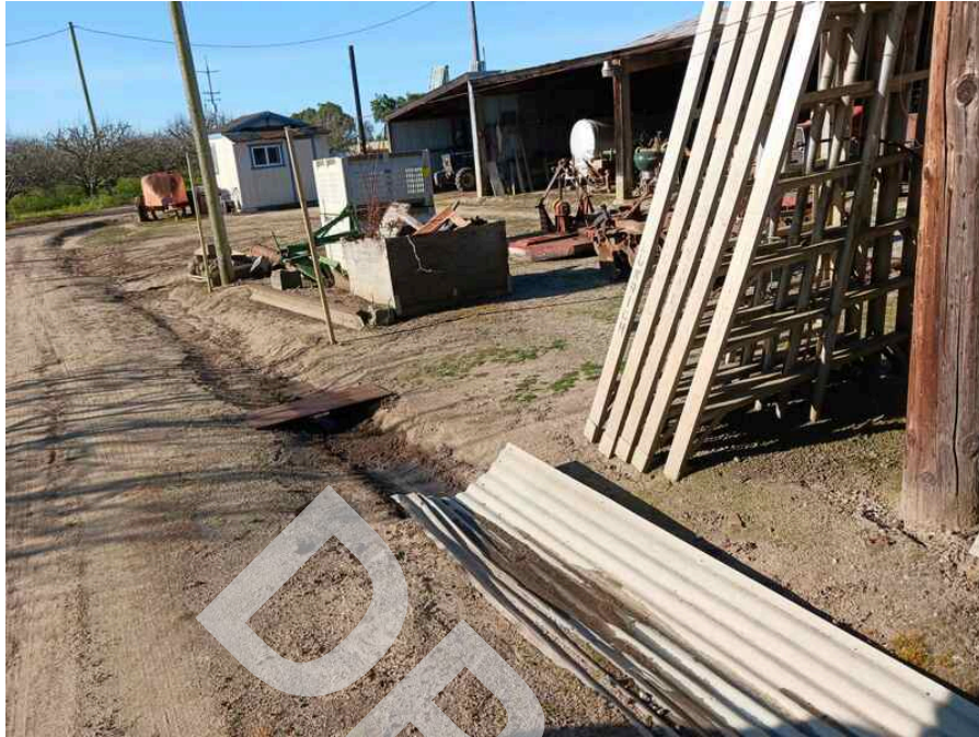
31. Trench area associated with the "gray water" drainage system.
