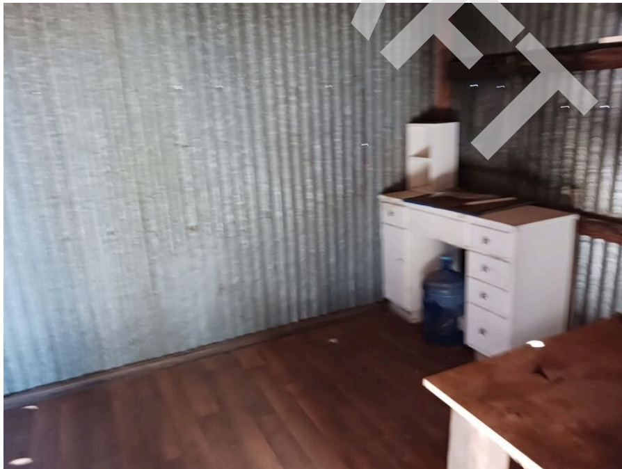
18. Overview of the office space interior.
