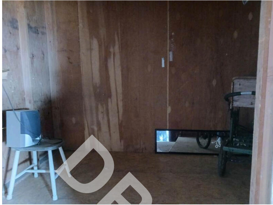
19. Overview of the office space interior.
