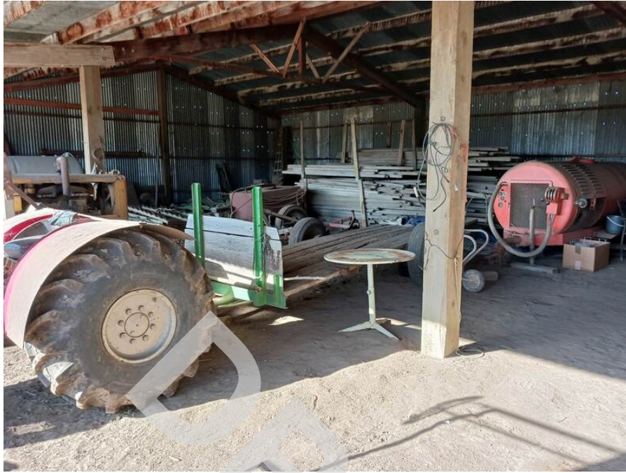
15. Open equipment storage area associated with the barn structure.
