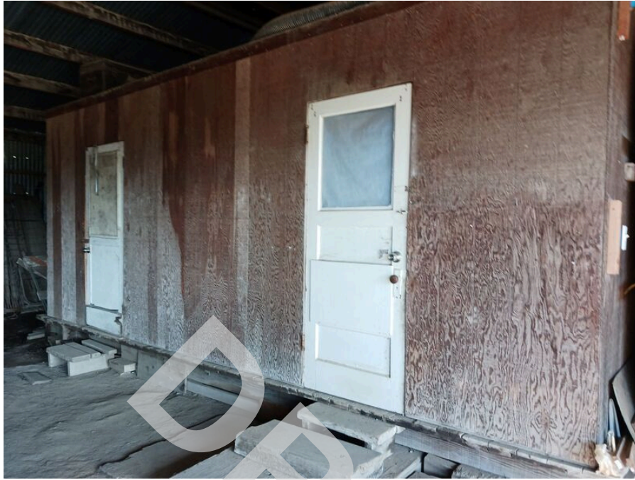
17. Office space observed within the open equipment storage area.
