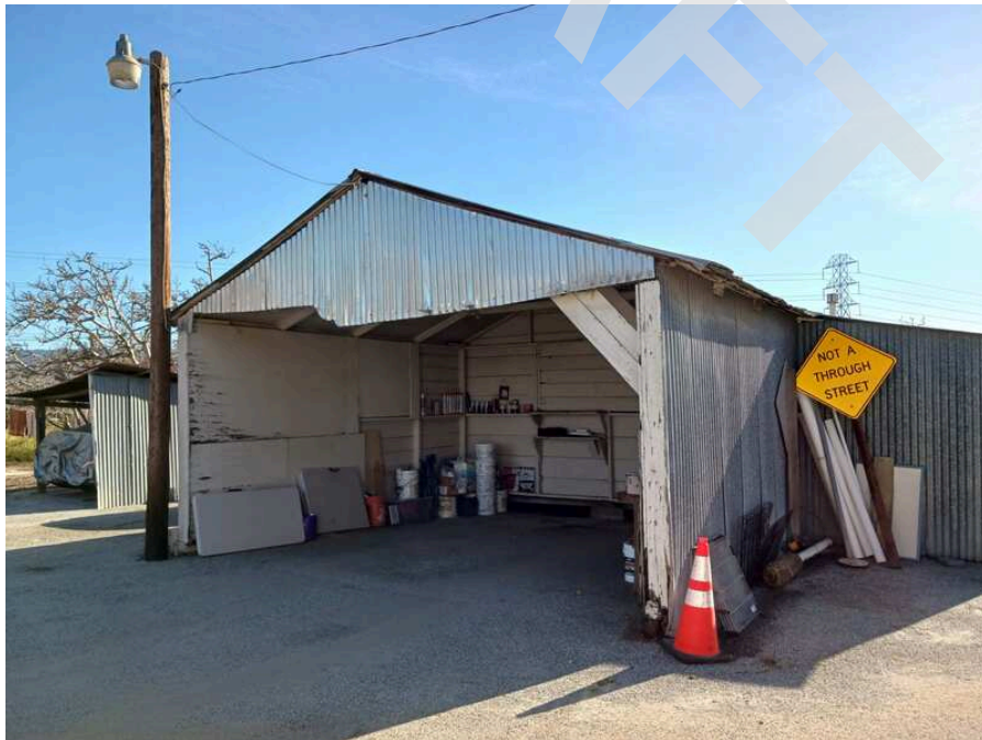
4. Overview of the garage structure.
