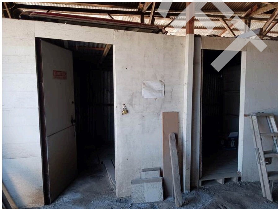
26. Storage rooms observed within the barn structure.
