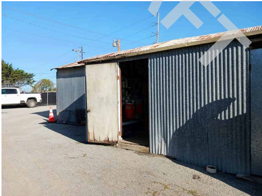
6. Storage rooms attached to the garage structure.
