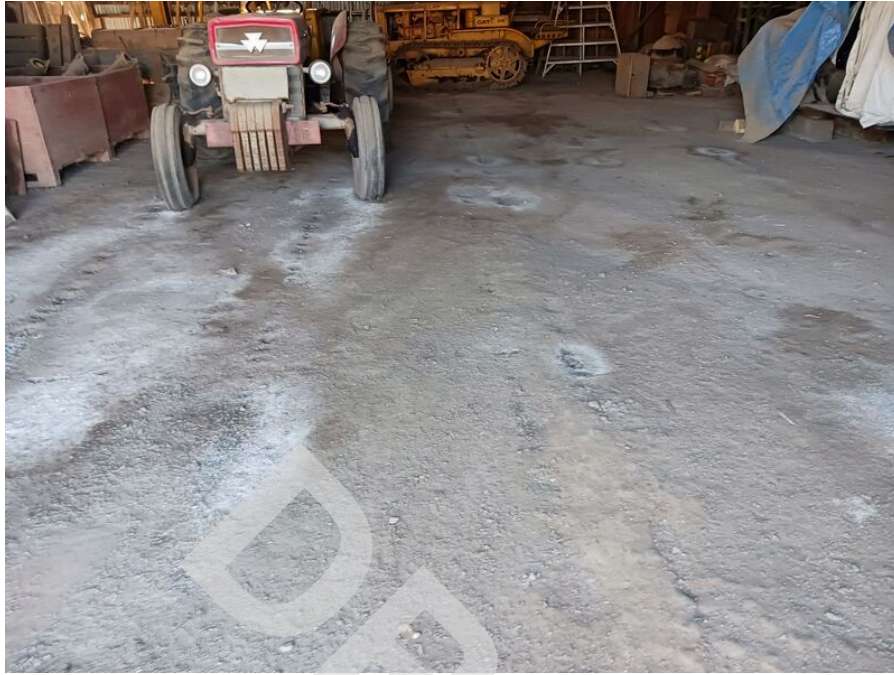
21. Interior of the barn structure.
