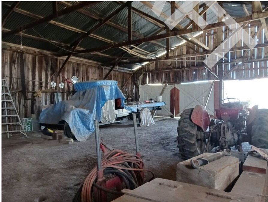
24. Interior of the barn structure.
