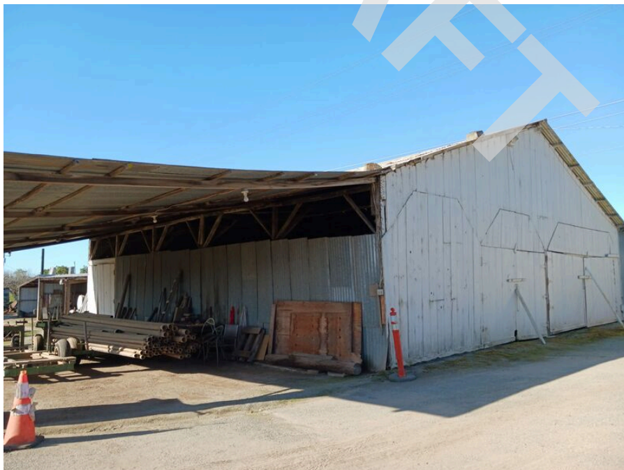
14. Exterior of the barn structure.
