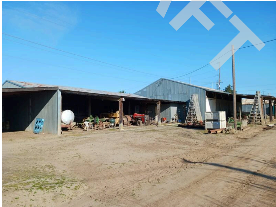
20. Overview of the area occupied by the barn structure.
