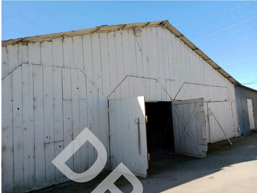
13. Exterior of the barn structure.
