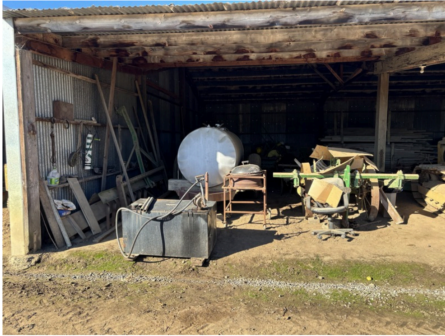
27. 100 gallon diesel AST, southern interior of barn
