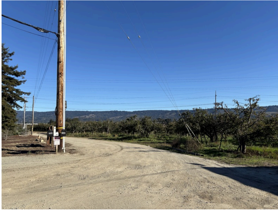
1. View Northeast of Minto Road and Subject Property
