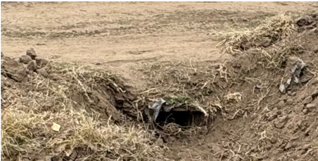
FIGURE 4: EXISTING 15-INCH CMP CULVERT
