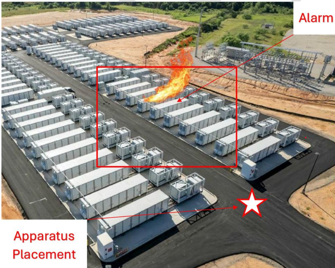
Figure 27 Safe Staging for Asset Protection
