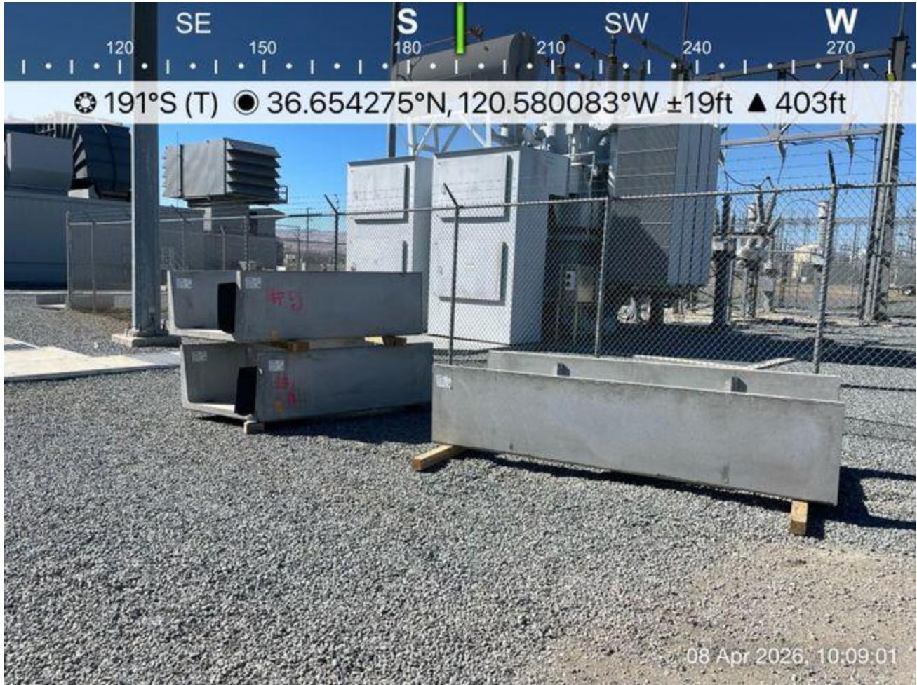
Materials staged onsite
