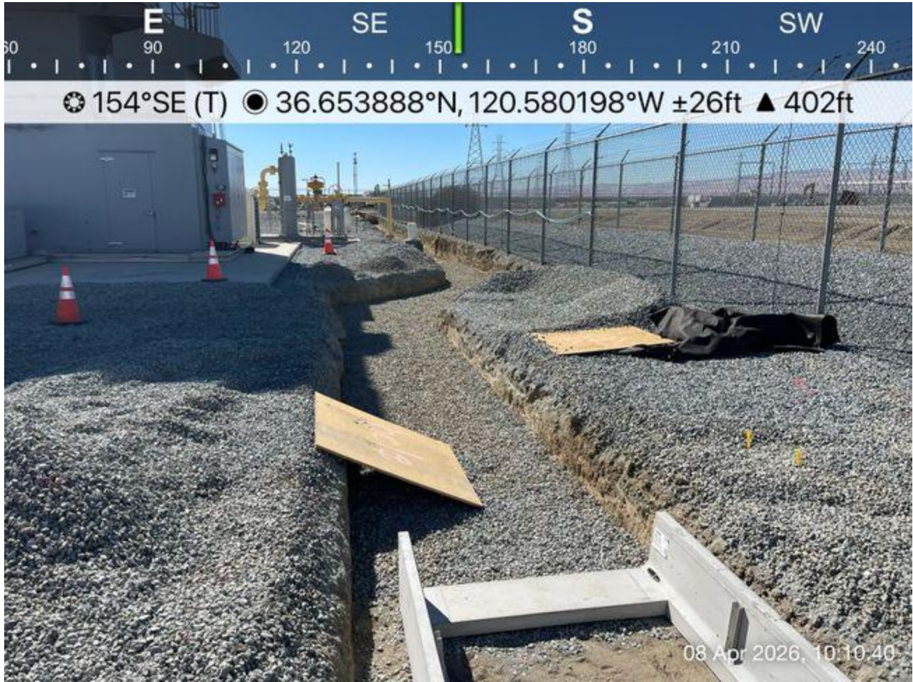
Escape ramps placed in the open trench
