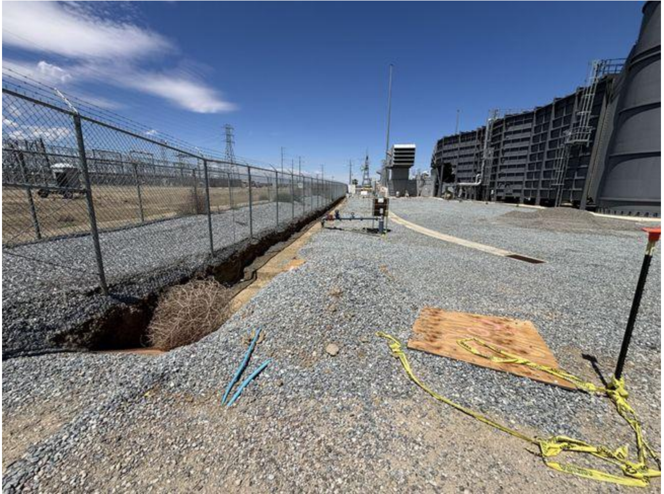
Trench with adequate ramp and covered holes. Tumble weed was removed.
