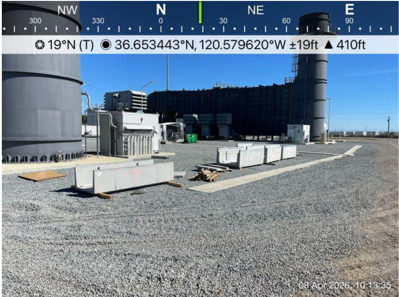
More staged work materials
