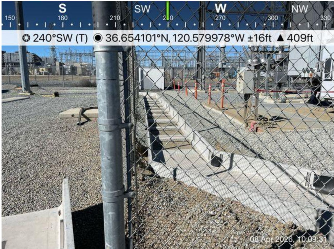
Overview of work area within the fence of the transformer
