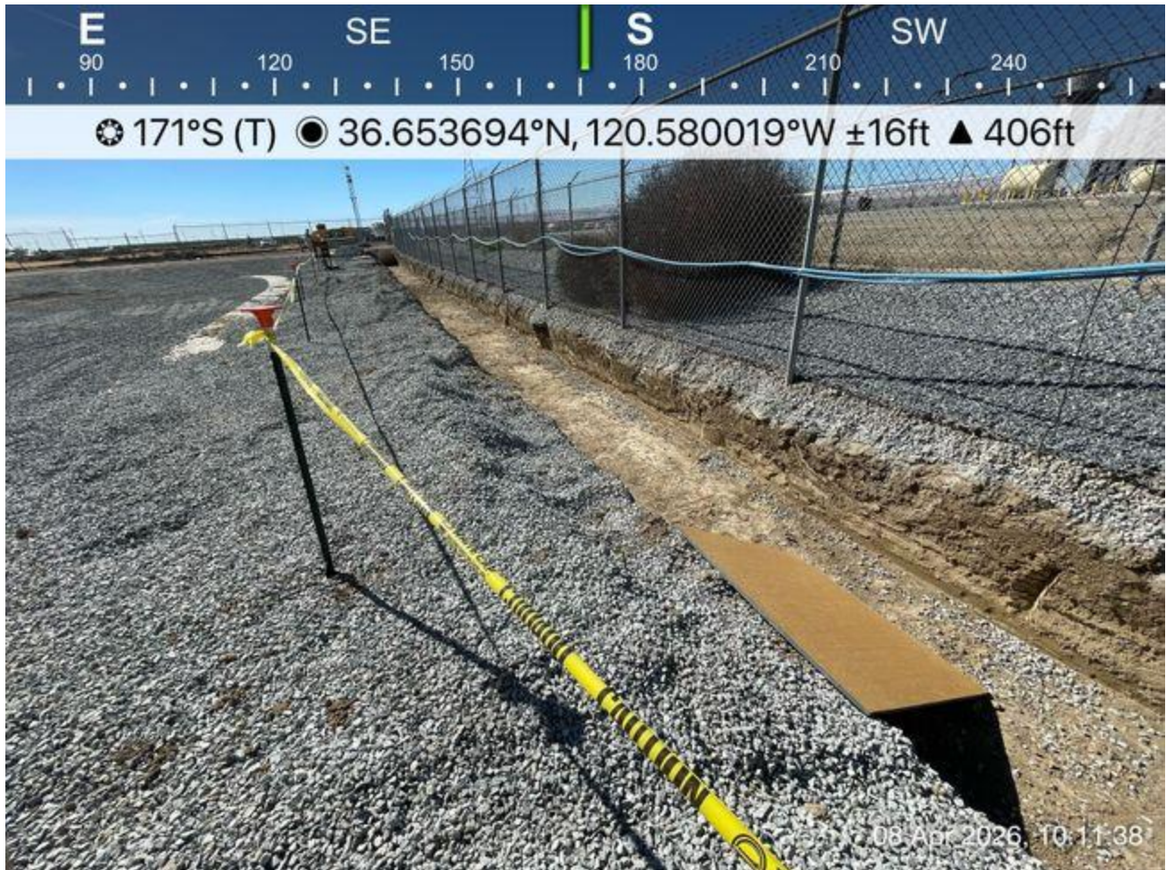
Overview of open trench
