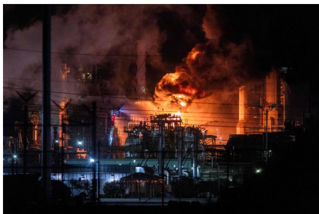
Figure 14. Fire at Chevron Refinery Outside of Los Angeles 97
