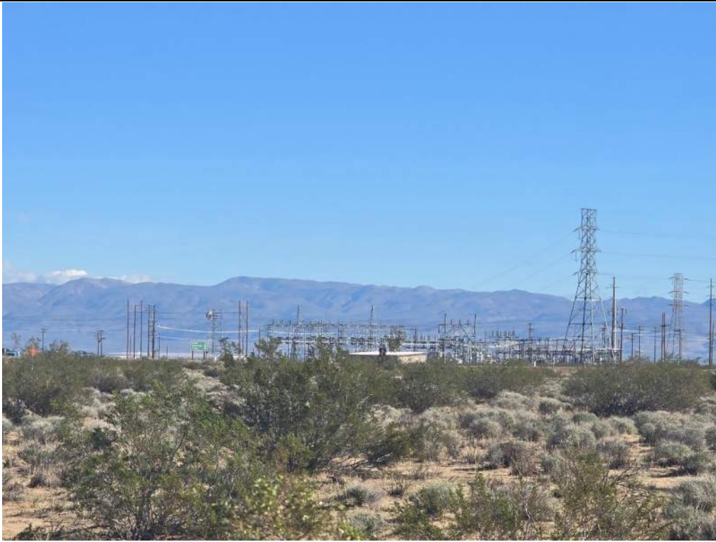
Photo 33: View of electric substation approximately 0.35-miles northeast from near the southeastern corner of the eastern portion of the Subject Property.
