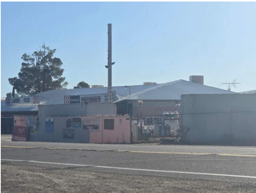
Photo 6: View of hardware store and multiple propane tanks on adjacent property to the south of the Subject Property across CA-178.
