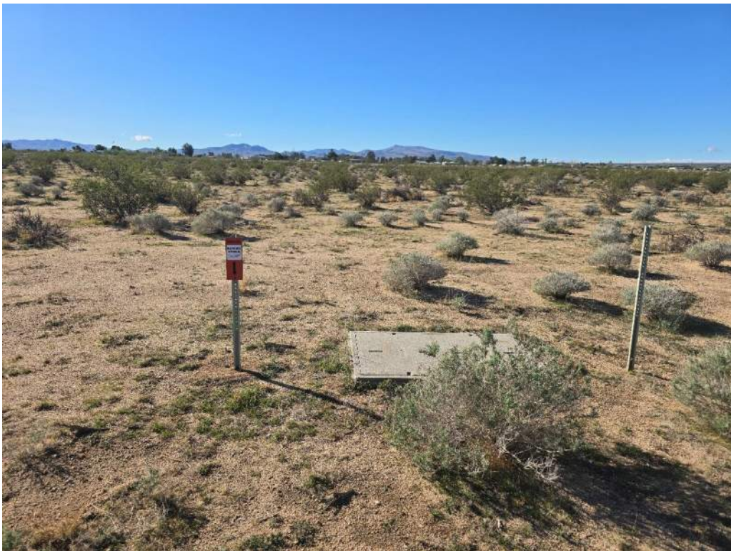
Photo 30: View of buried cable in narrow segment between eastern and western portions of Subject Property facing south from near Nadine St.
