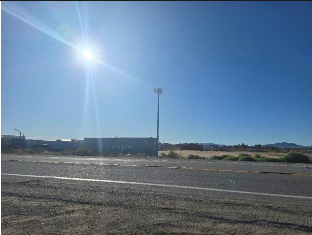
Photo 5: View of cell tower on adjacent property facing south from near the southwestern corner.
