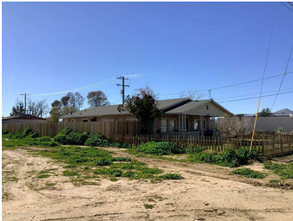
Photo 2. Primary and west facades, view toward southeast.
