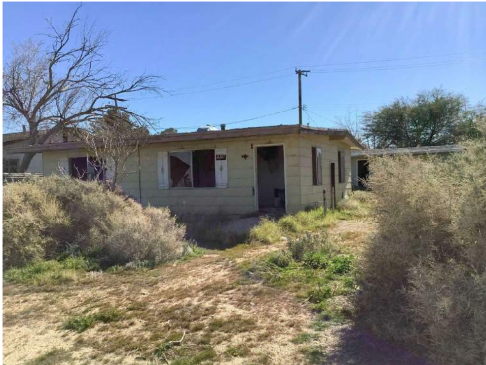
Photo 2. East facade, view toward southwest.
