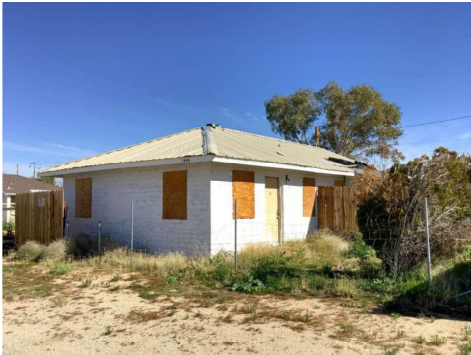
Photo 8.: Building Three: View toward northeast.
