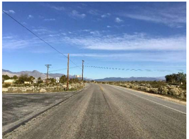
Image 4. Segment 1, view of Old Highway 396.
