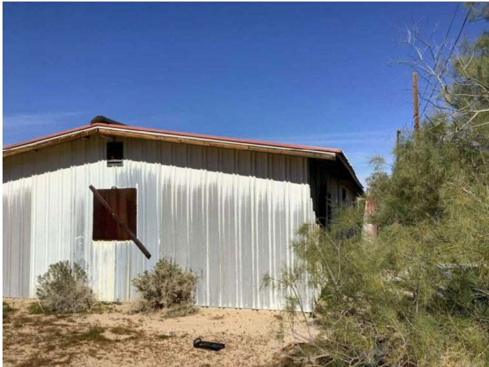
Photo 2. Side façade, view toward north.
