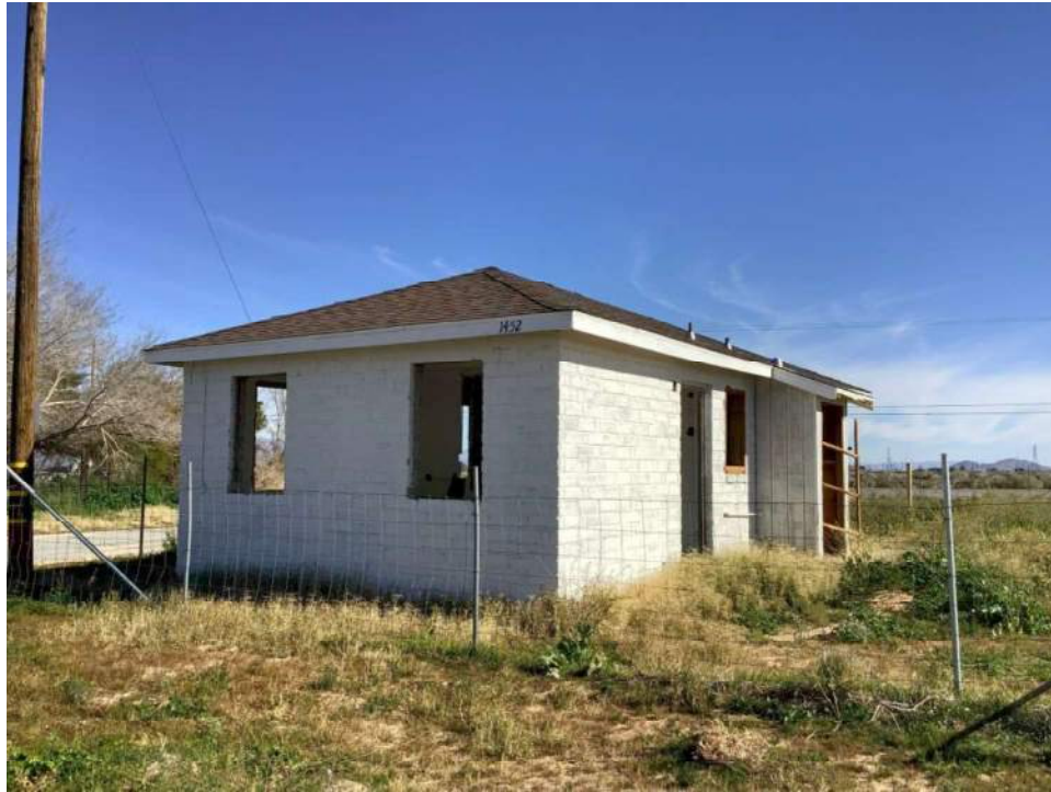
Photo 5.: Building Two: rear and side façades, view toward northwest.
