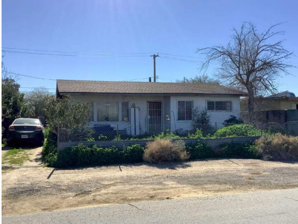
Photo 1. North facade, view toward south.
