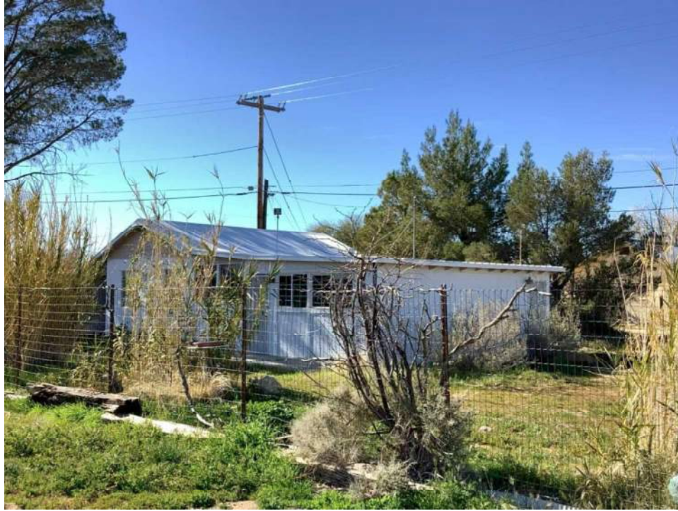
Photo 3. Rear and side façade, view toward southwest.
