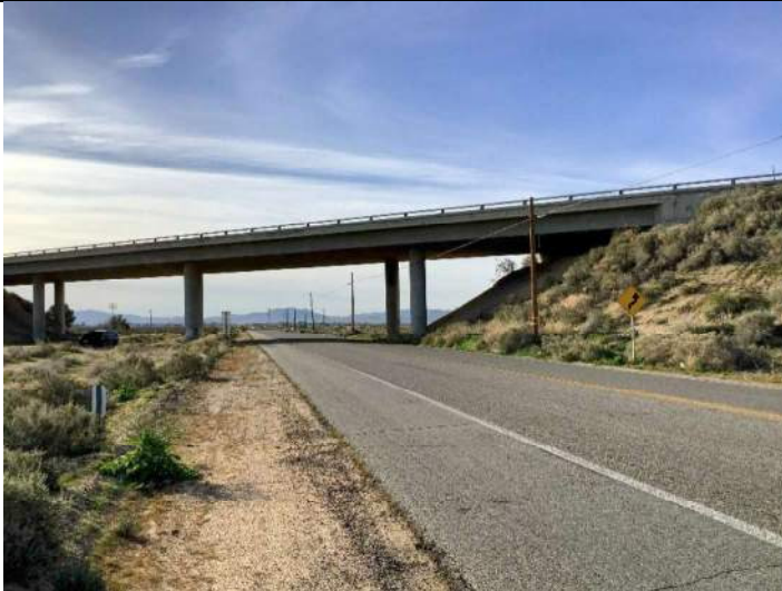
Image 3. Segment 1, view of Highway 395 overpass of Brown Road, old Highway 395.
