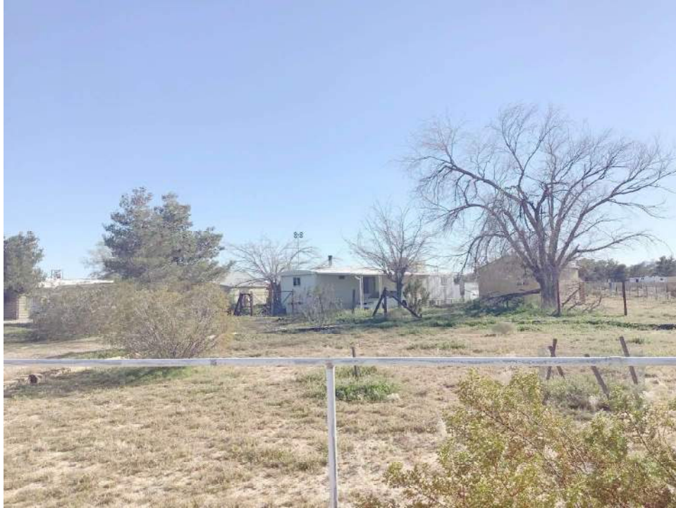
Photo 1. North and east facades, view toward southwest.
