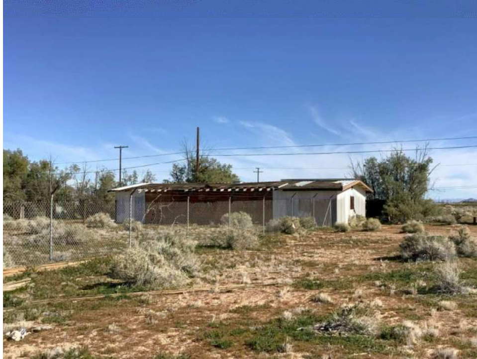
Photo 1. Primary and side façades, view toward northeast.
