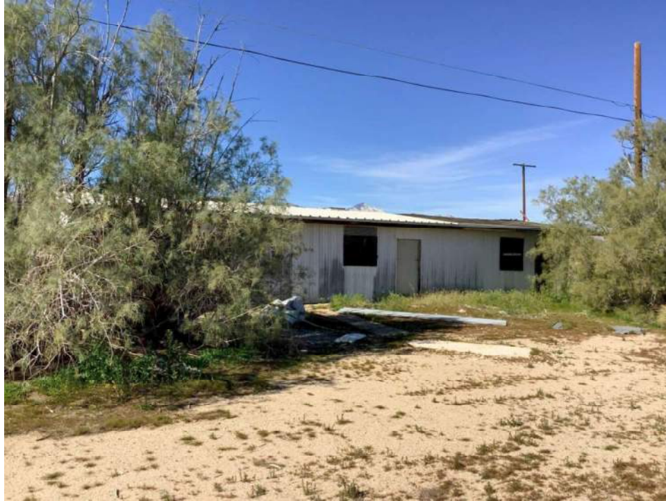
Photo 3. Rear façade, view toward northwest.
