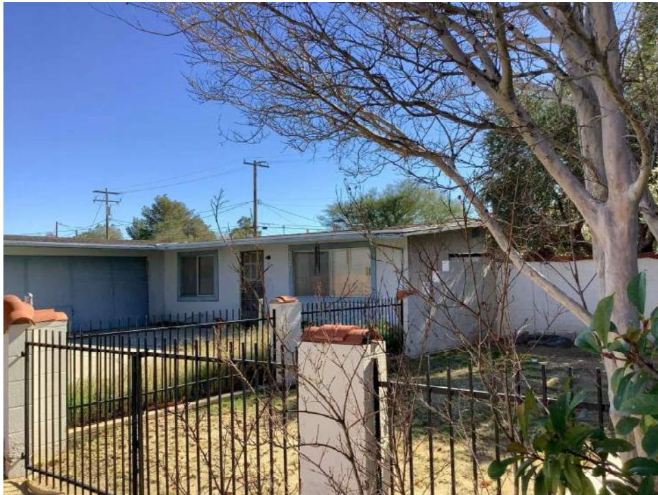
Photo 2. East facade, view toward southwest.
