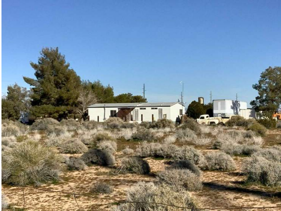
Photo 1. East and south facades, view toward northwest.
