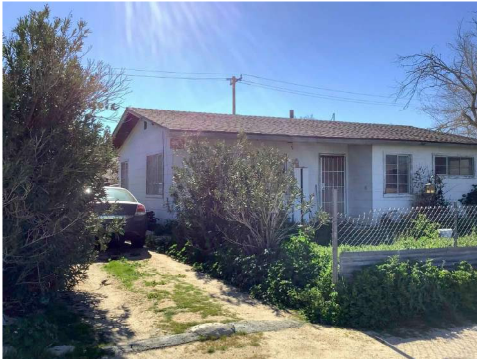
Photo 2. North and west facade, view toward southeast.
