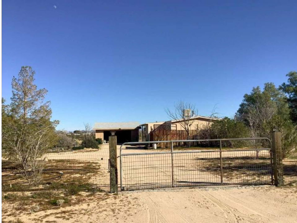
Photo 1. East facades, view toward west.
