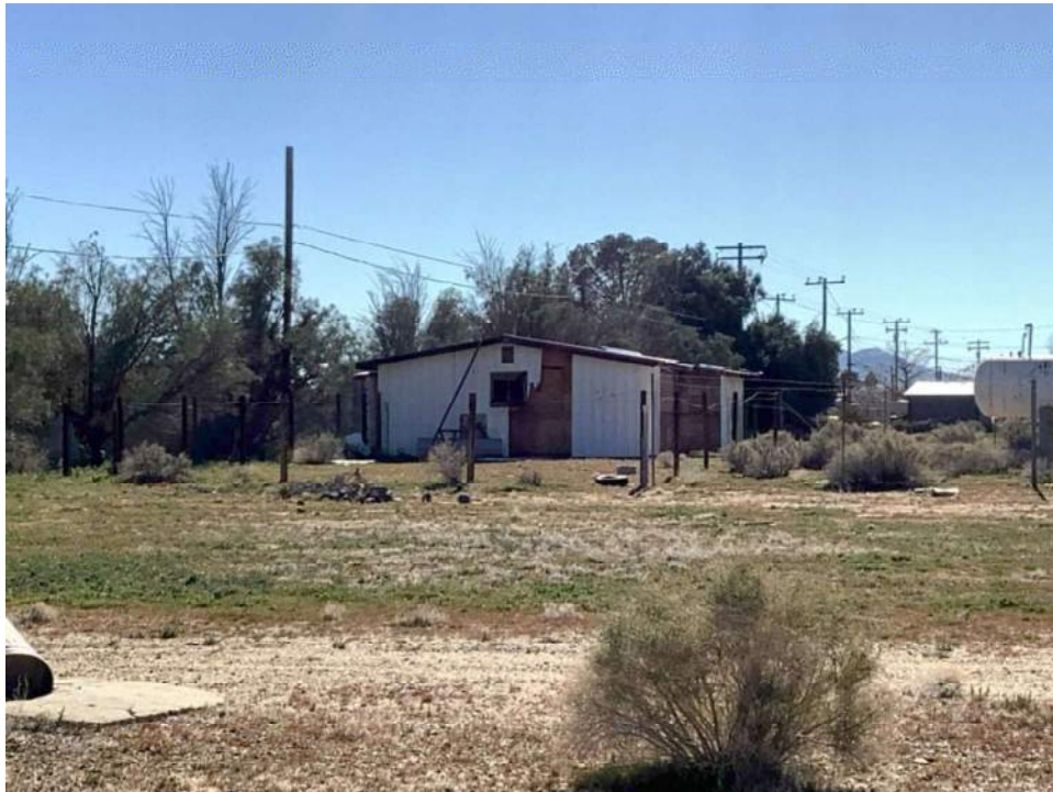
Photo 4. Side façade, view toward south.
