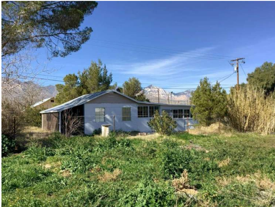
Photo 2. Side façade, view toward west.
