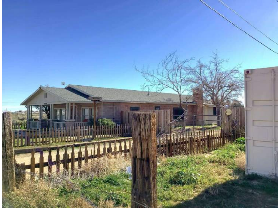
Photo 1. East facade, view toward southwest.
