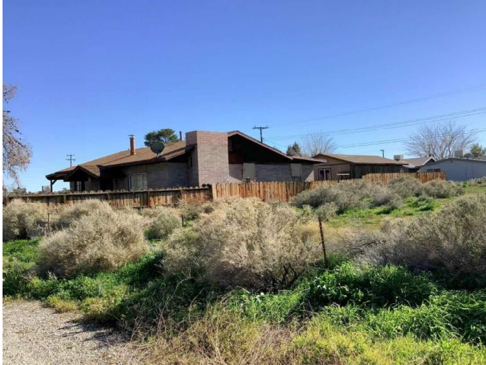
Photo 1. North and east facades, view toward southwest.
