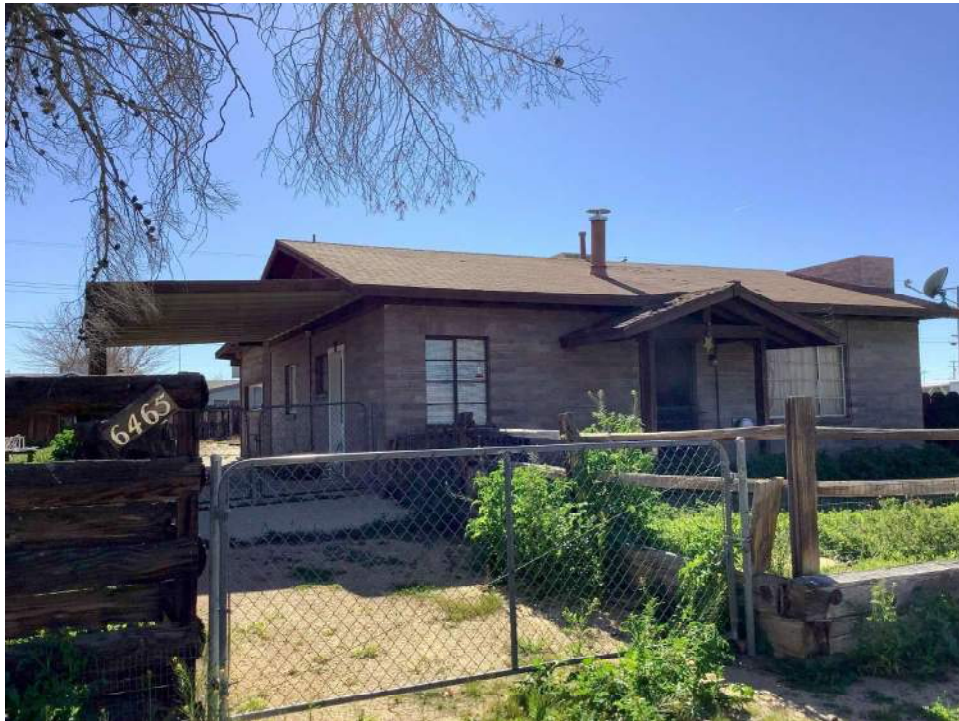
Photo 2. North and west facade, view toward southeast.
