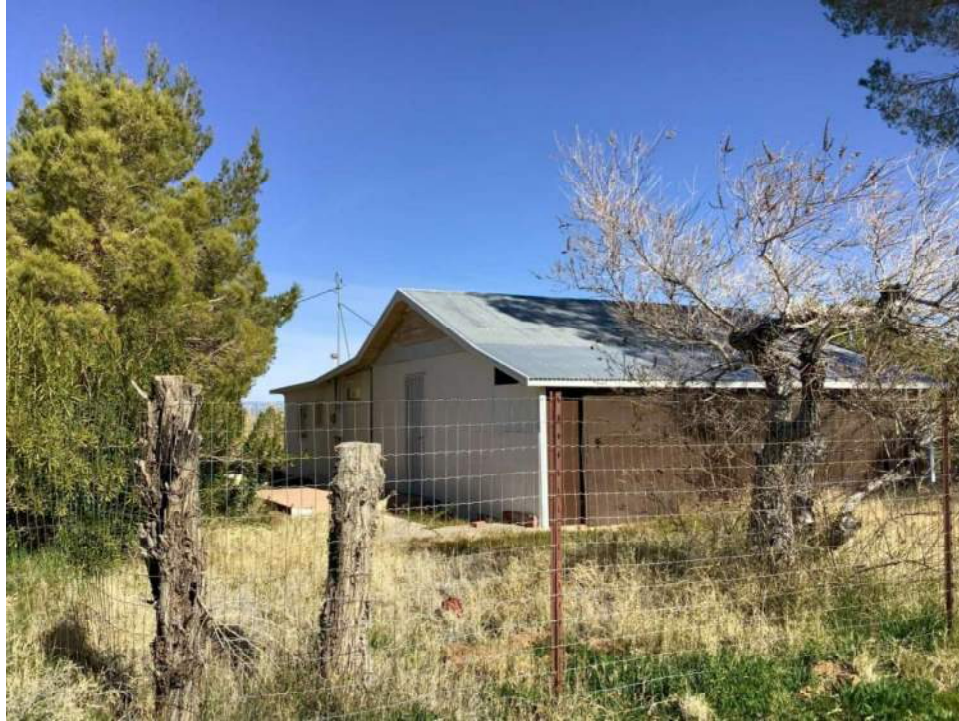
Photo 1. Primary and side façades, view toward northeast.
