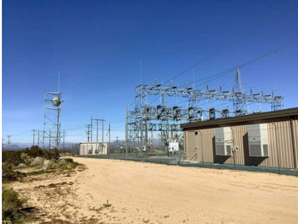
Photo 5. View of both sheds. View toward northeast.
