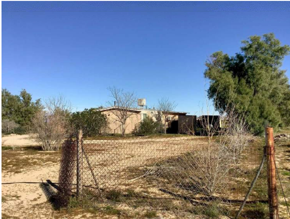
Photo 2. South and east facades, view toward northwest.
