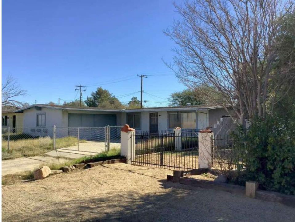
Photo 1. North and east facades, view toward southwest.
