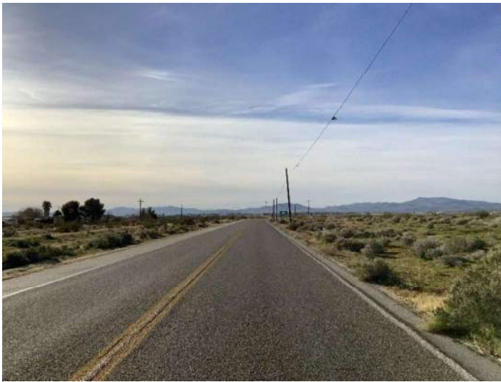
Image 1. Segment 1, Brown Road, just above the intersection of present Highway 395.
