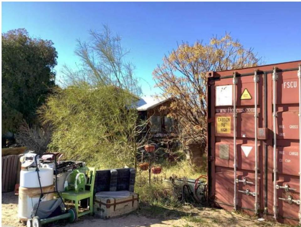
Photo 4. Rear façade and addition, view toward southwest.
