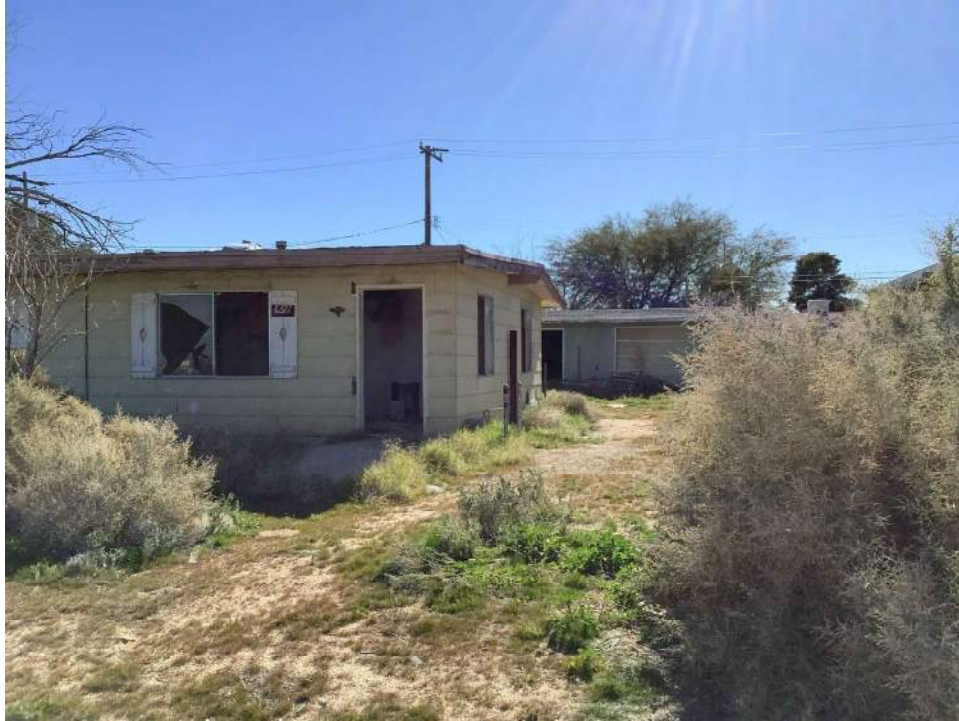
Photo 1. North and east facades, view toward southwest.
