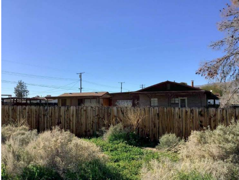
Photo 3. West façade, view toward east.
