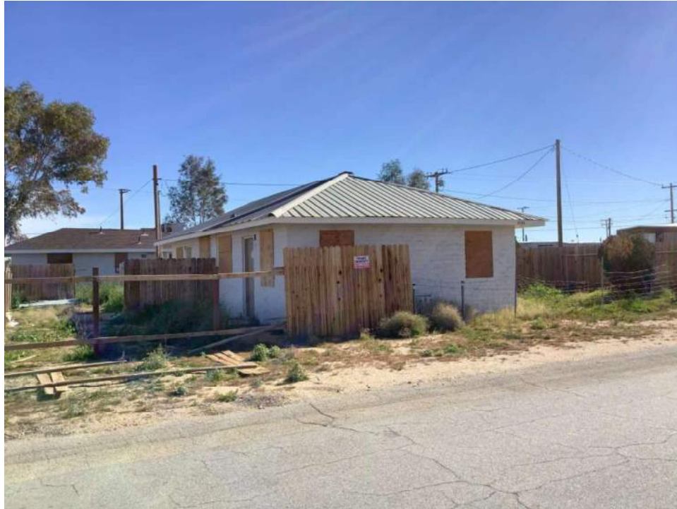
Photo 7.: Building Three: View toward southeast.
