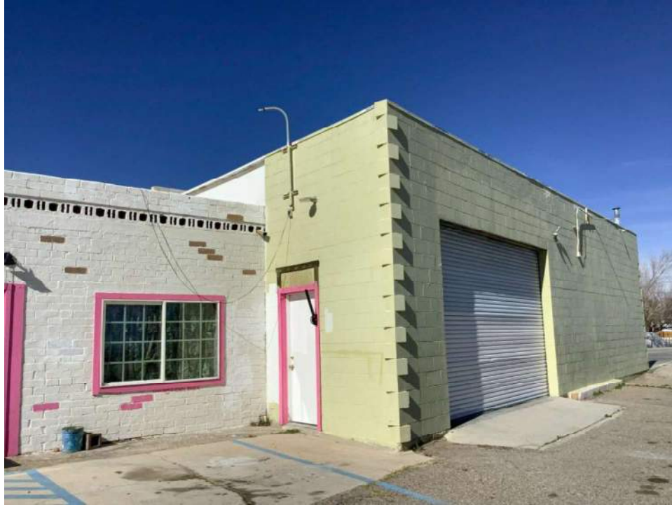
Photo 5. Façade of original section of building and addition facing Brown Road, view toward northwest.
