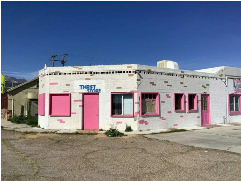
Photo 6. Detail of southern section of the building. View toward northwest.
