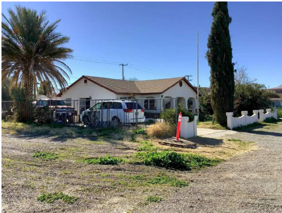
Photo 2. North and west facade, view toward southeast.
