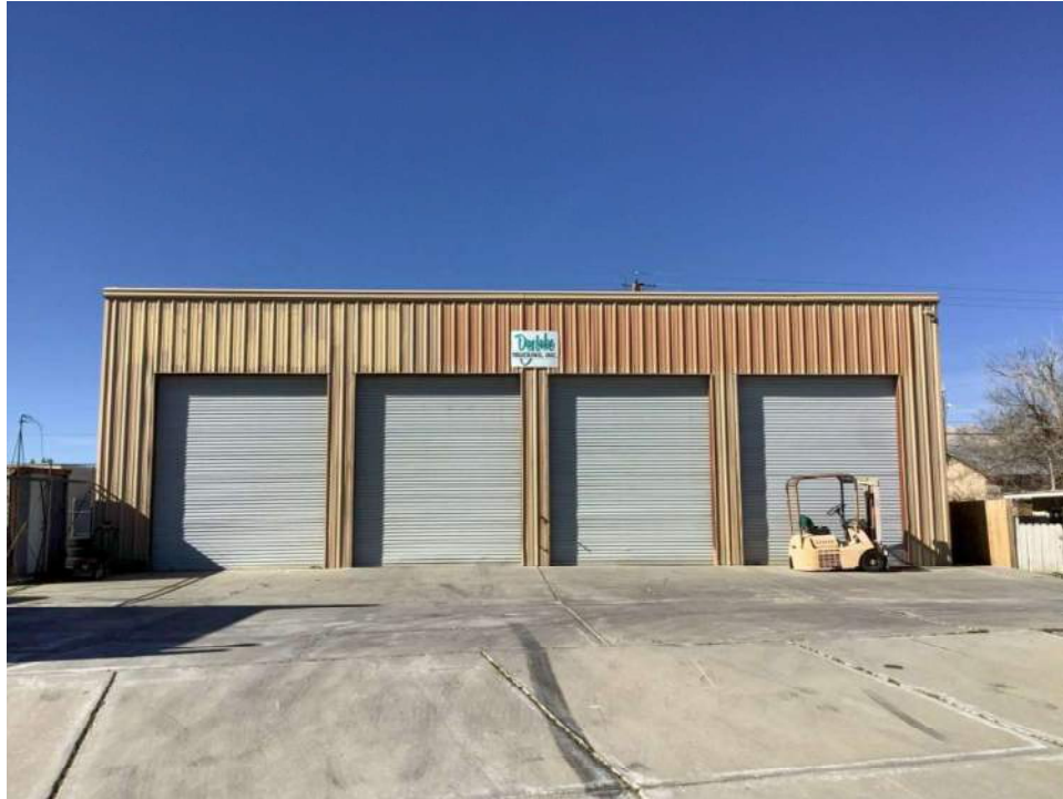
Photo 5. Commercial garage building. View toward west. View from Brown Road.
