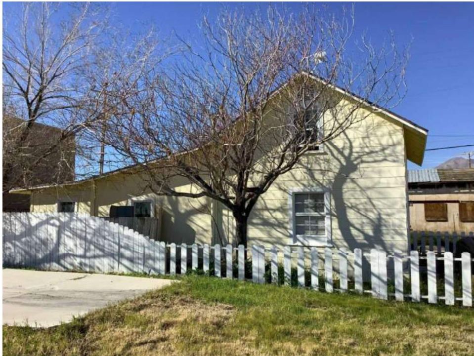
Photo 2. Side façade, view toward west. View from Brown Road.
