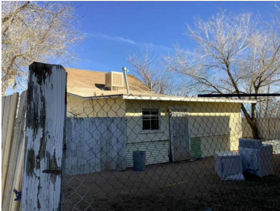
Photo 4. Rear façade, view toward northeast.
