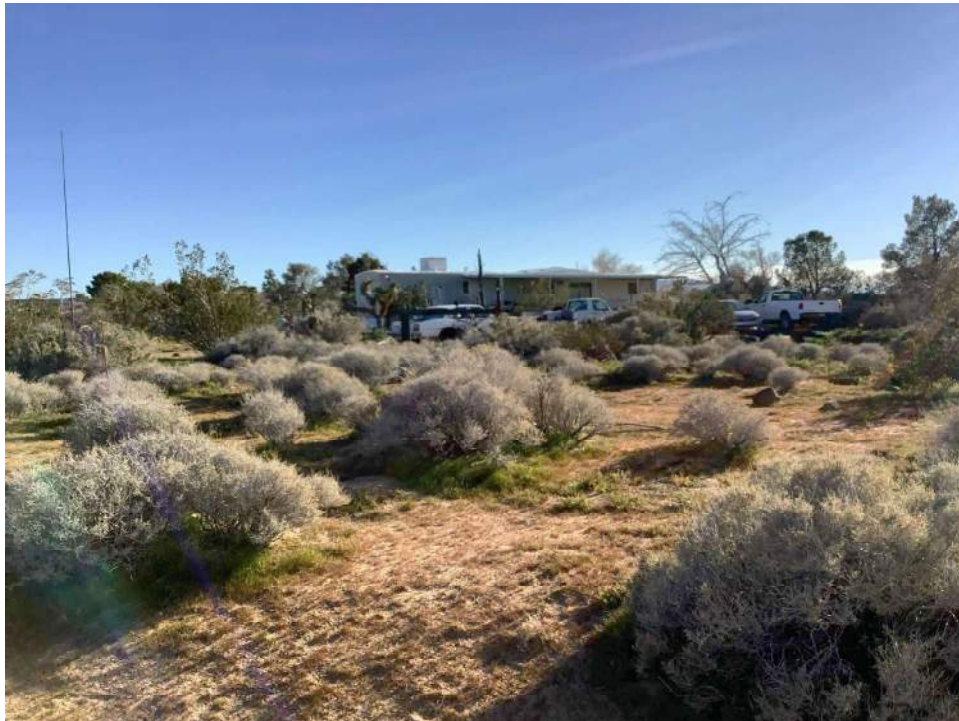
Photo 2. North and east facades, view toward southwest.
