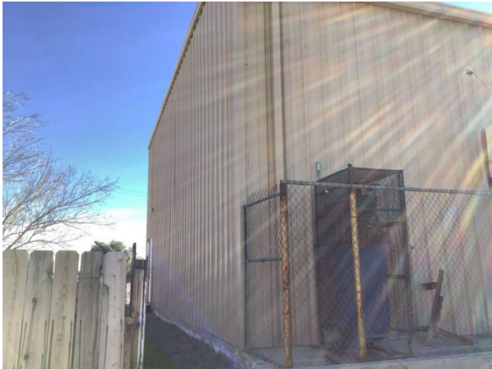
Photo 6. Detail of alley between 101 Ash Avenue (residence) and commercial garage building.
