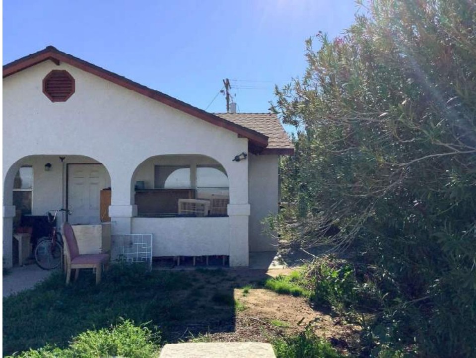
Photo 1. Detail image of north facade, view toward south.
