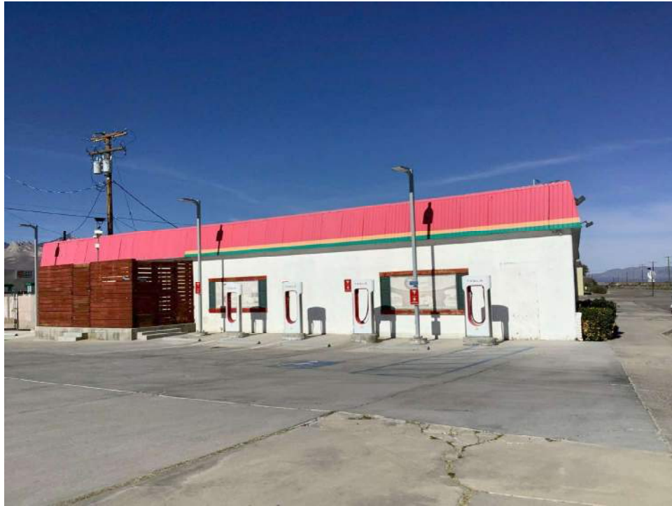
Photo 1. Rear façade, view toward north.
