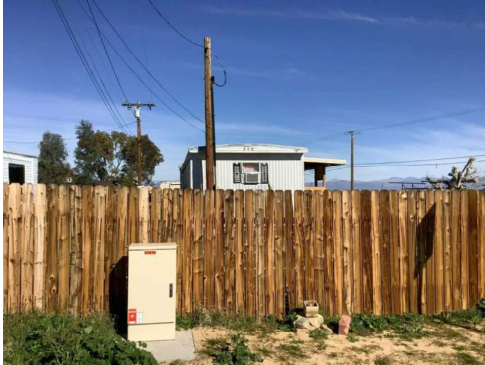
Photo 3. Side façade, view toward north.
