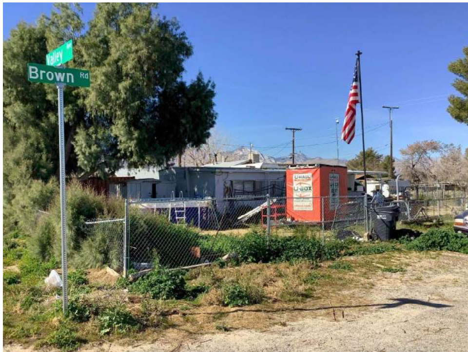
Photo 2. South and west facades, view toward northeast.
