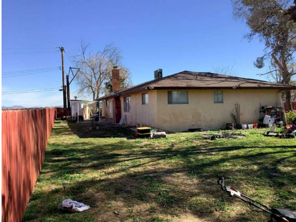
Photo 1. East and north facades, view toward west.
