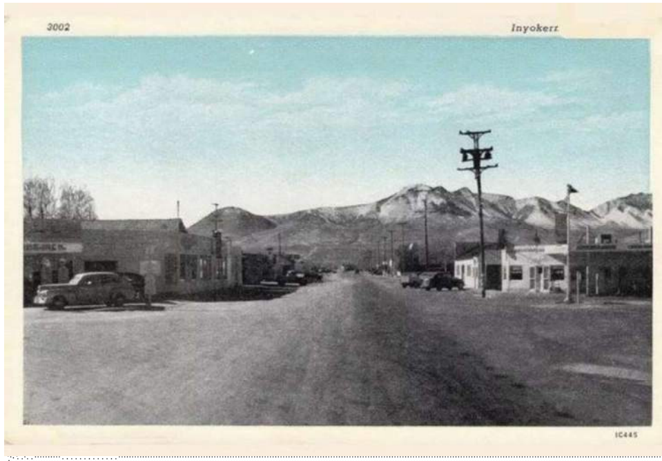
Figure 5.1 Inyokern 1951; 1401 N Brown Road visible
