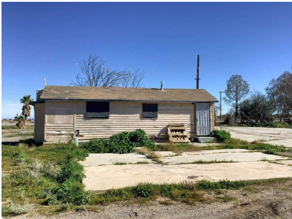
Photo 3. North façade of building three, view toward south.
