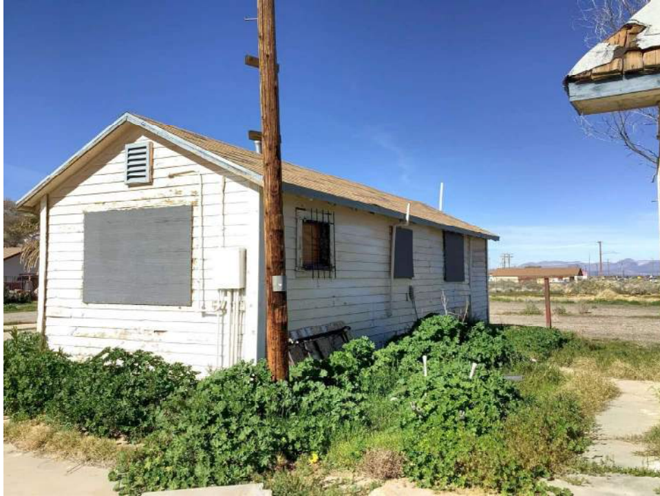
Photo 3. South and east facades of building three, view toward northwest.
