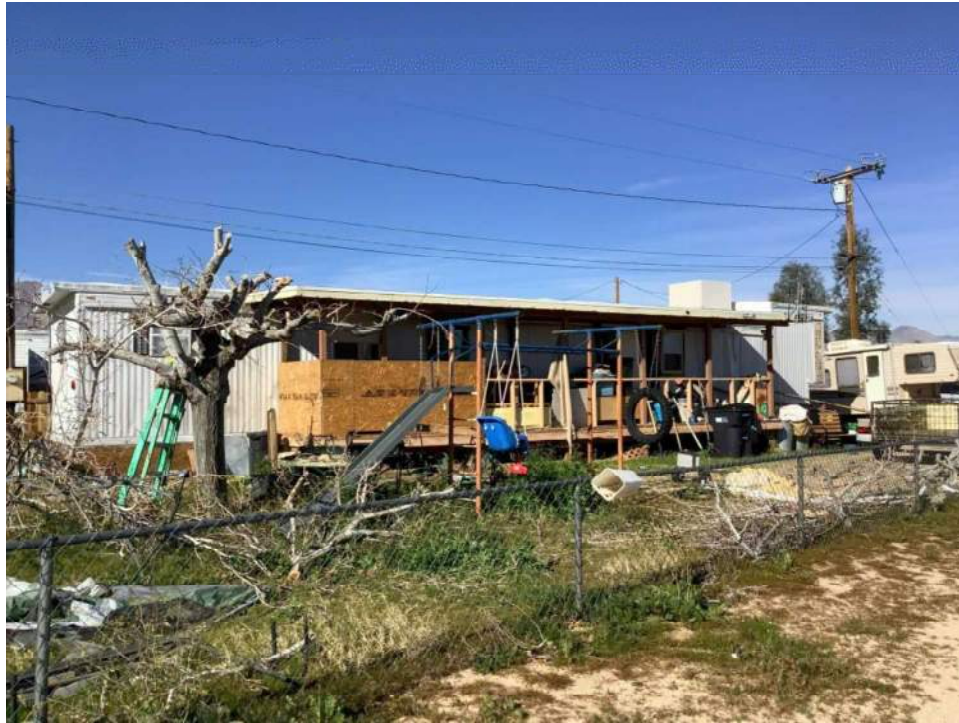
Photo 1. Primary façade facing Brown Road. View toward west.
