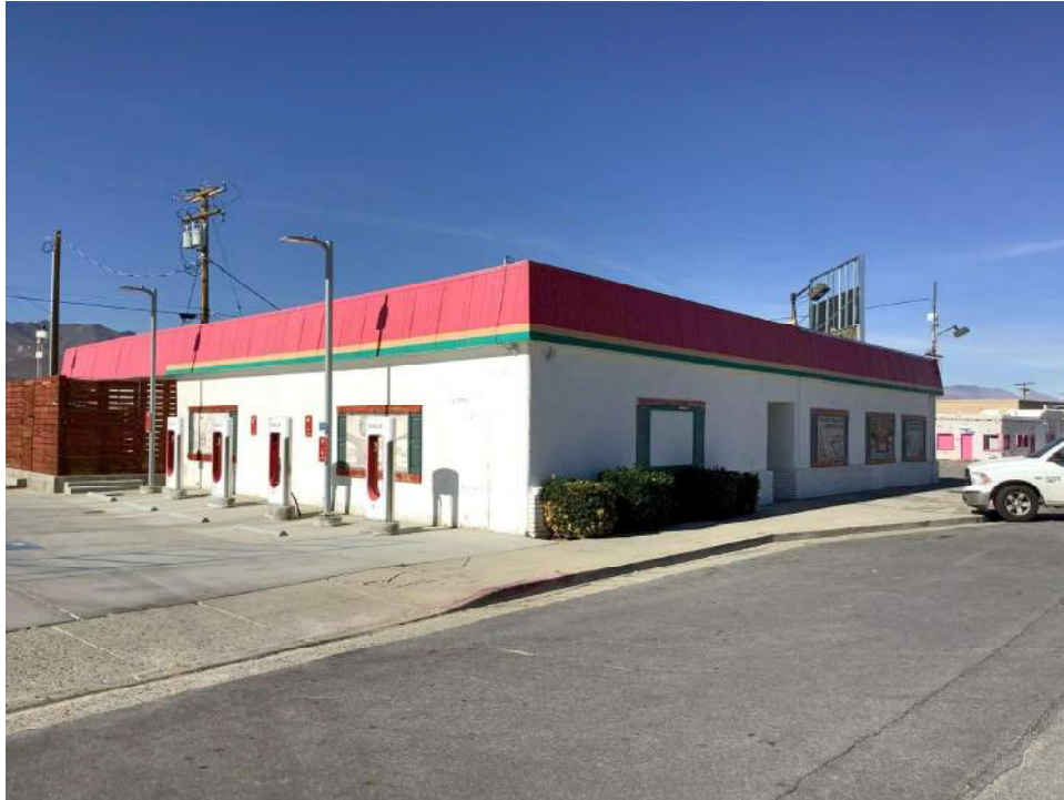
Photo 5. South and west facades, view toward northeast.
