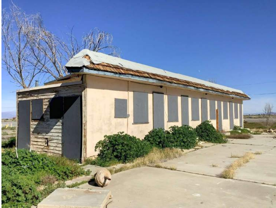
Photo 1. South façade of building two, view toward northwest.
