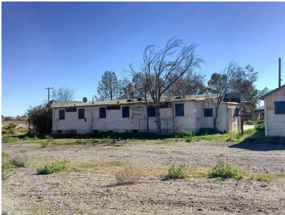
Photo 2. North façade of building two, view toward south.
