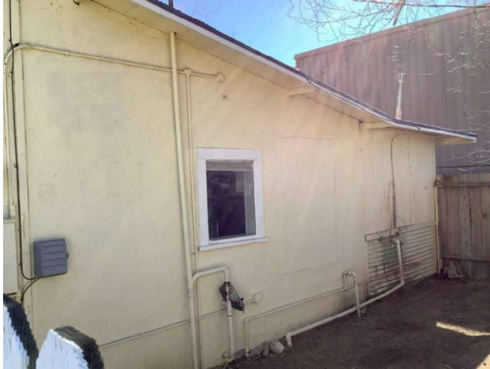
Photo 3. Detail of addition area of side façade. View toward southeast.
