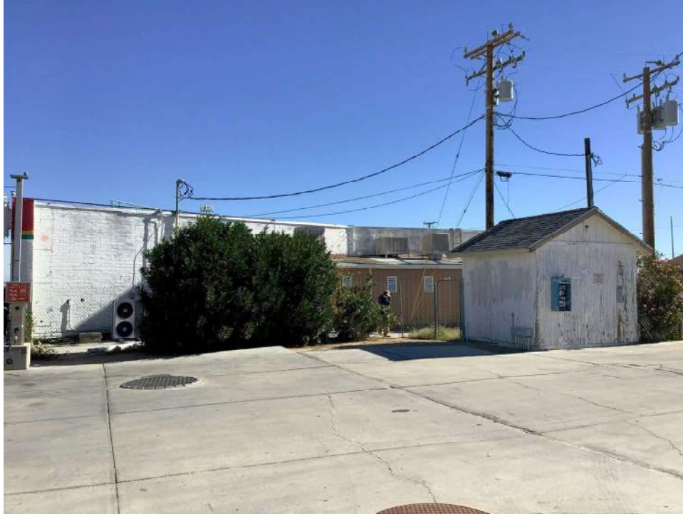
Photo 3. View of east façade. View toward west.
