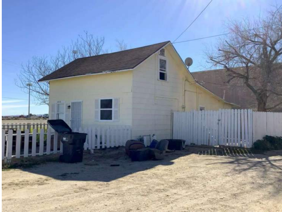
Photo 1. Primary and side façades, view toward southeast.
