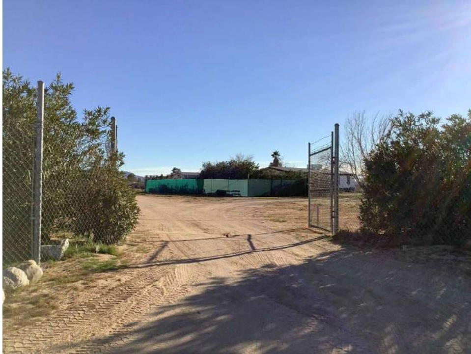
Photo 3. West façade, view toward southeast.
