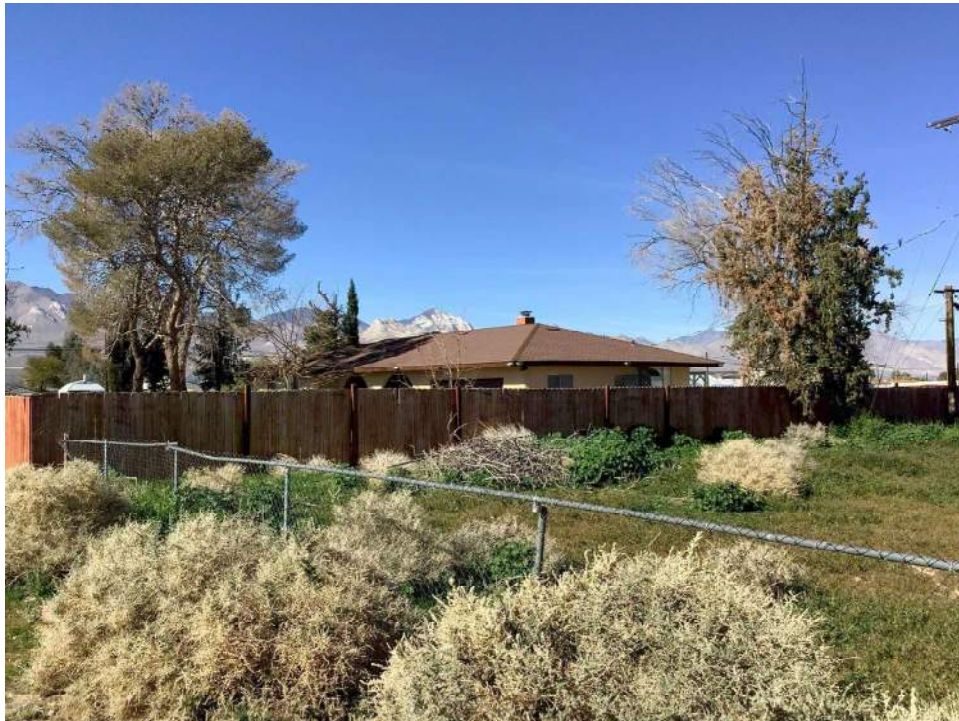
Photo 2. West facade, view toward northeast.
