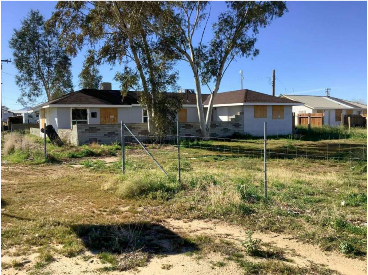
Figure 4.5.1 1447 N Brown Road (Building One), view toward northwest.
