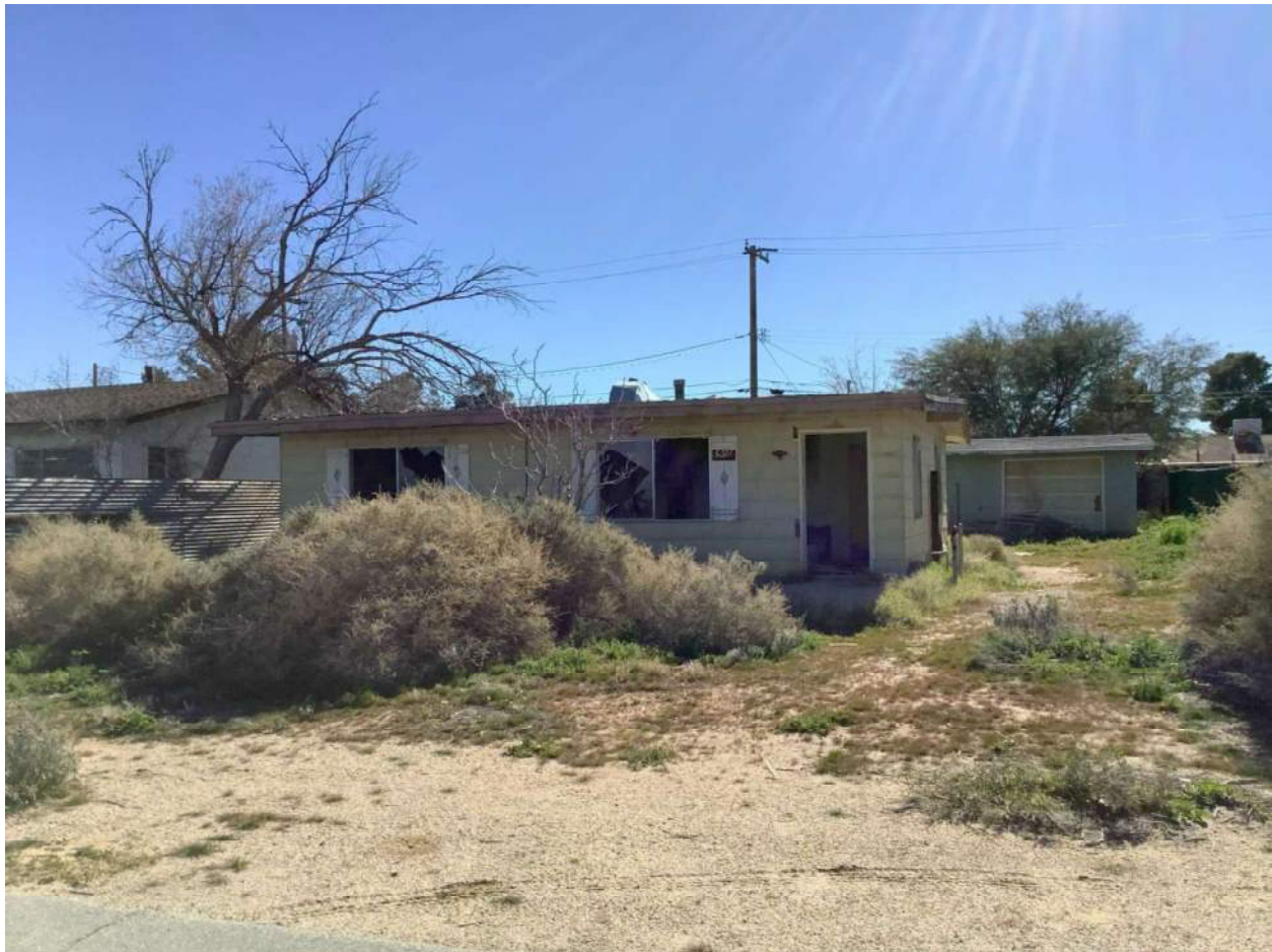
Figure 4.13 6517 Sunset Avenue, view toward south.
