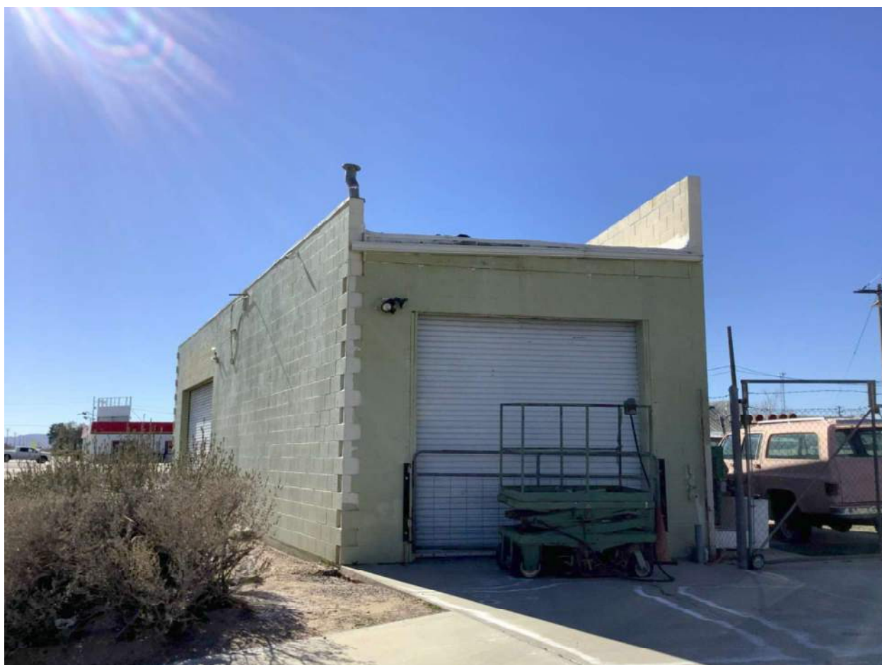
Figure 4.8.3 Addition (1966) to 1401 N Brown Road, view toward south.
