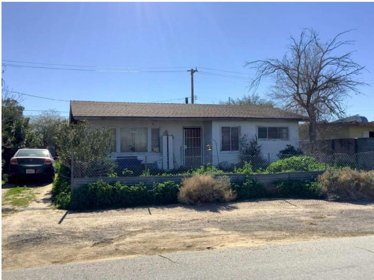
Figure 4.14 6513 Sunset Avenue, view toward south.
