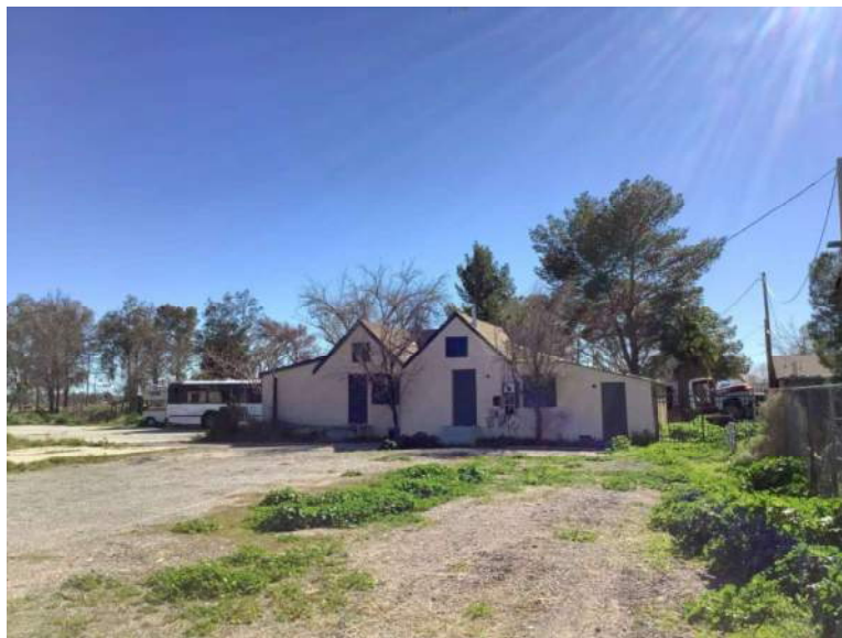
Figure 4.16.1 1233 N Brown Road (Building One), view toward south.
