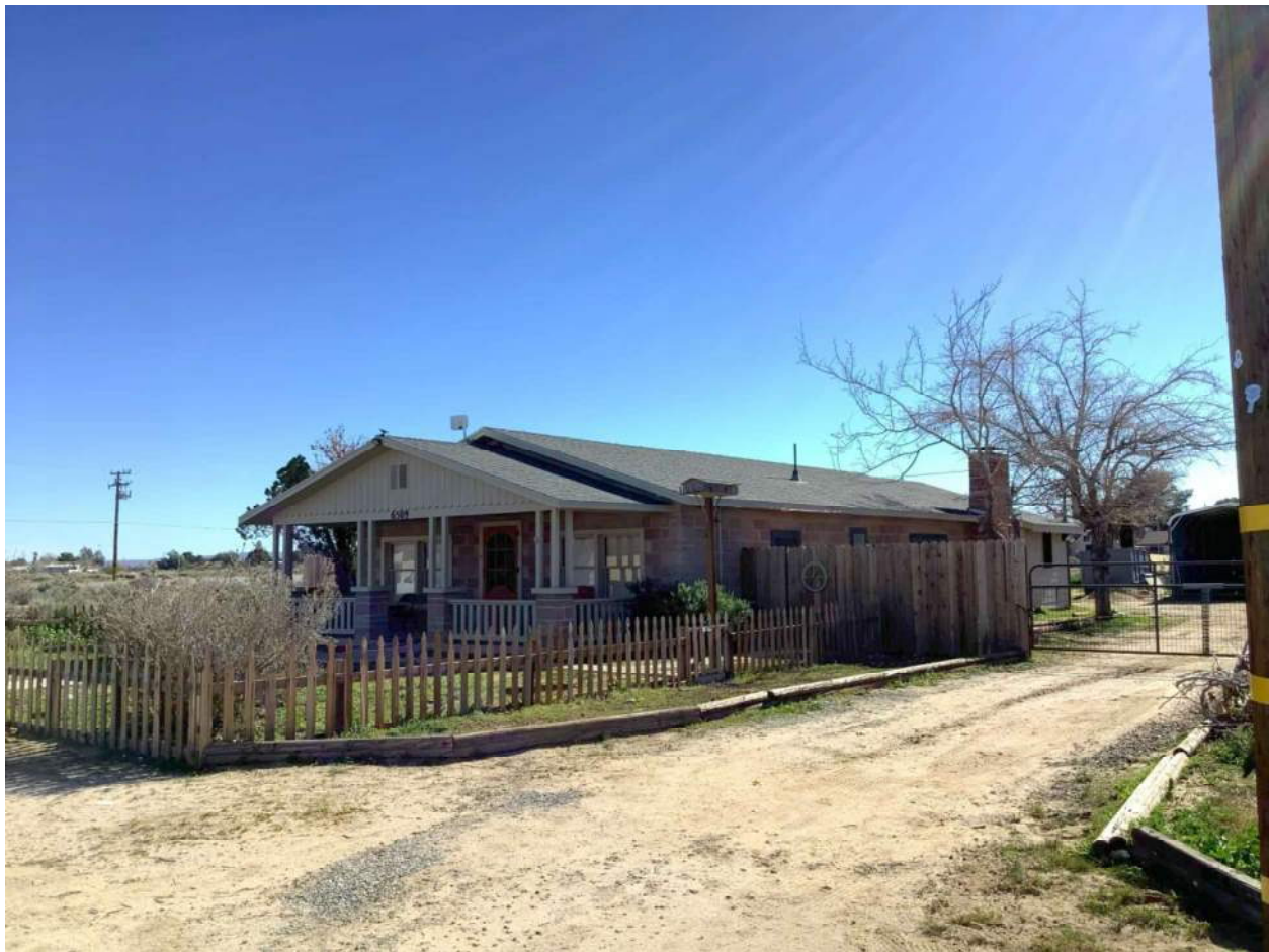
Figure 4.10 6509 Locust Avenue, view toward southwest.
