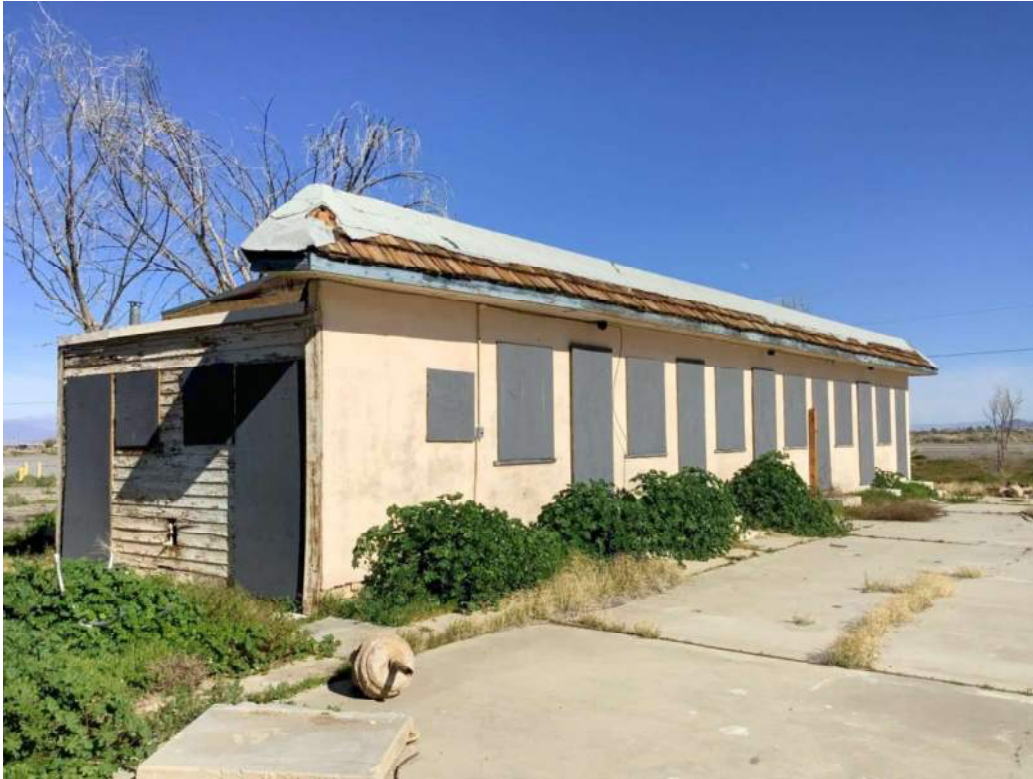
Figure 4.16.2 1233 N Brown Road (Building Two), view toward northwest.
