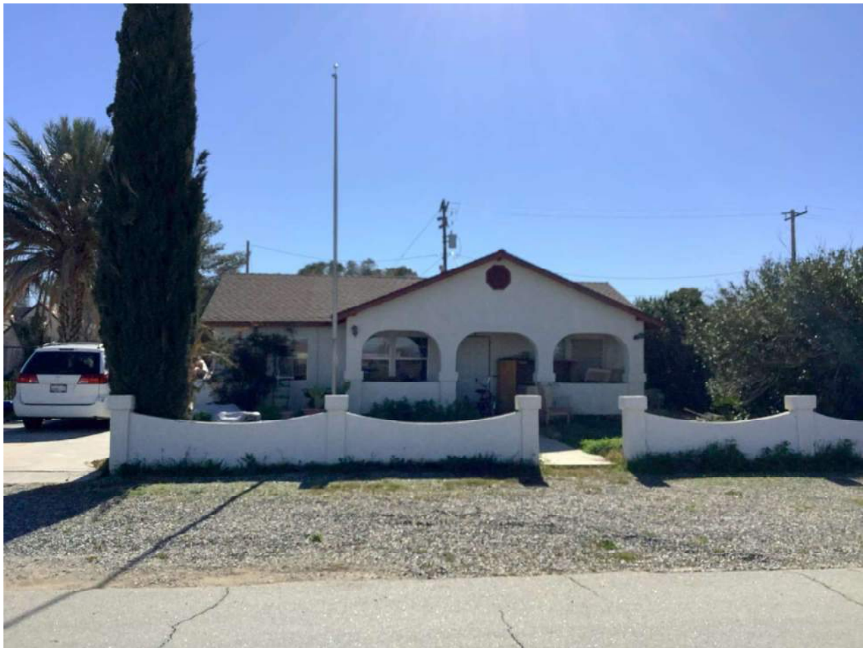
Figure 4.15 109 Sunset Avenue, view toward south.
