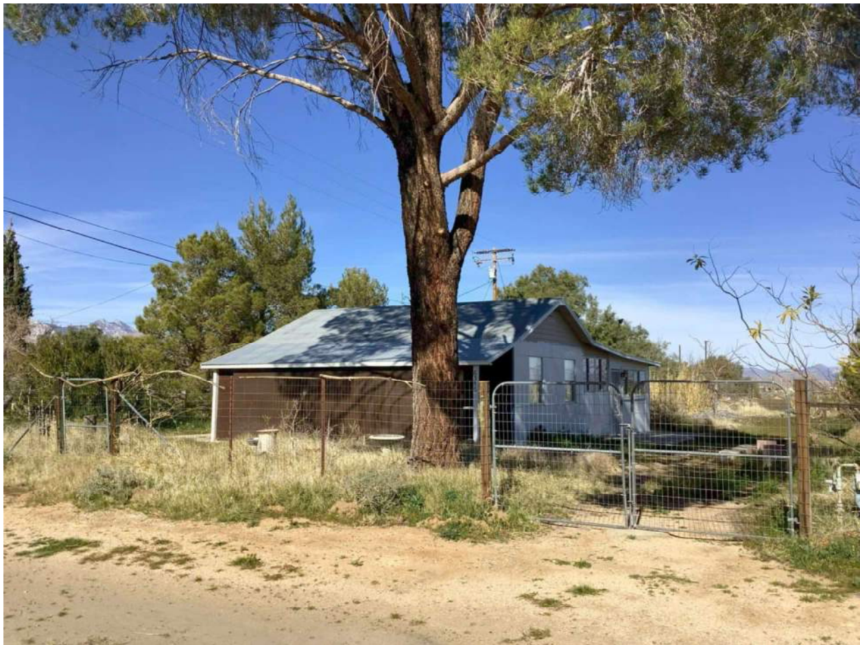
Figure 4.3 6546 Orchard Avenue, view toward northwest.
