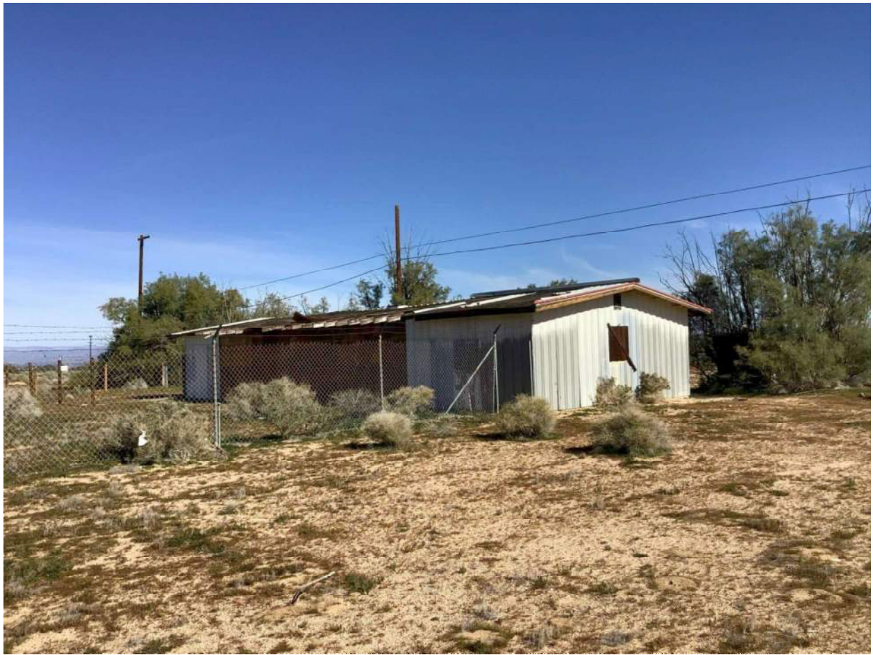
Figure 4.2 1520 Second Street, view toward northeast.
