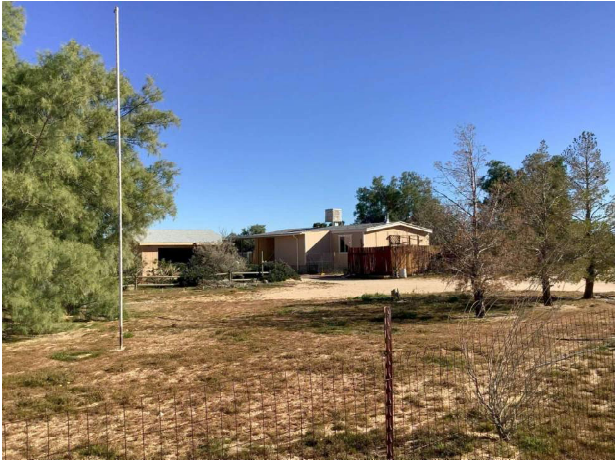
Figure 4.27 View of 1540 N Mercury Street, view toward west.
