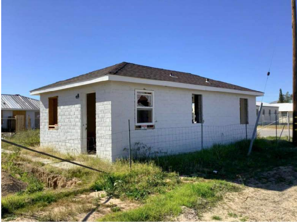
Figure 4.5.2 1447 N Brown Road (Building Two), view toward northwest.
