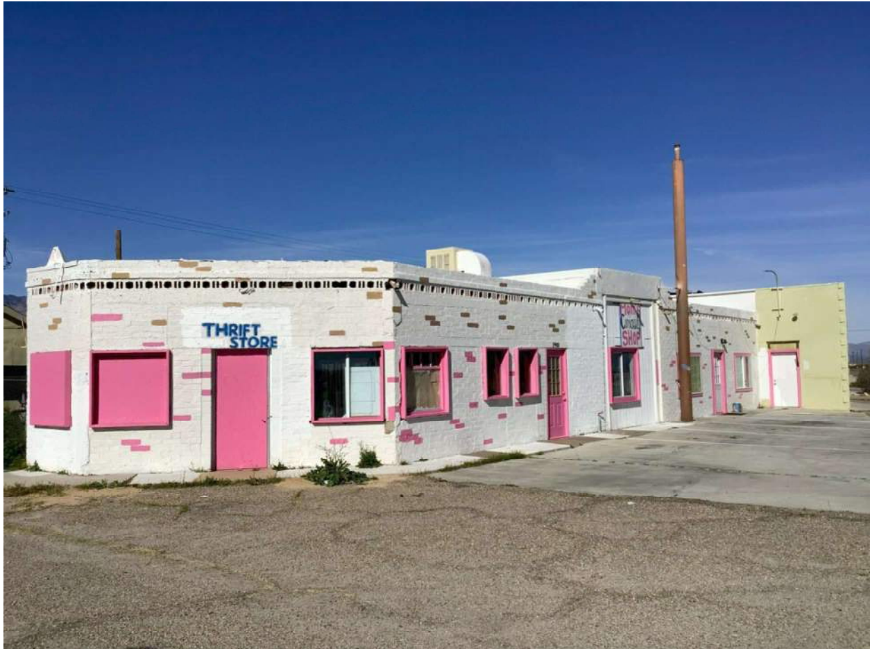
Figure 4.8.1 1401 N Brown Road, view toward northwest.
