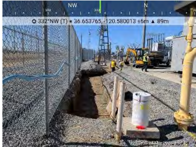
End of day trenching. Around mid point reached.
