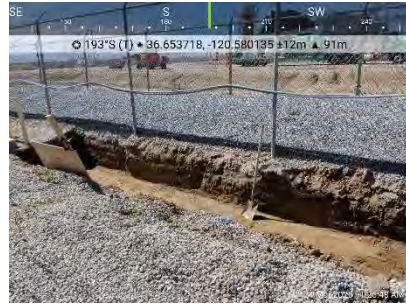
Max 3ft depth at middle of fenceline
