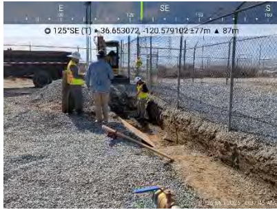
End of day trench.
