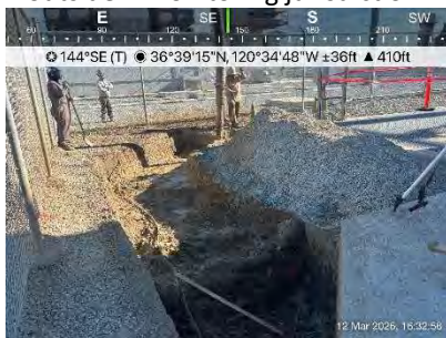
End of day, extent of trench
