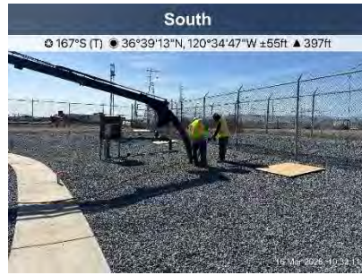
Crew making the potholes at designated distances from each other
