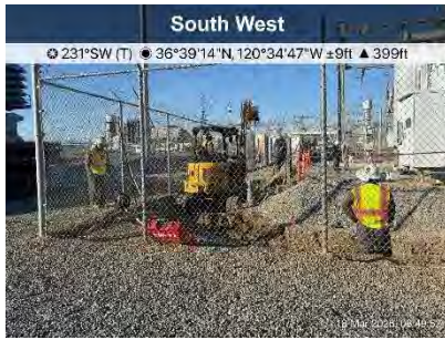
Beginning of day, first usage of excavator inside of the GSU
