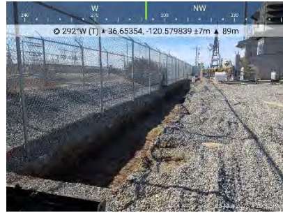
End of day trench (1/2)
