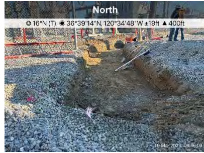
Conclusion of excavation for this week
