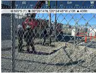
Holes that were excavated using the hydrovac
