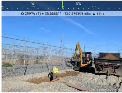
Start of day trenching along innerpeaker plant fence.
