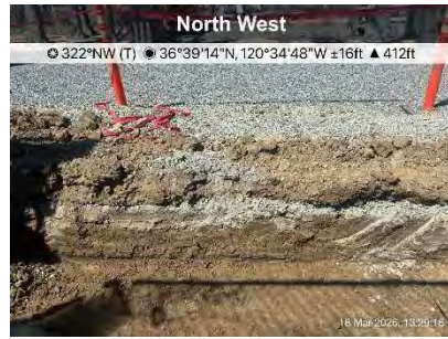
Sidewall of trench
