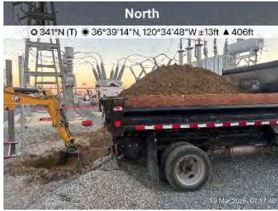
Spoil inspection after removal.
