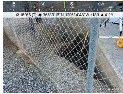
Continuation of trench from the 3ft pit.
