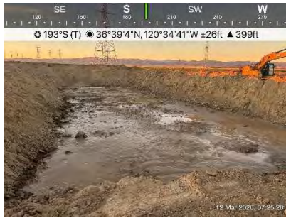
Spoil dump site that was inspected. However, it's a conglomerate for all "wet spoils" from across the entire plant so it is contaminated with spoils from outside if monitoring jurisdiction.
