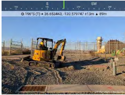
Gravel removal at S end of plant fenceline
