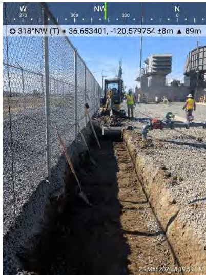
End of day trench (2/2)
