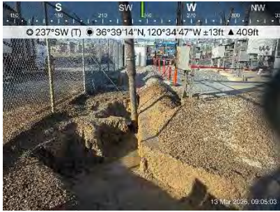
Beginning of day, trenching continuing
