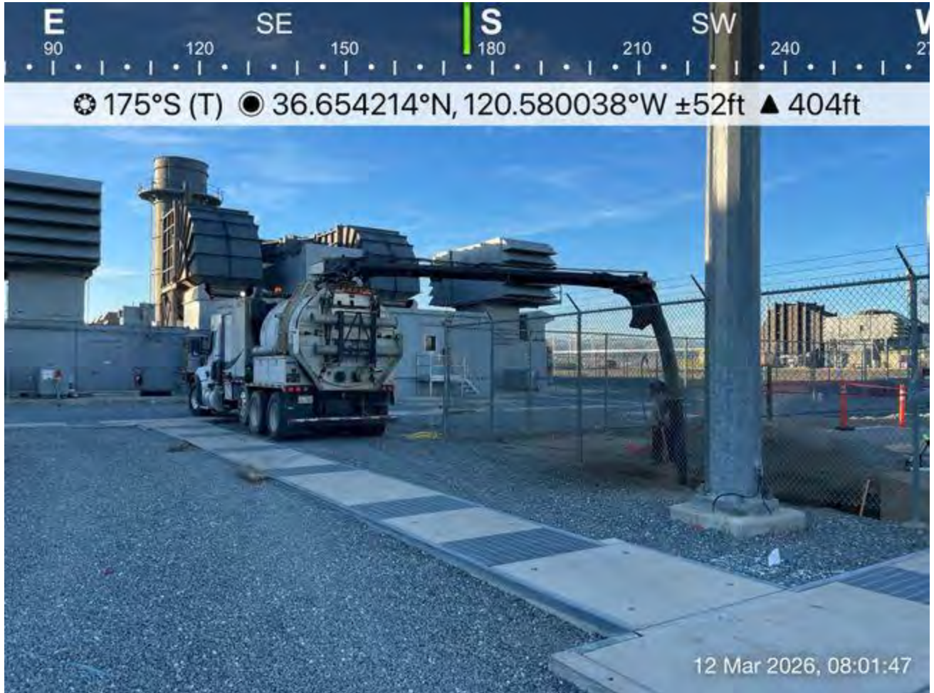
Hydrovac works begins
