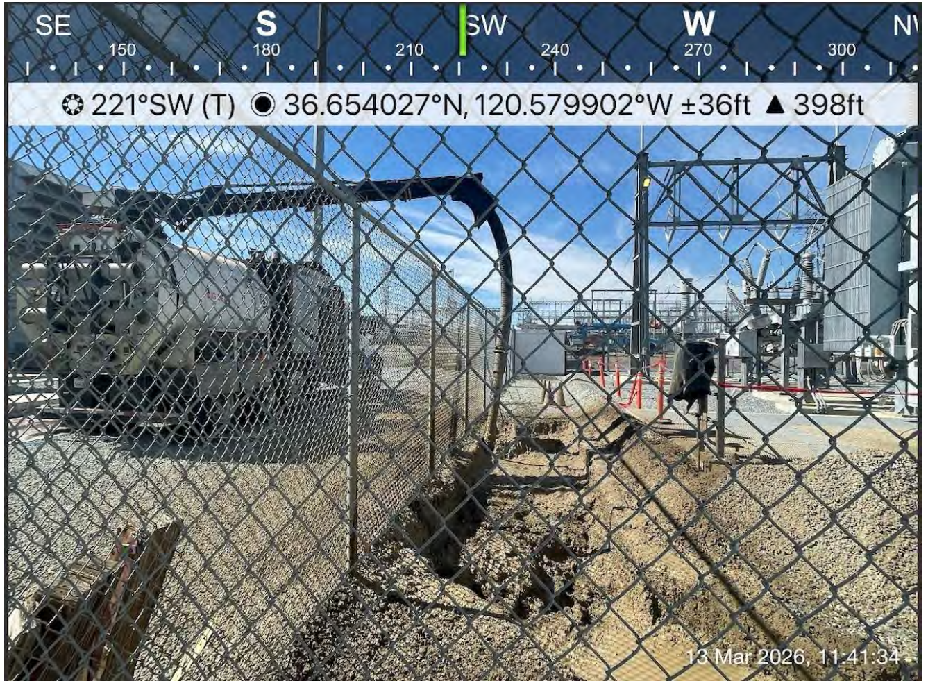
Continued hydrovac work
