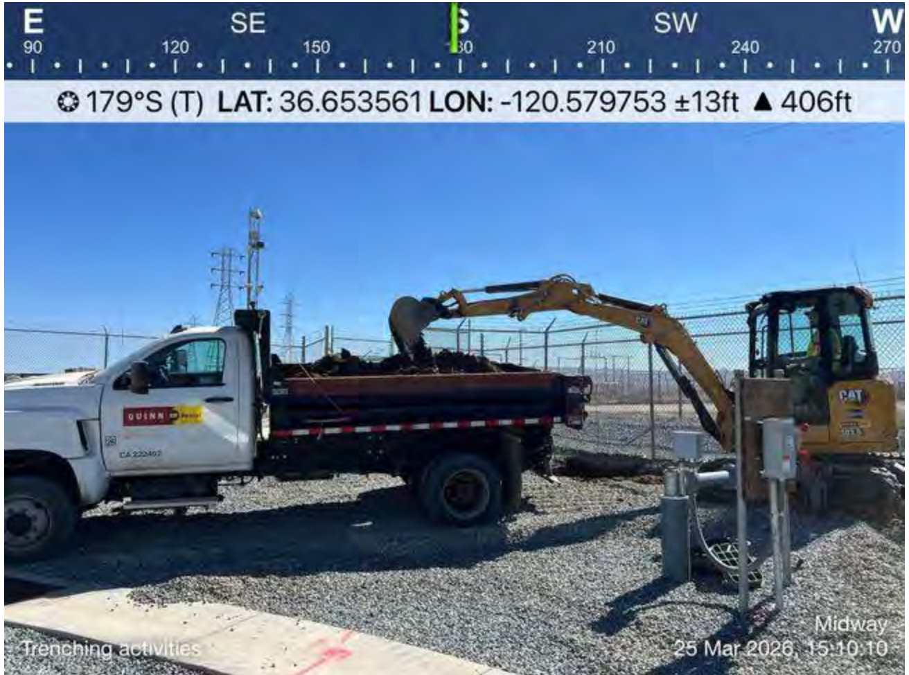
Trenching earthwork activities continued.
