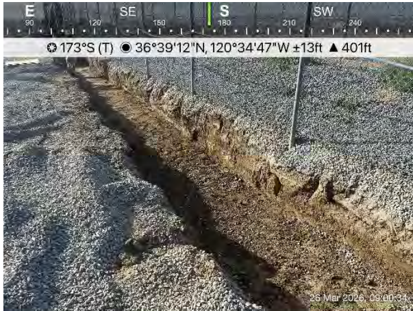
09:00 Facing south Teichert overview of completed section of trench.
