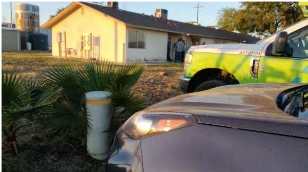
07:29 Facing south Preconstruction meeting
