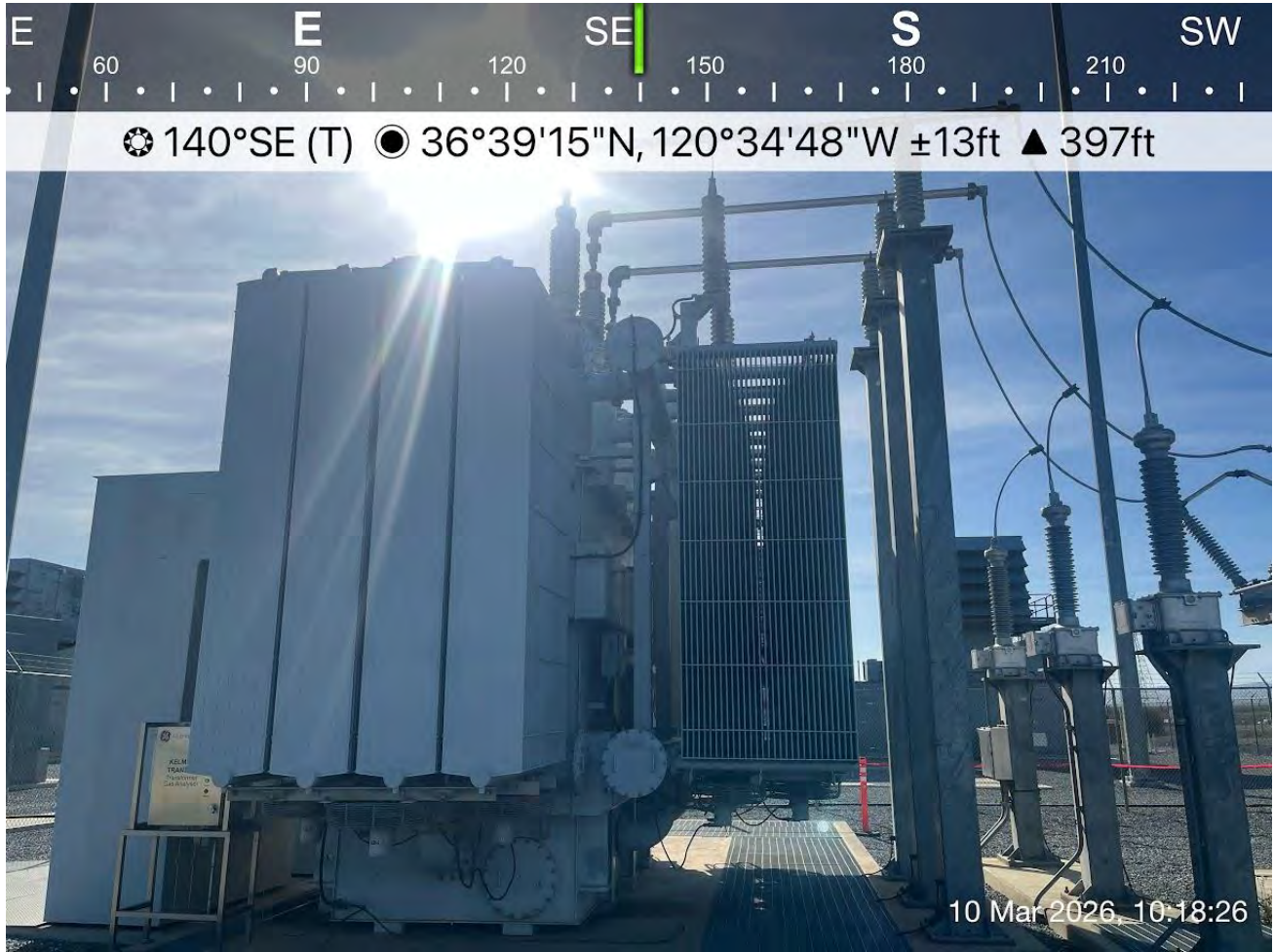
Photo 1: Heat sinks in substation where potential HOFI nests were located.
