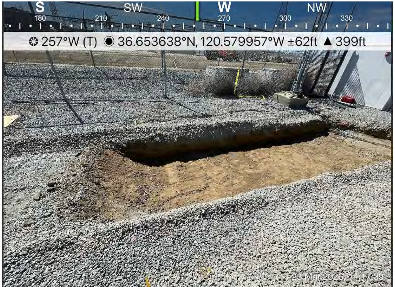
Trench with earthen wildlife escape ramp installed
