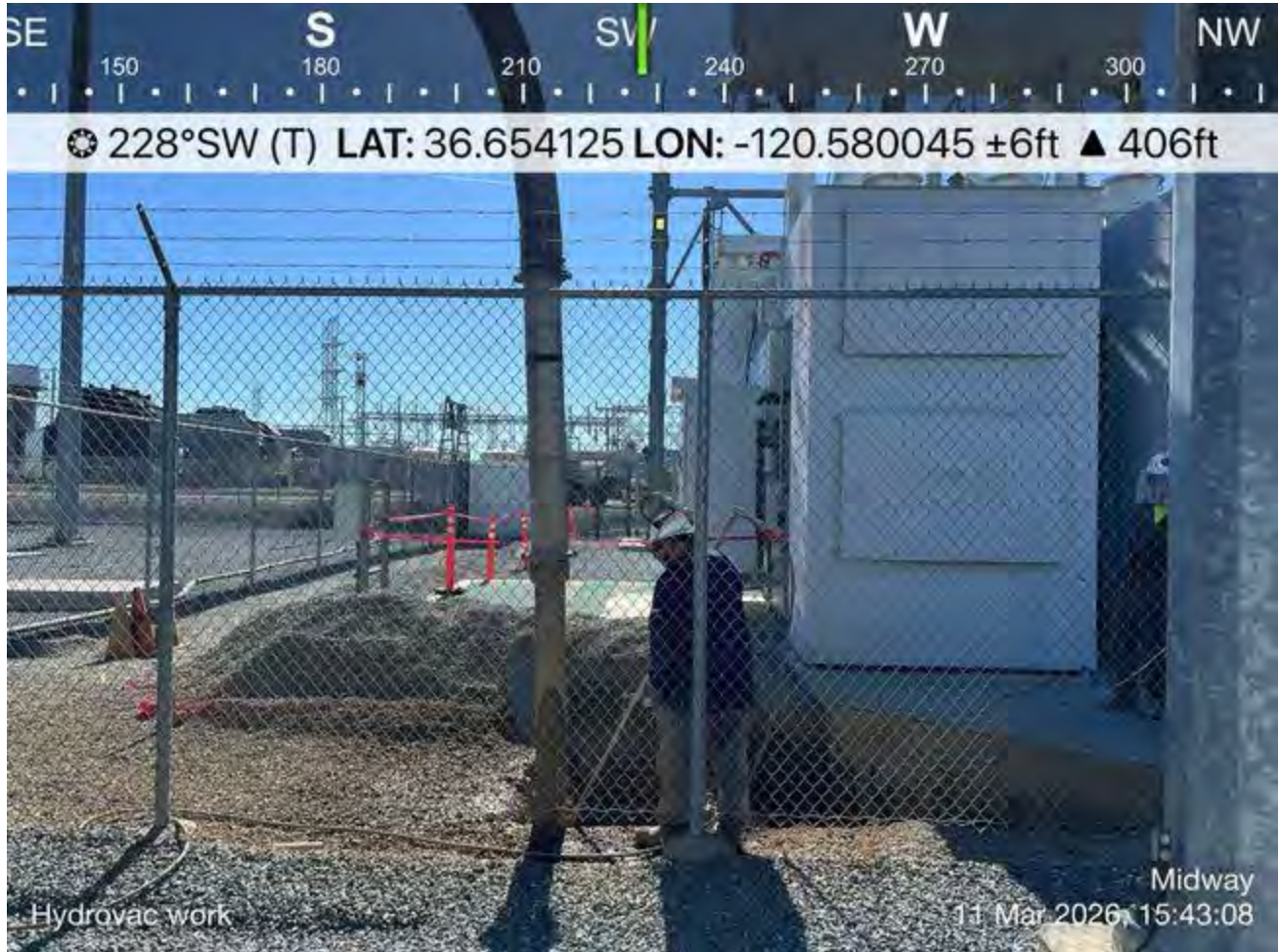
Hydrovac work activities continued.
