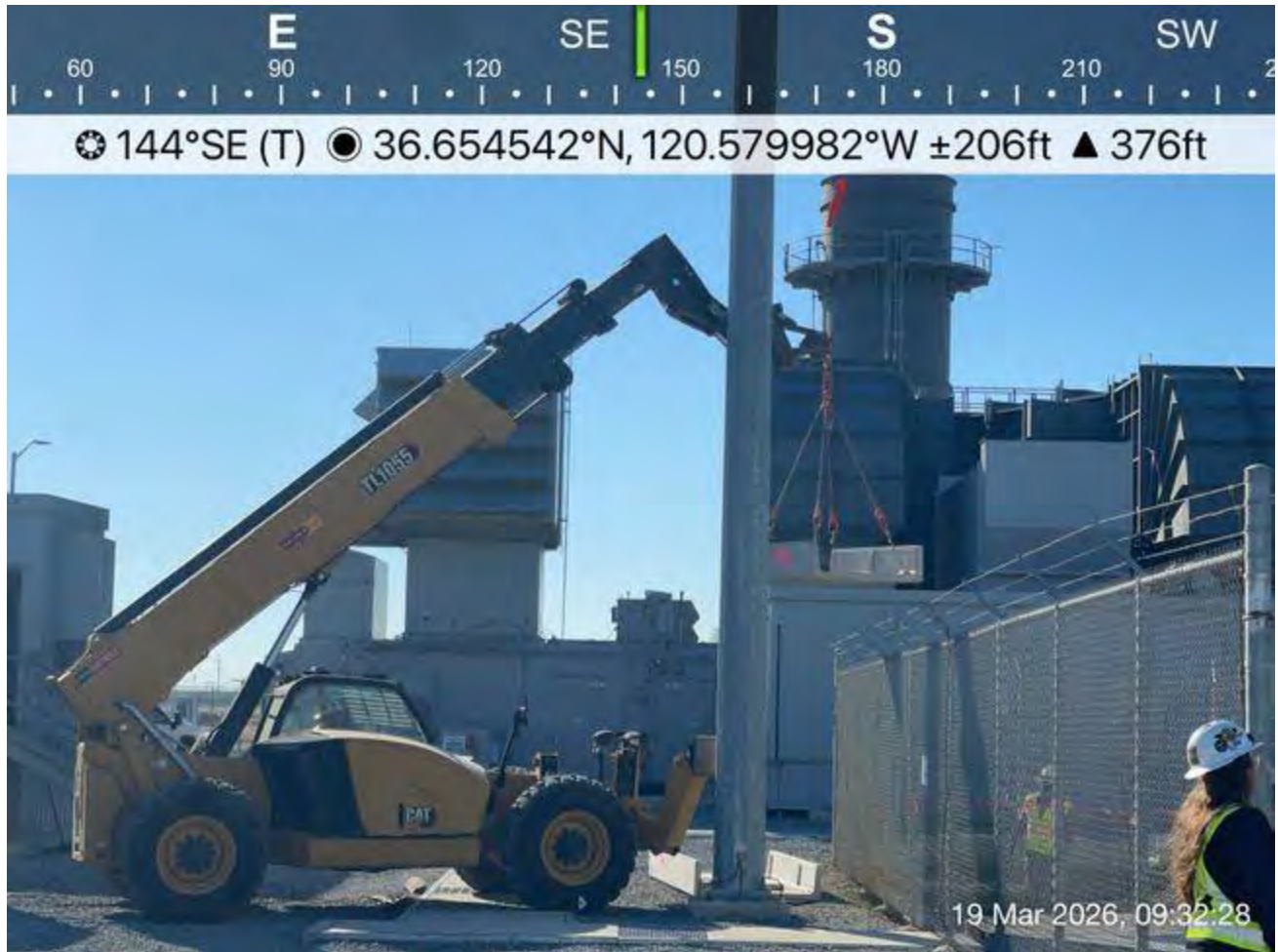
Placement of concrete runs
