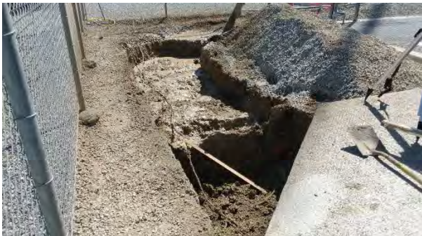
13:42 Facing southwest Trench overview
