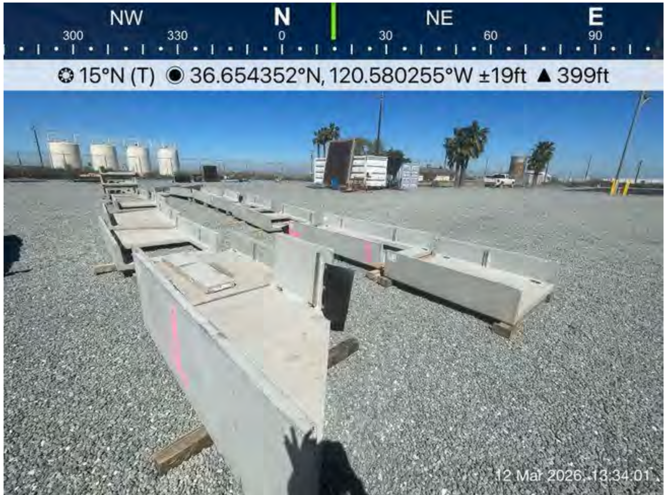
Delivery of materials in peaker plant
