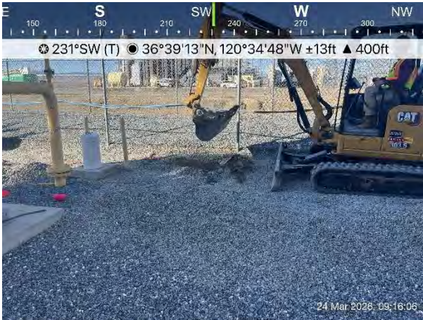
09:16 Facing southwest Teichert excavating the trench.
