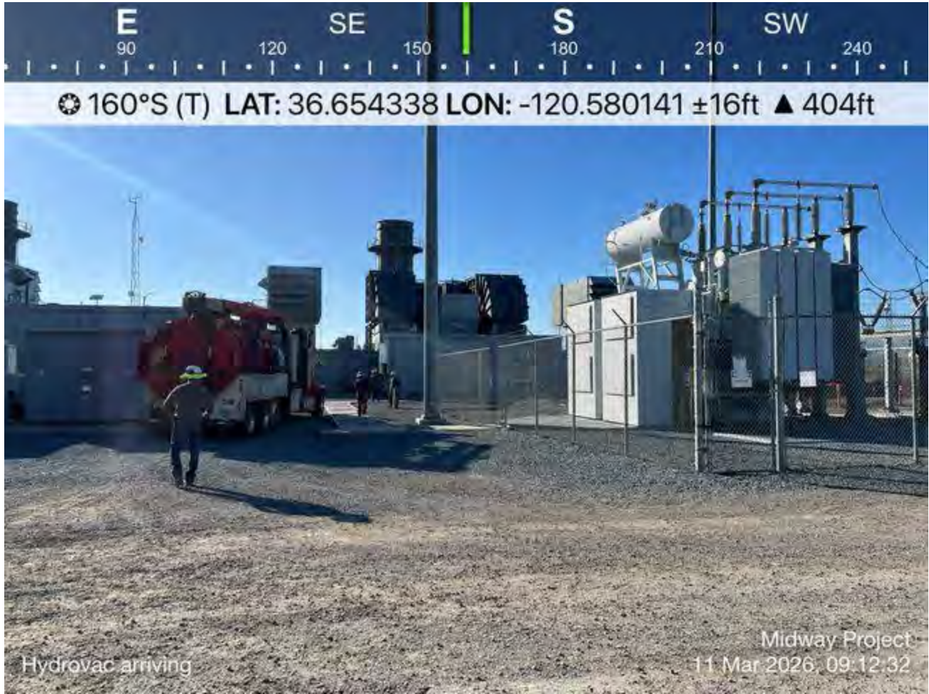
Hydrovac truck arriving on site.
