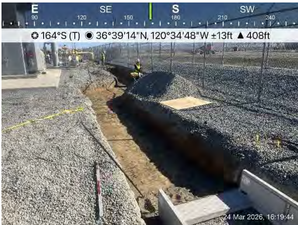
16:19 Facing south End of the day overview of excavated trench
