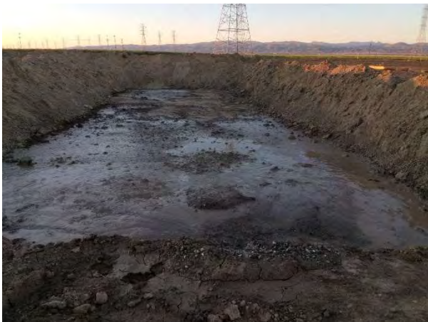
07:36 Facing south Spoils pit overview
