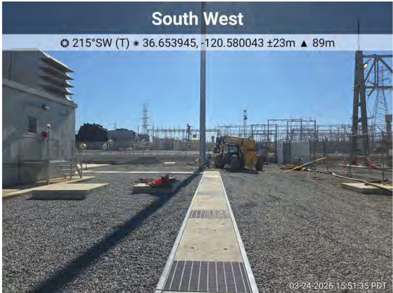
Lowering of concrete runs in trench.
