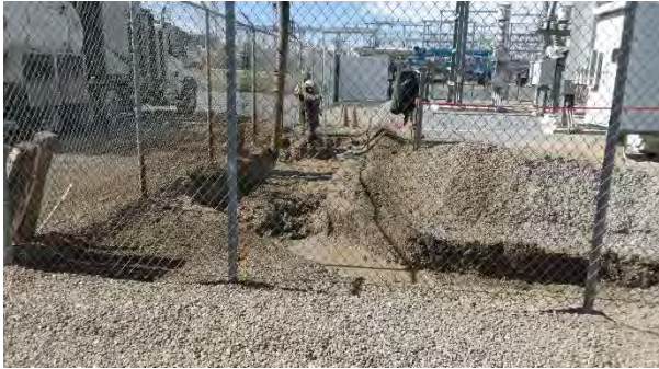
Facing south Potholing in peaker plant
