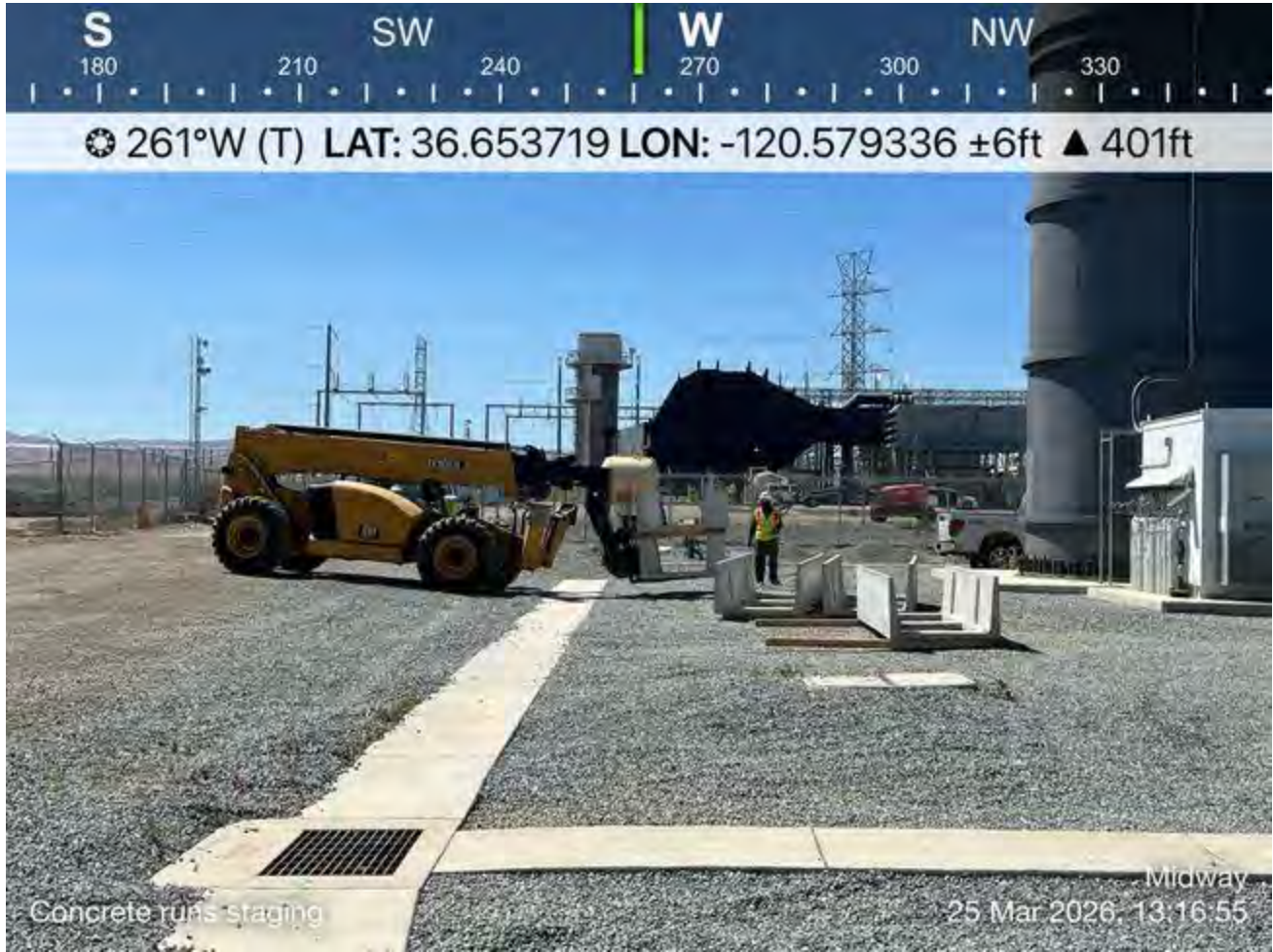
Forklift utilized for concrete run staging.
