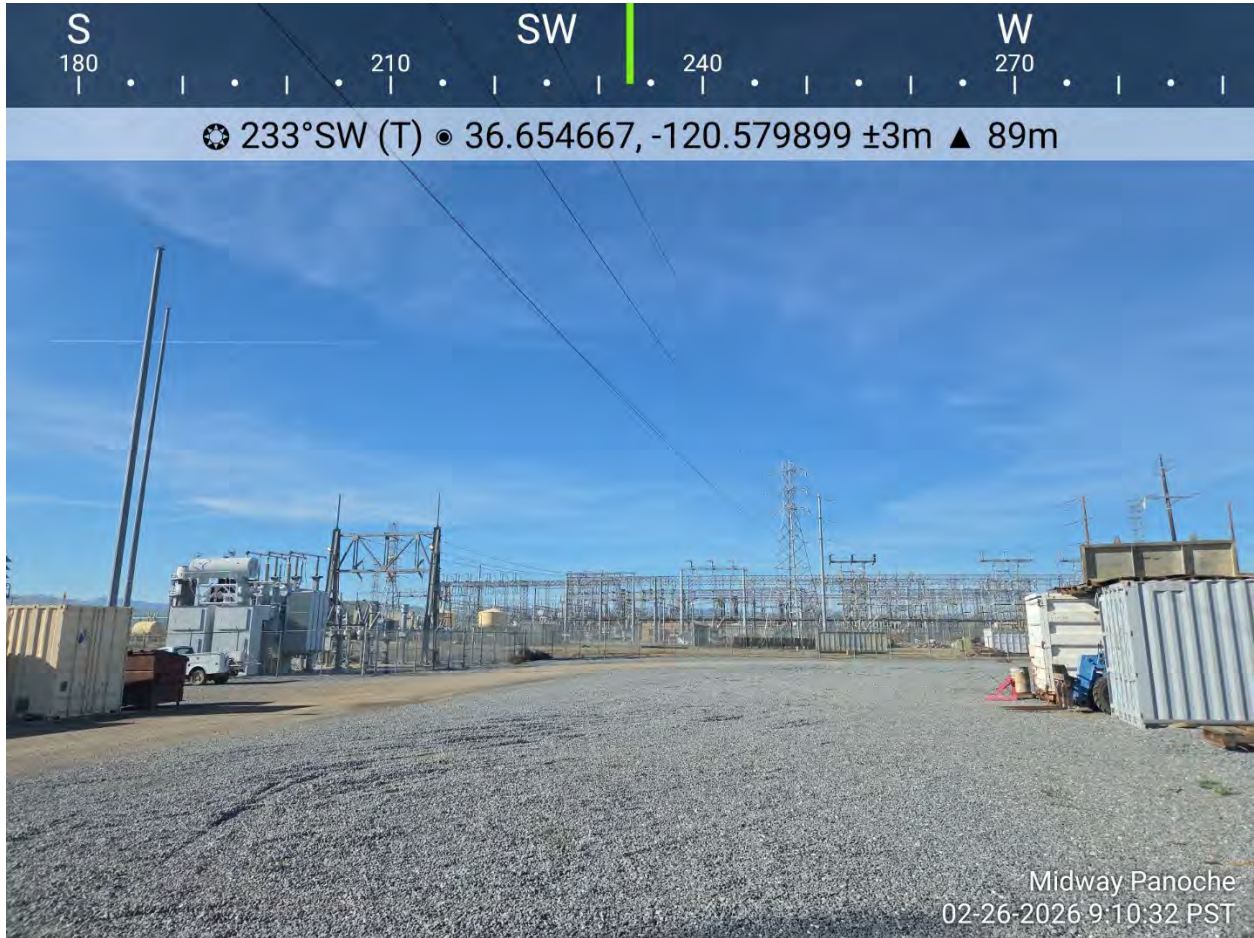
Overview of laydown area
