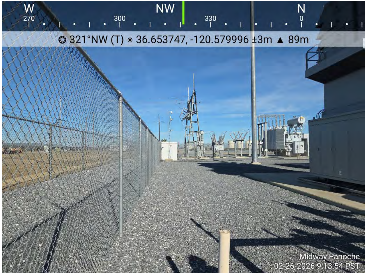
Overview of gen-tie excavation route
