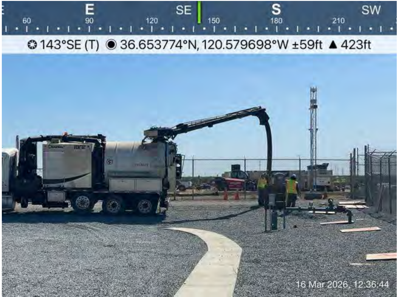
Hydrovac potholing activities
