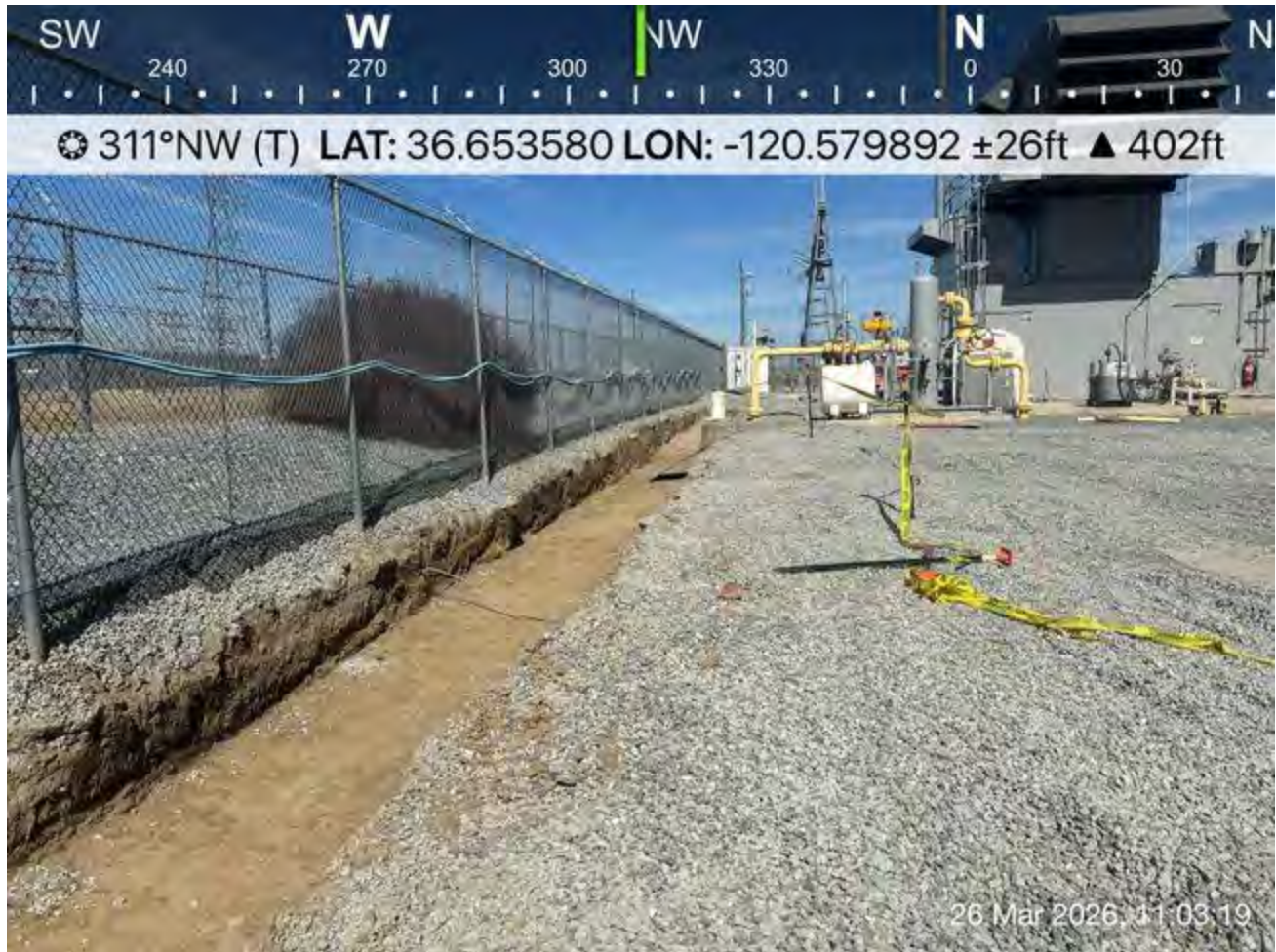
Additional wildlife ramp placed in trench.
