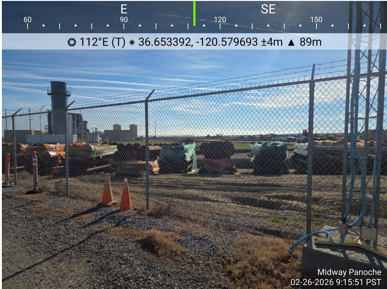
Partially uncovered pipe supports
