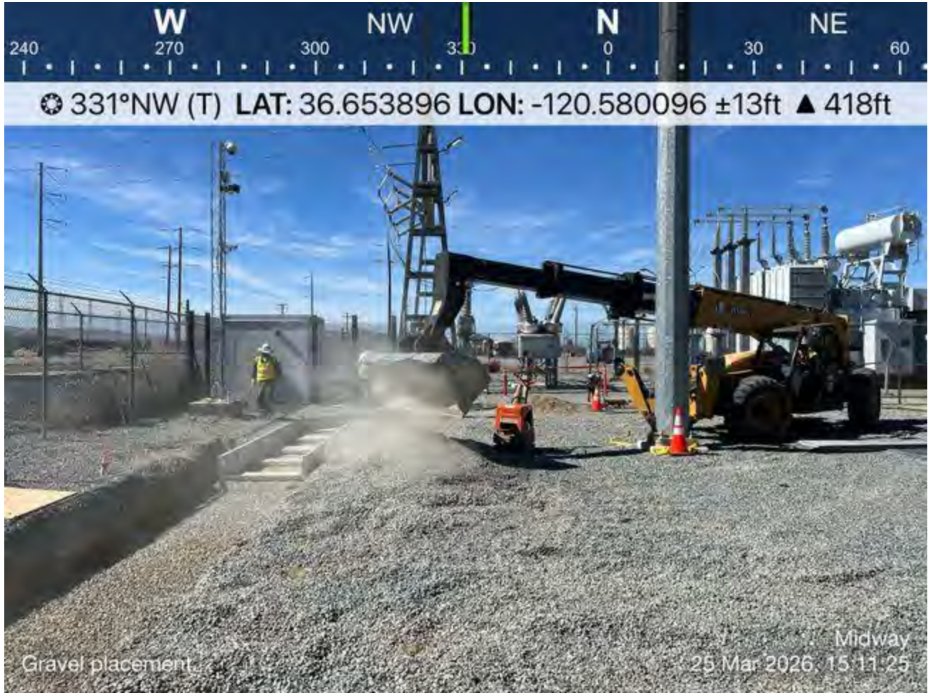
Gravel placement occurring near recently installed concrete runs.
