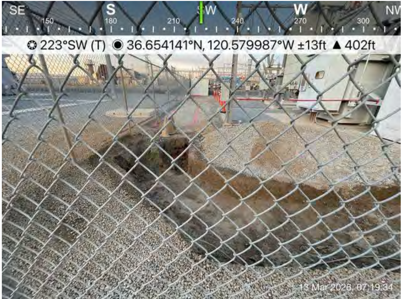
Morning sweep of open trench
