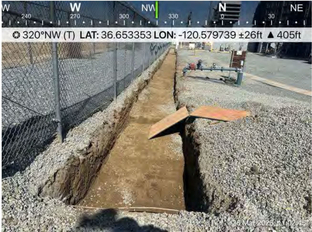
Wildlife escape ramp placed in trench.
