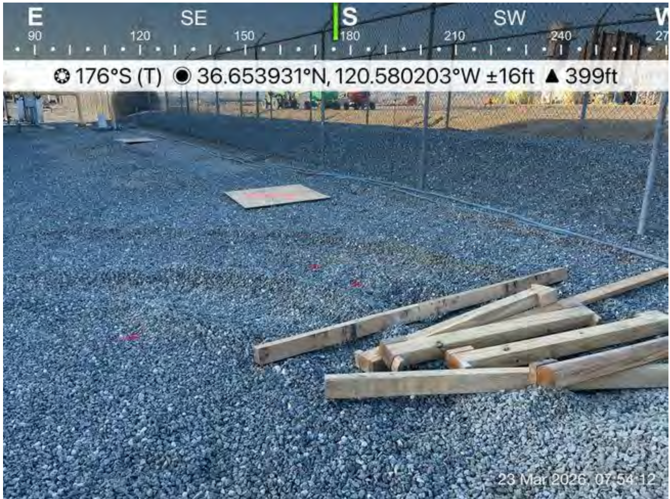
Morning sweep of the site that will be excavated
