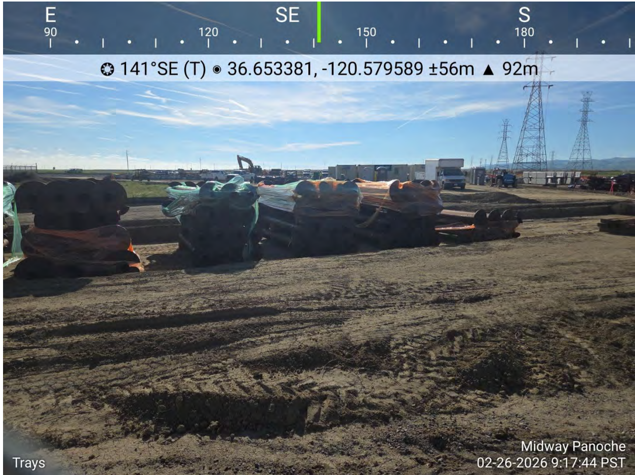
View of laydown area
