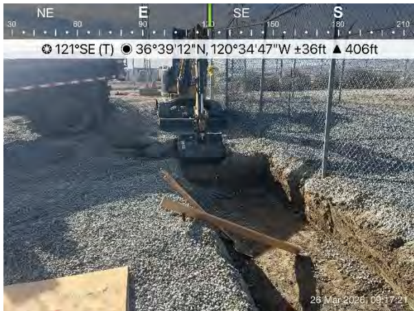
09:17 Facing southeast Teichert excavating the E end of trench.
