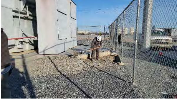
08:42 Facing north Site overview: Site preparation
