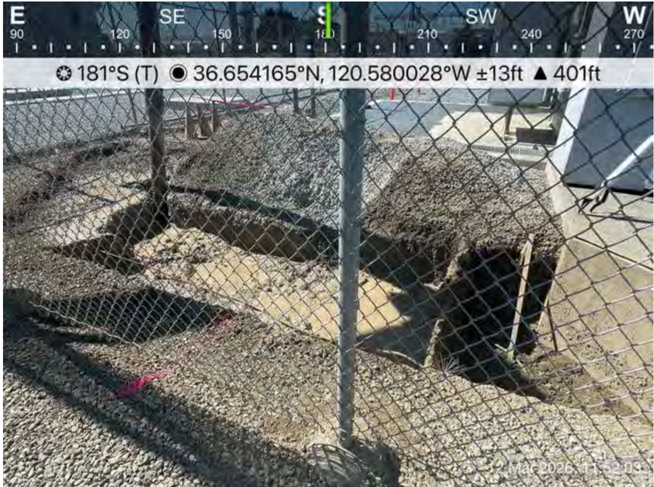
Continued hydrovac work
