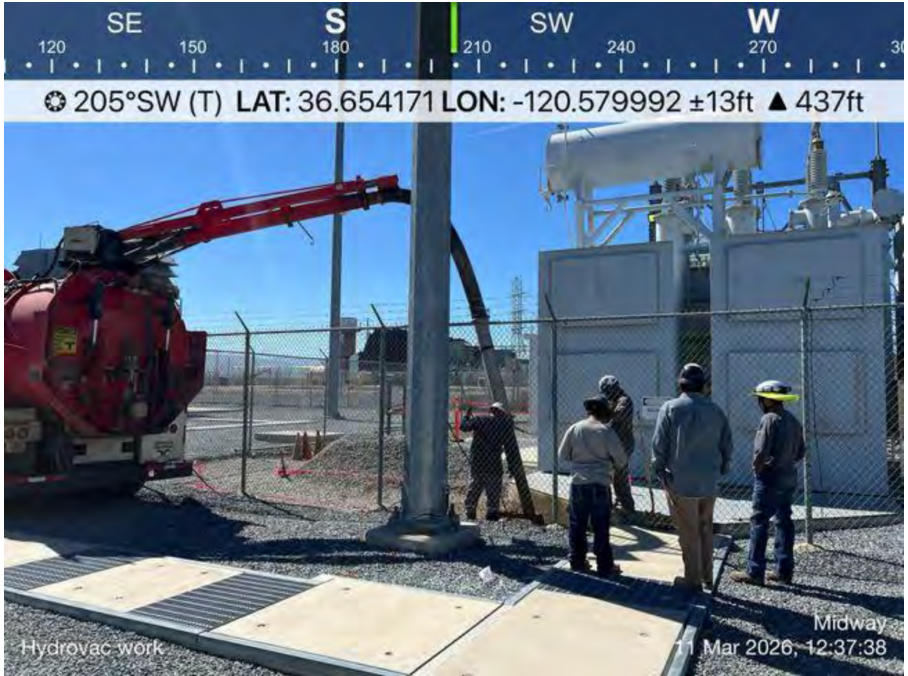
Hydrovac work activities continued.
