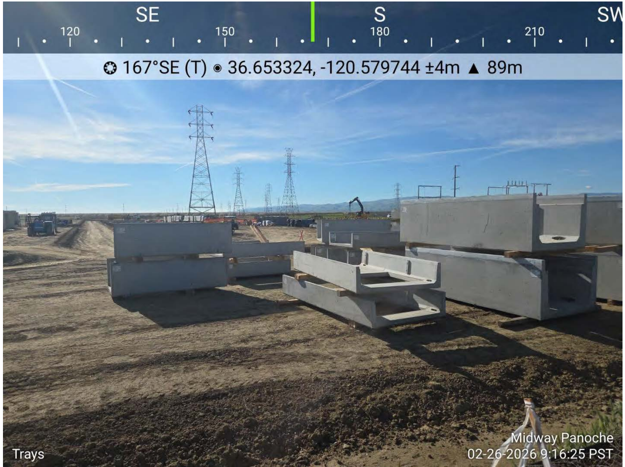
Trays to be installed in the excavation
