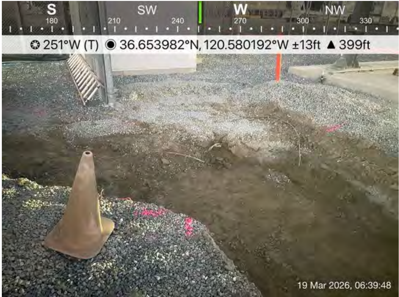
Morning trench check
