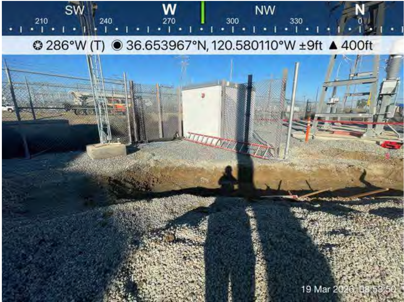
Excavation completed. Earthen ramp installed
