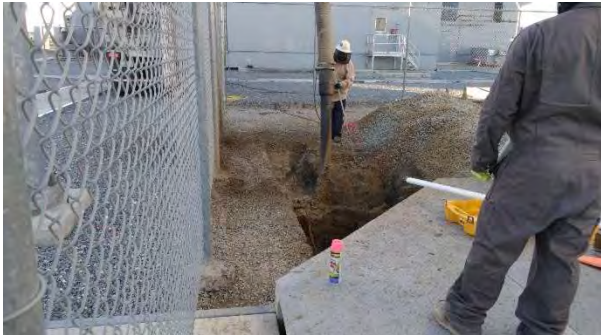
08:15 Facing south Potholing in peaker plant
