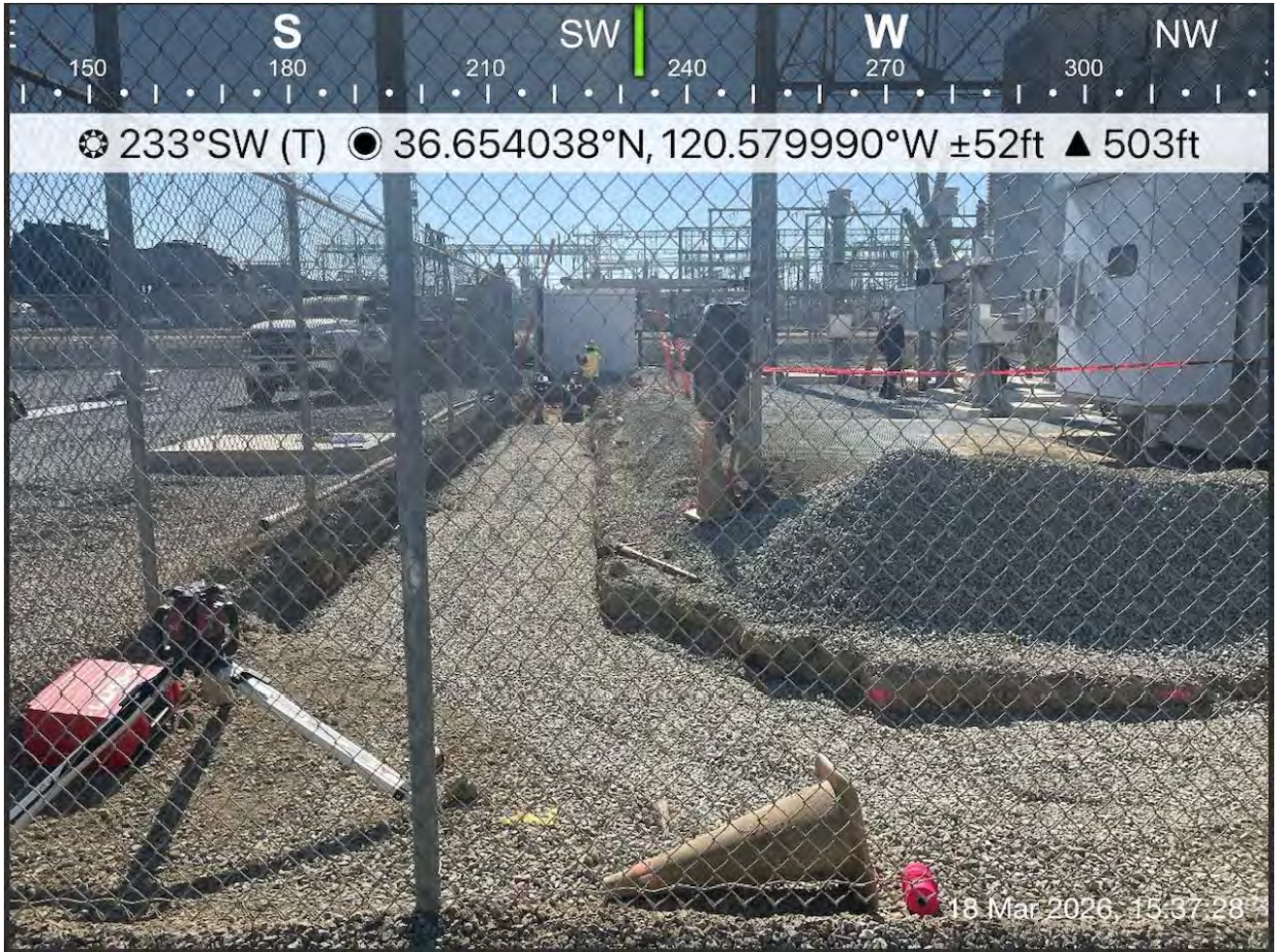
Gravel spread along the trench
