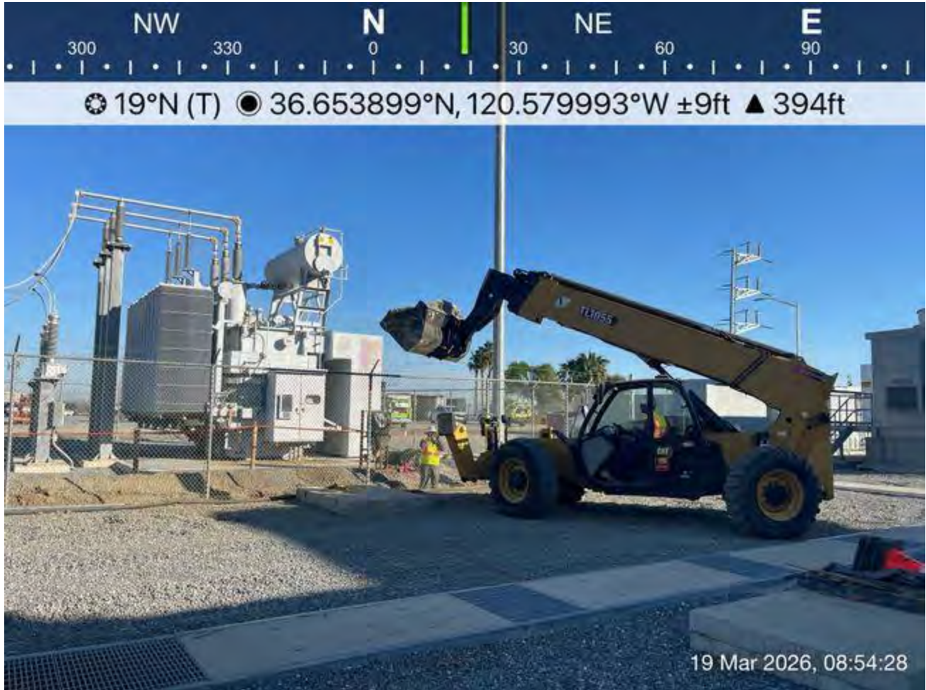
Gravel spread within trench
