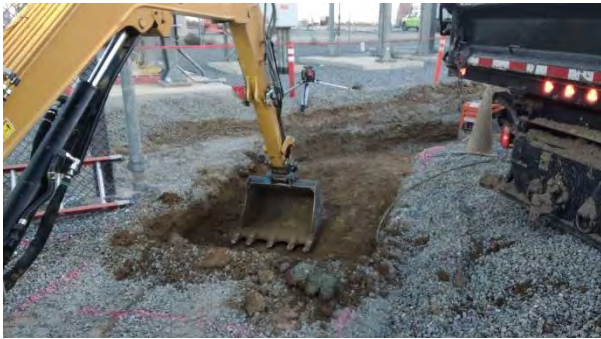
08:49 Facing southeast Trench overview
