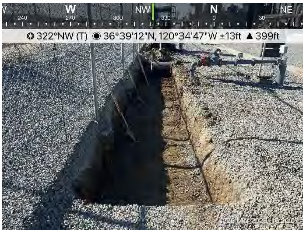
16:19 Facing northwest End of the day overview of excavated trench.
