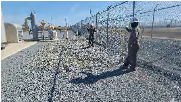
15:18 Facing west Gravel removal west side of site
