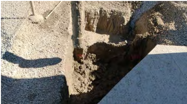
14:36 Facing southwest Trench overview
