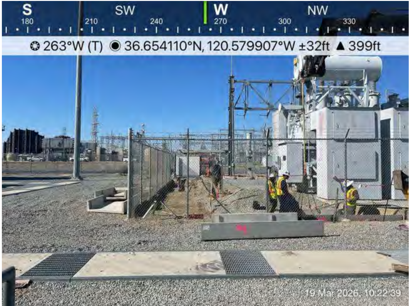
Progress within the trench
