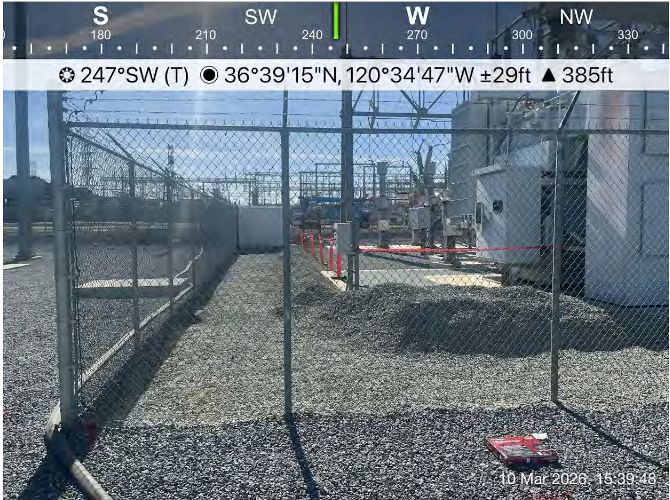
Photo 3: View of substation with rock removed.
