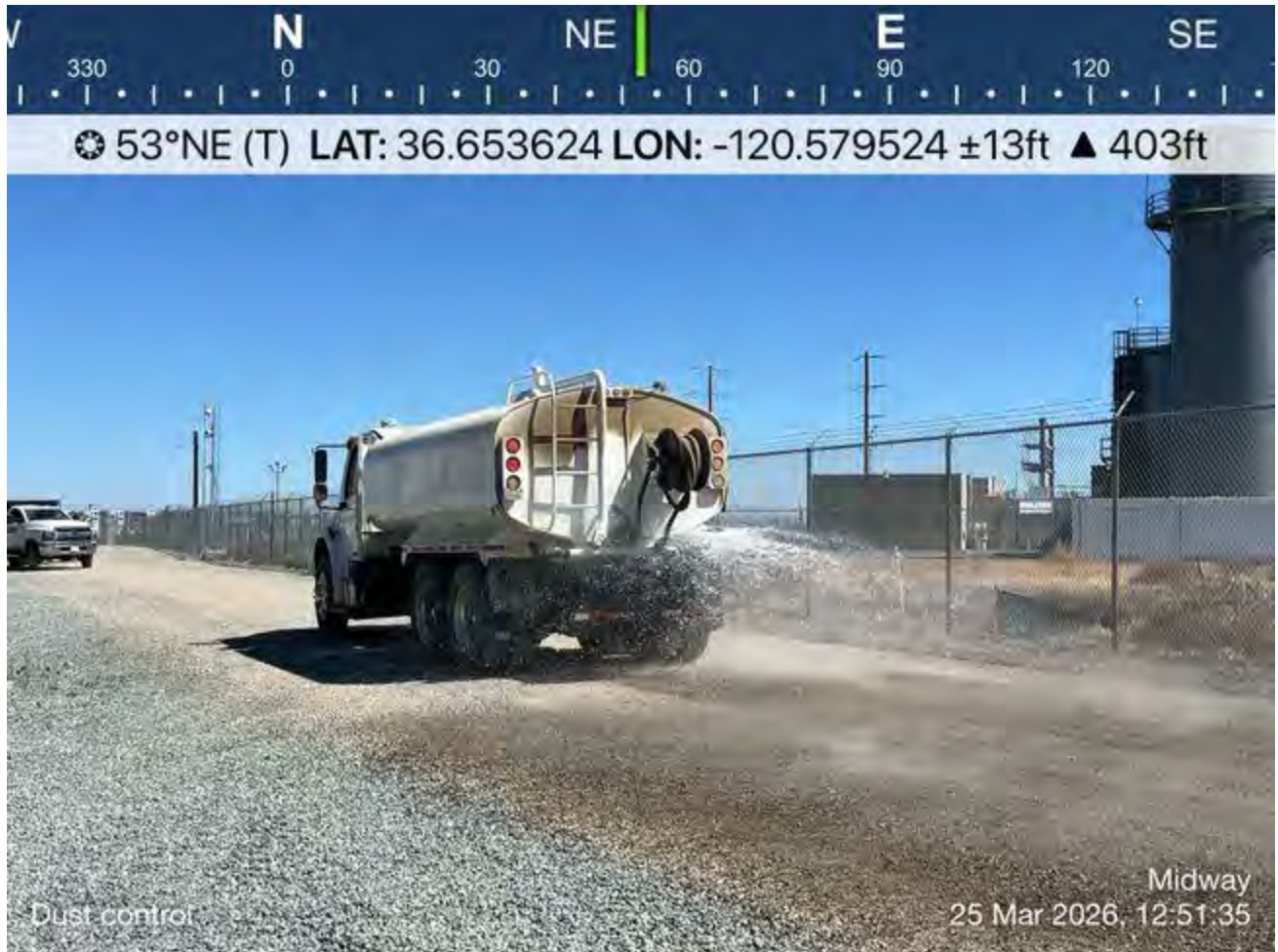
Water truck observed for dust control onsite.
