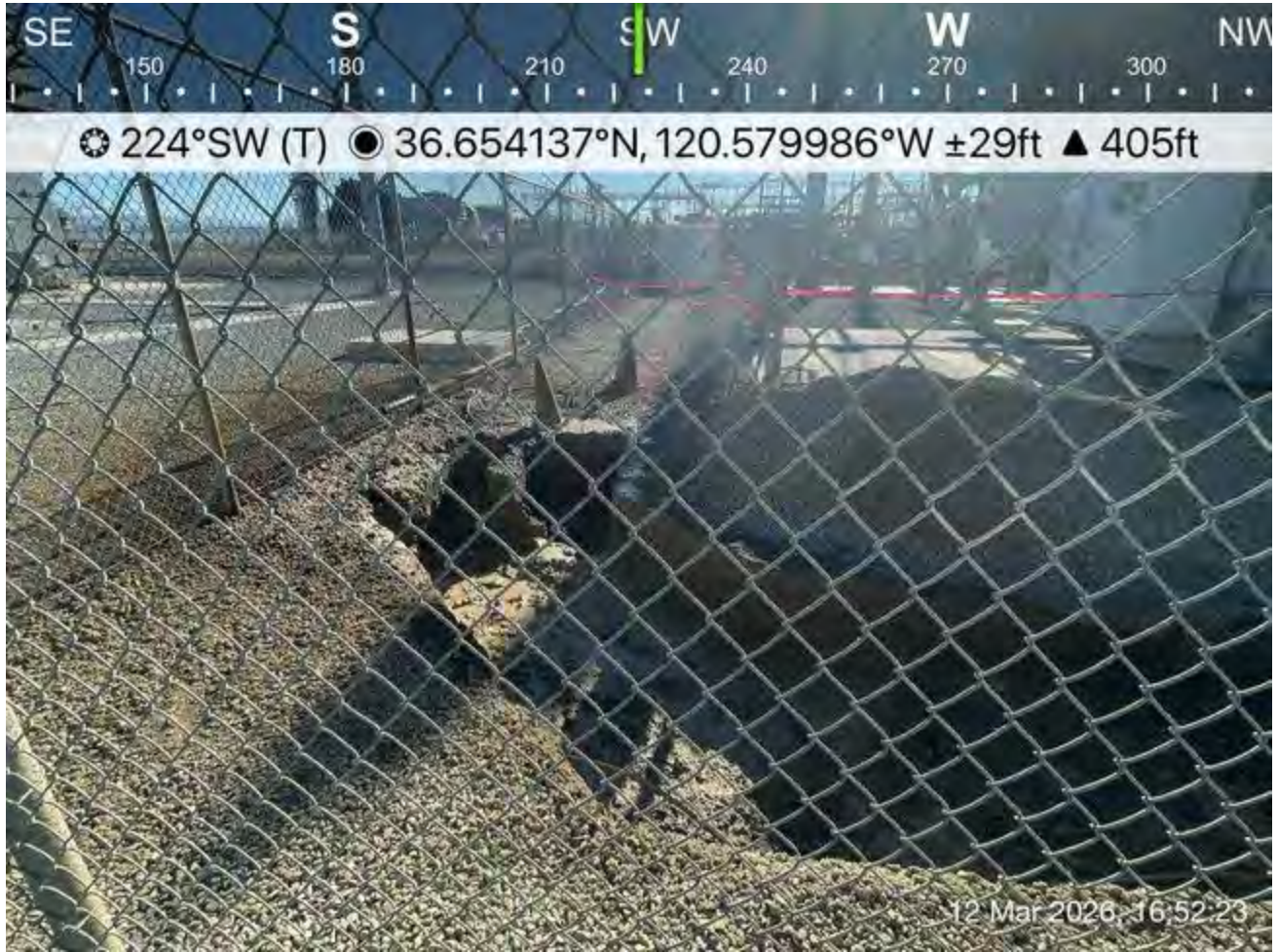
Excavation at end of day with adequate wildlife ramp
