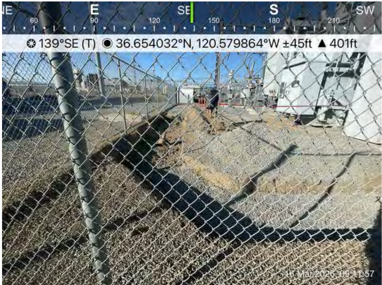
Sweep of open trench in the morning before work began
