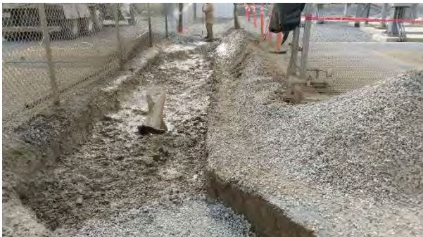
Facing southwest Trench overview
