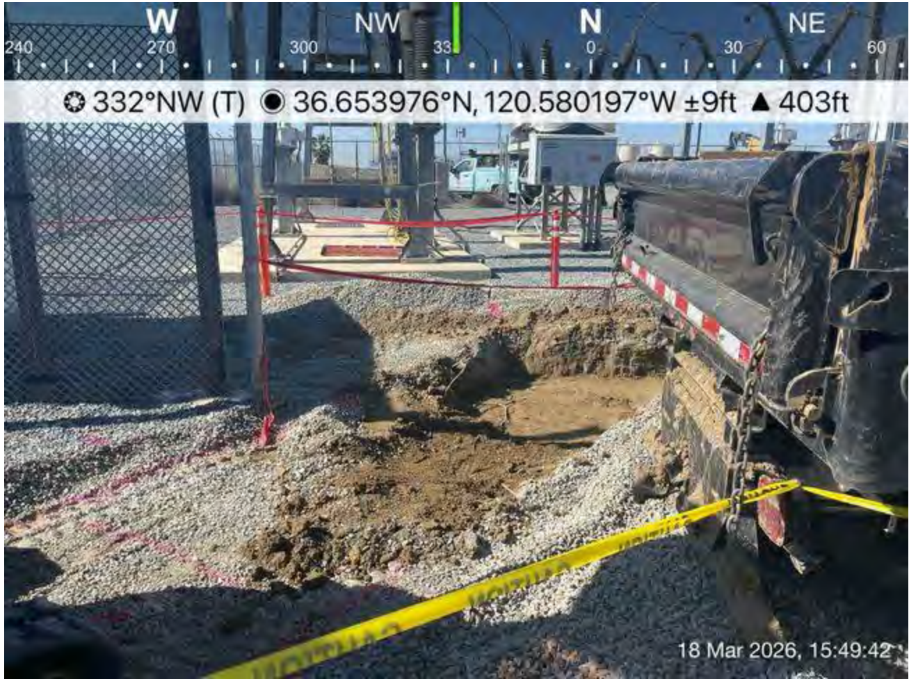
Trench ramped at end of day
