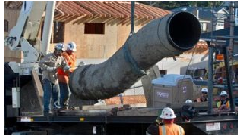
Decommissioned segment of pipeline removed by PG&E. Credit: The Mercury News
