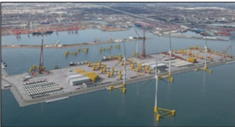
Staging and Integration (Rendering of Pier Wind) Source: Port of Long Beach
