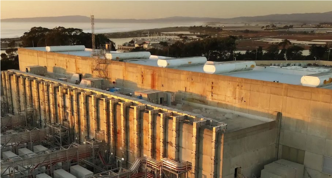
Source: Vistra (Moss Landing)
