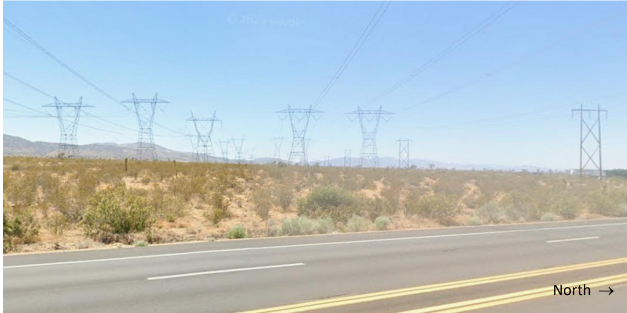
Figure 4. Existing Transmission Corridor that terminates at the Vincent Substation.
