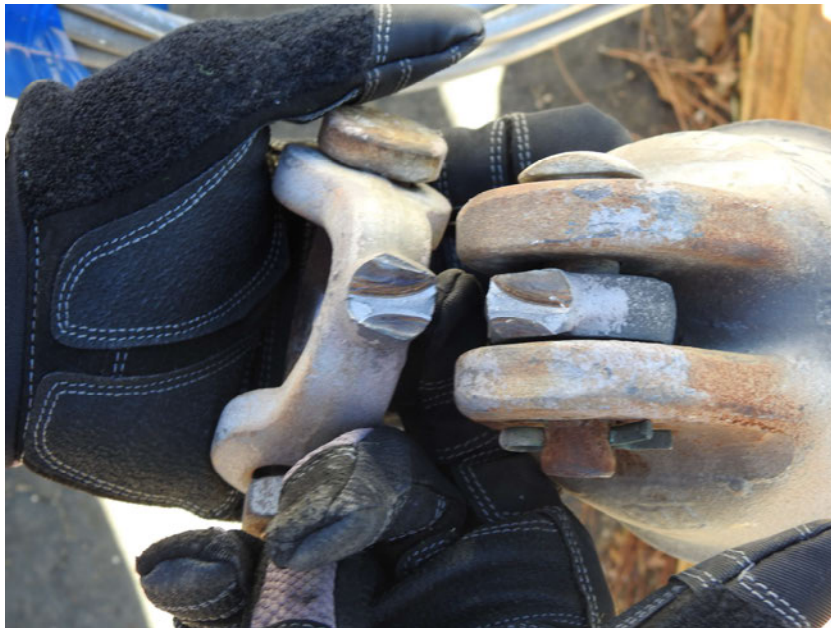
Figure 5: a photograph taken on October 25, 2019, at the evidence inspection at the SCE service yard, shows corrosion on the failed section of Y-clevis that supported the B-phase 220 kV conductor on tower M5-T2.
