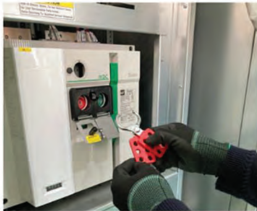
Figure 14: E-Panel LOTO location (DC Main Circuit)
