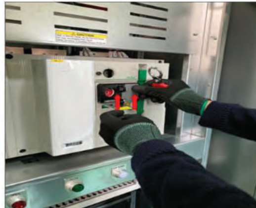
Figure 14: E-Panel LOTO location (DC Main Circuit)
