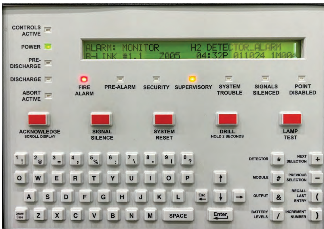
Figure 32: FACP Screen After Detection of H2 Sensor
