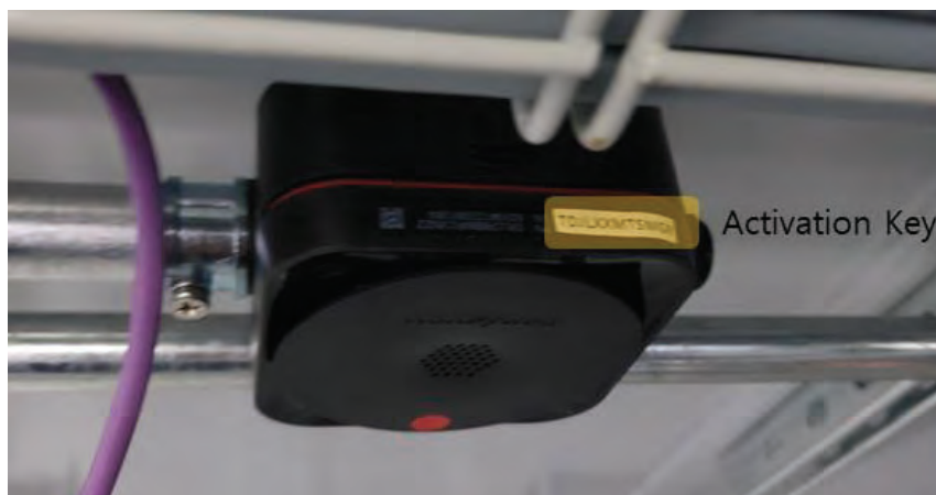
Figure 47: Activation key of the combustible gas sensor
