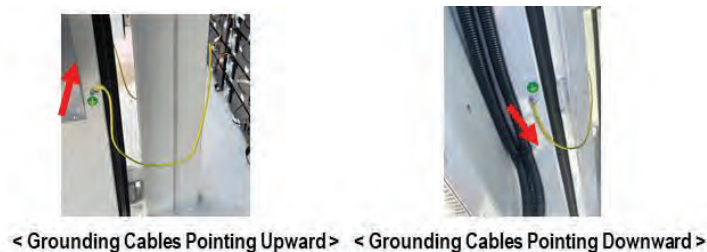
Figure 40: Grounding cable orientation
