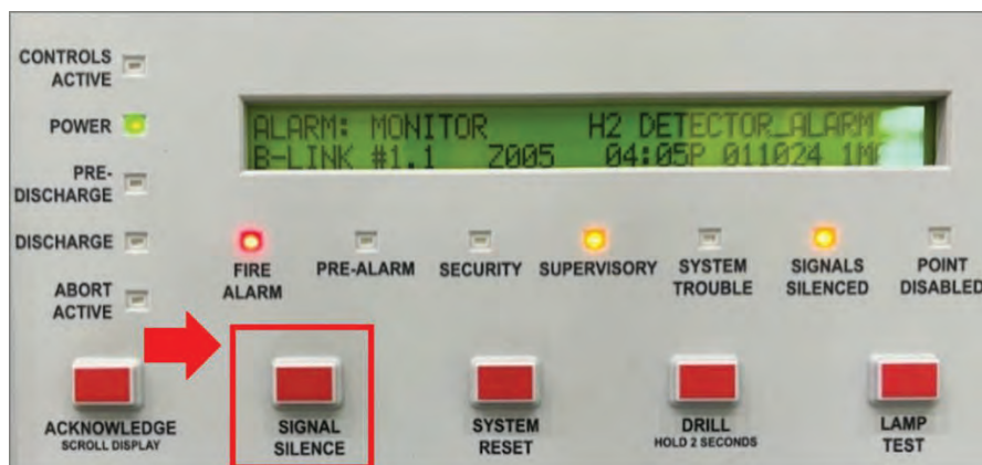
Figure 33: FACP screen after pressing SIGNAL SILENCE
