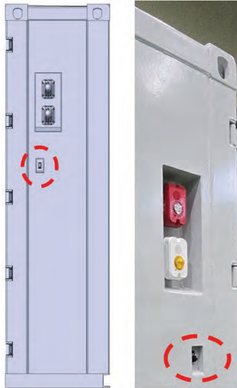
Figure 52: Location of LAN cable at the DC LINK
