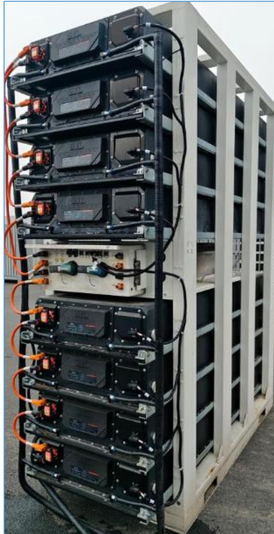
Figure 4.2 – View of single SYL SU5016U1250KC battery bay housing 8 modules.
