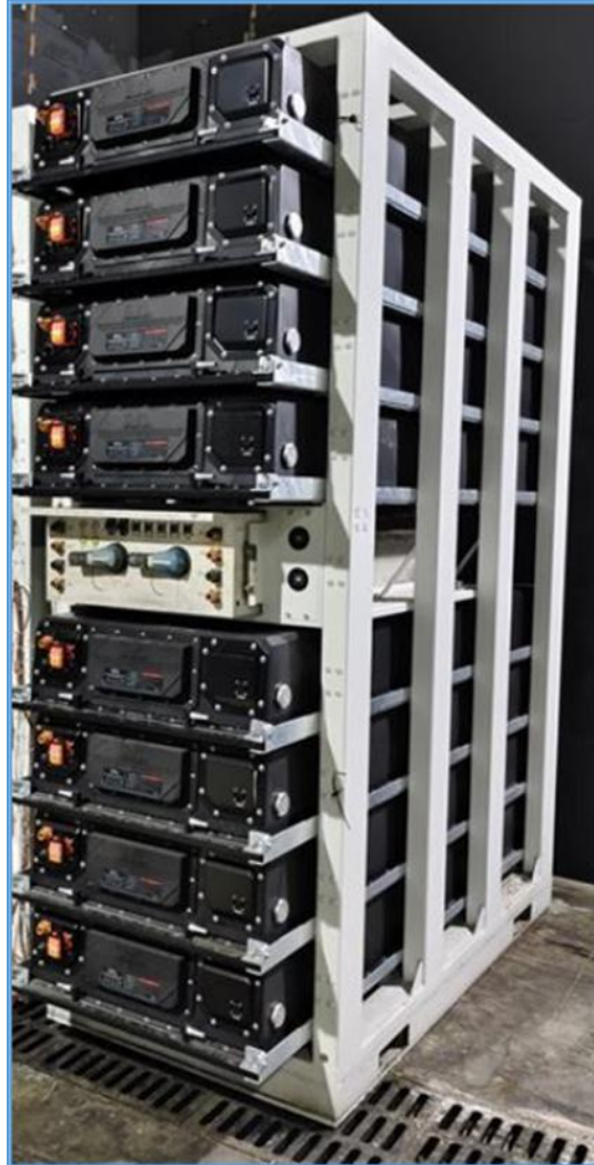
Figure 4.2 – View of single SYL SU3794U3794KC battery bay housing 8 modules.
