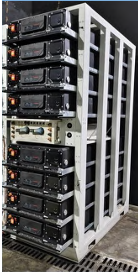
Figure 4.2 – View of single SYL SU3794U3794KC battery rack, containing 8 modules.
